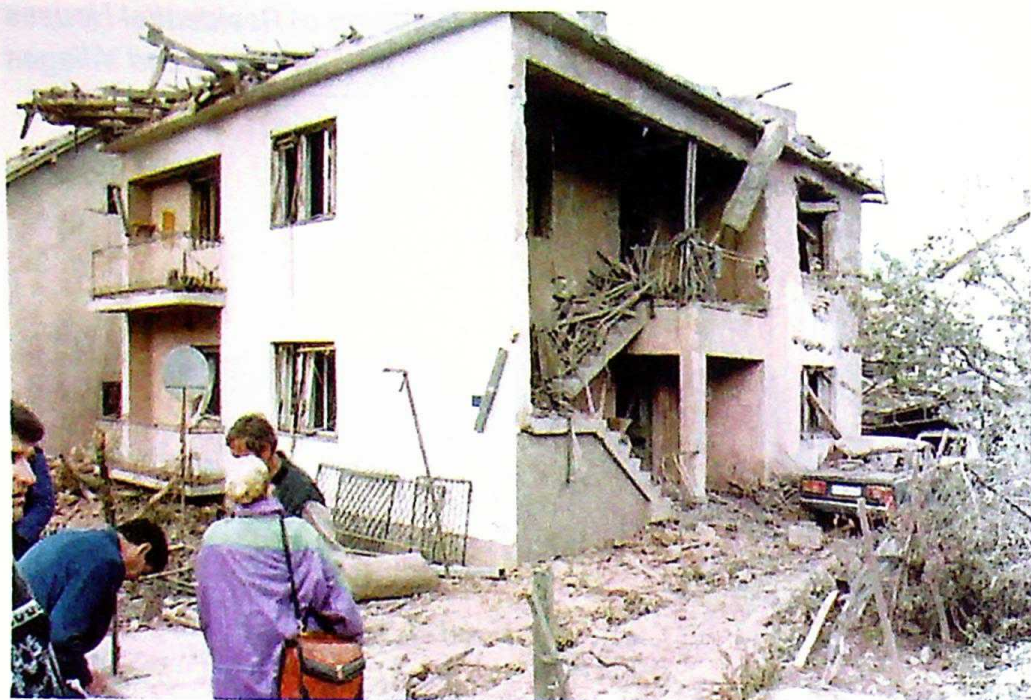
Photo 3 Close-up of demolished house of Dragan Stefanović, located in the immediate vicinity of the site of missile impact
