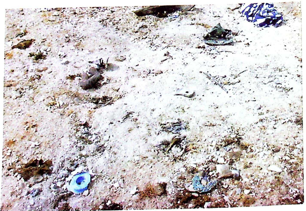
Photo 30 Broad view of damaged asphalt and scattered items
