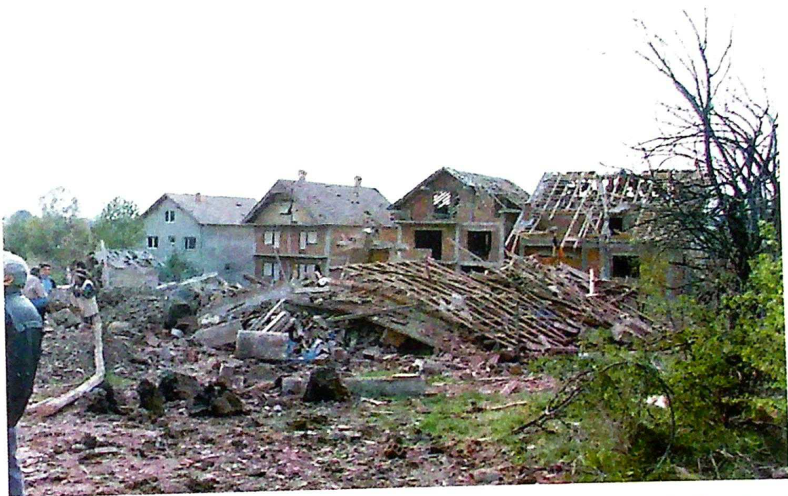
Photo 6 Broad view of the houses of Radica Ristić, No.20 Beogradska Street and Draganka Cvetković No. 18 Beogradska Street which were razed to the ground
