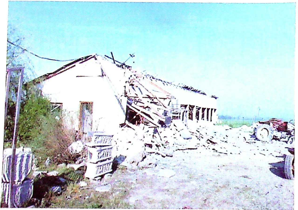
Photo 3 Demolished facility on the site where the refugee column was bombed
