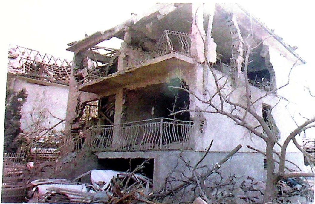
Photo 4 View of demolished house of Slobodan Milošević, No. 5 Zmaj Jovina Street, Surdulica
