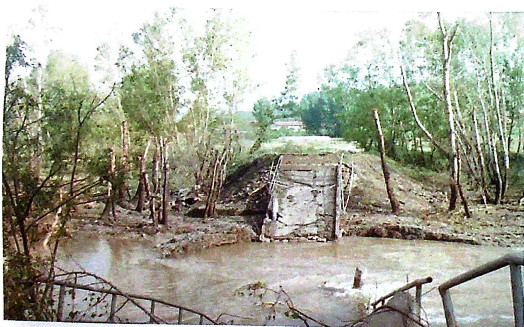
Photo 9 Demolished road bridge on the river Toplica in the village of Podina – Žitorada – Prokuplje, 29 April 1999 (Three attacks at 8:30 p.m., 10:30 p.m. and 11:00 p.m.)
