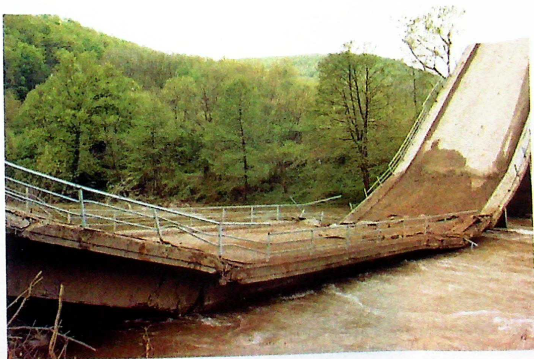
Photo 8 Close-up of the demolished "Sarajevo" bridge
