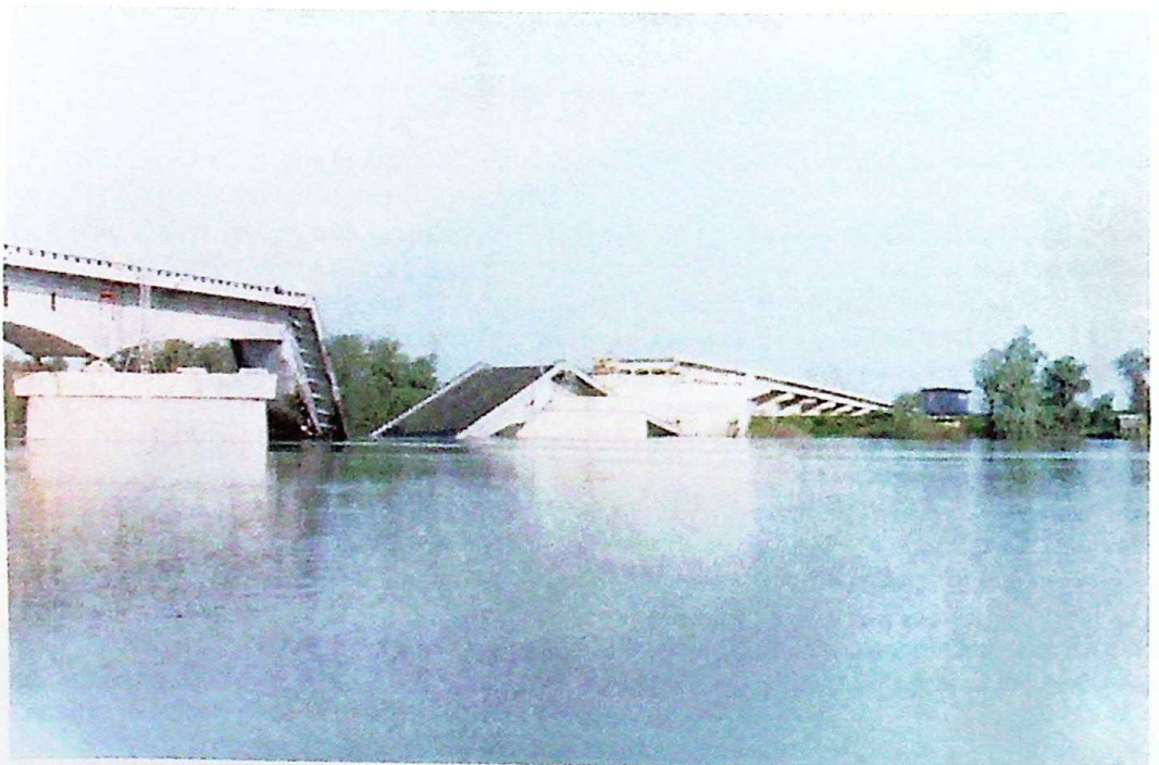
Photo 4 Broad view of the right side side of the demolished "Ostružnica" bridge
