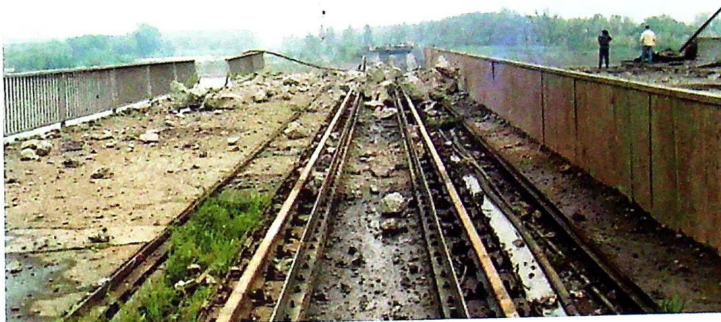
Photo 1 Demolished Žeželj Bridge on the Danube – Novi Sad, 26 April 1999 (Second attack)
