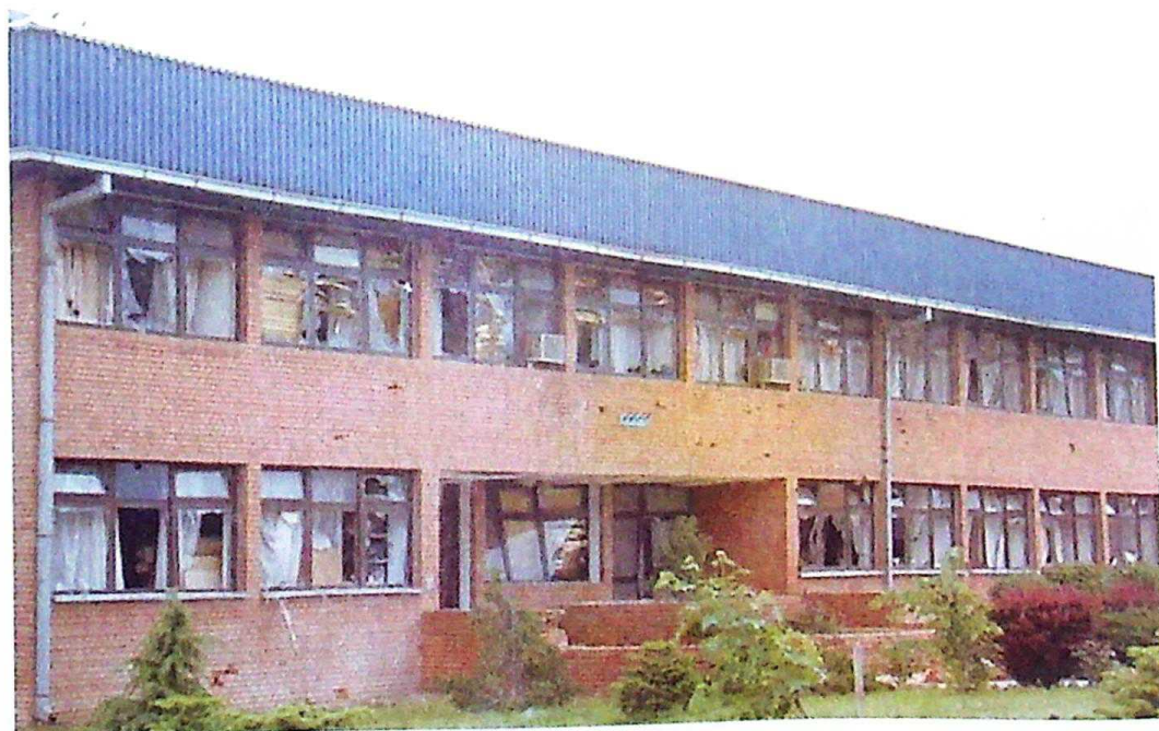
Photo 5 Bombed Administration Building of the KPD "Dubrava"
