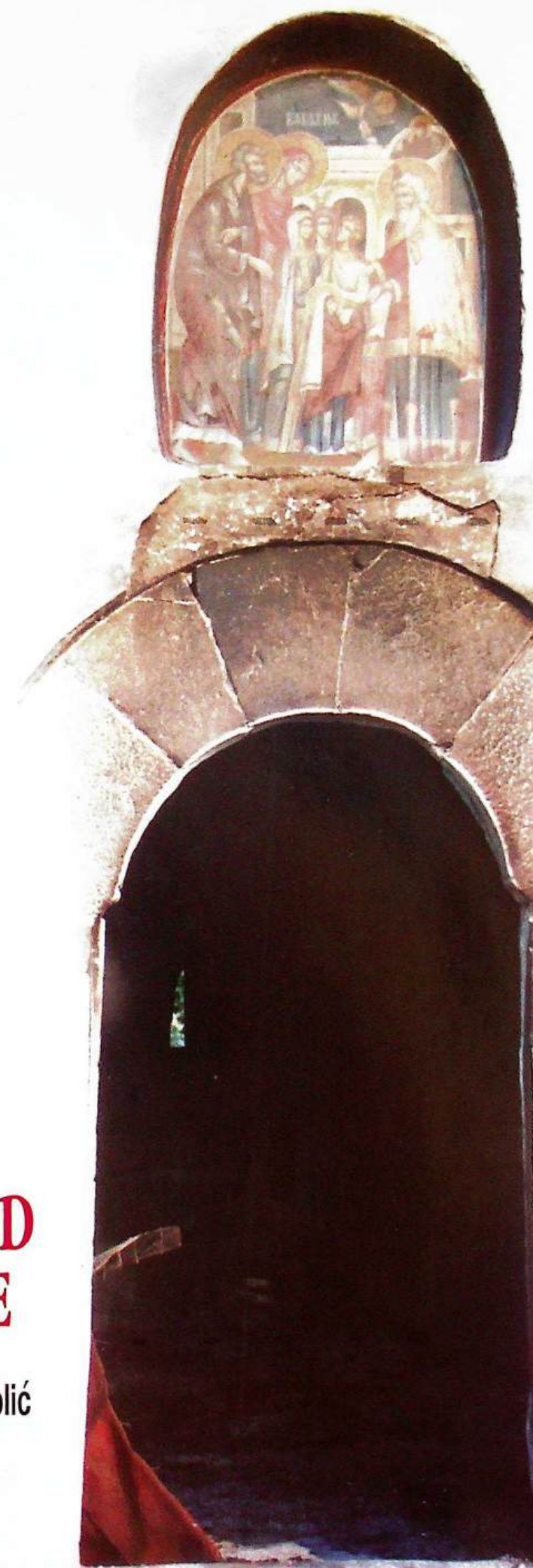
Dolac church (14 c). Main entrance. Mined and destroyed to the ground.
