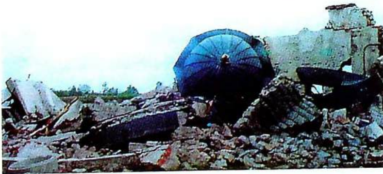
The Church after the Second Explosion.
