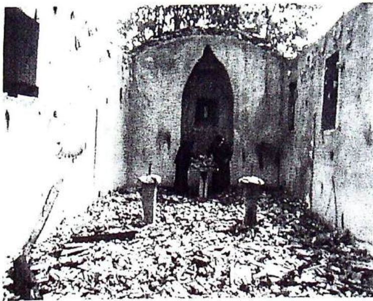
The Church in Zegra, after Demolishing and Burning.
