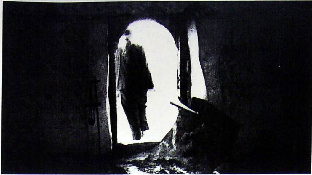
Demolished interior of the church in Dolac
