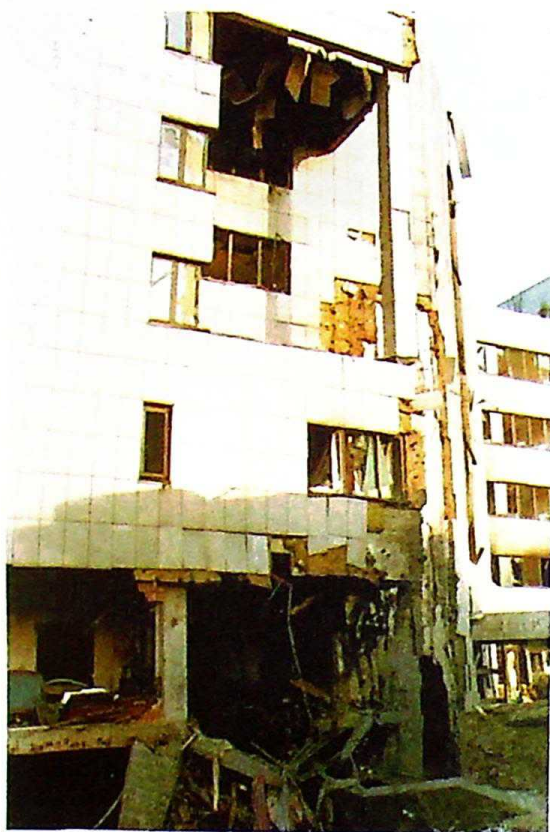
Photo 62 Demolished part of the western wing of the main building
