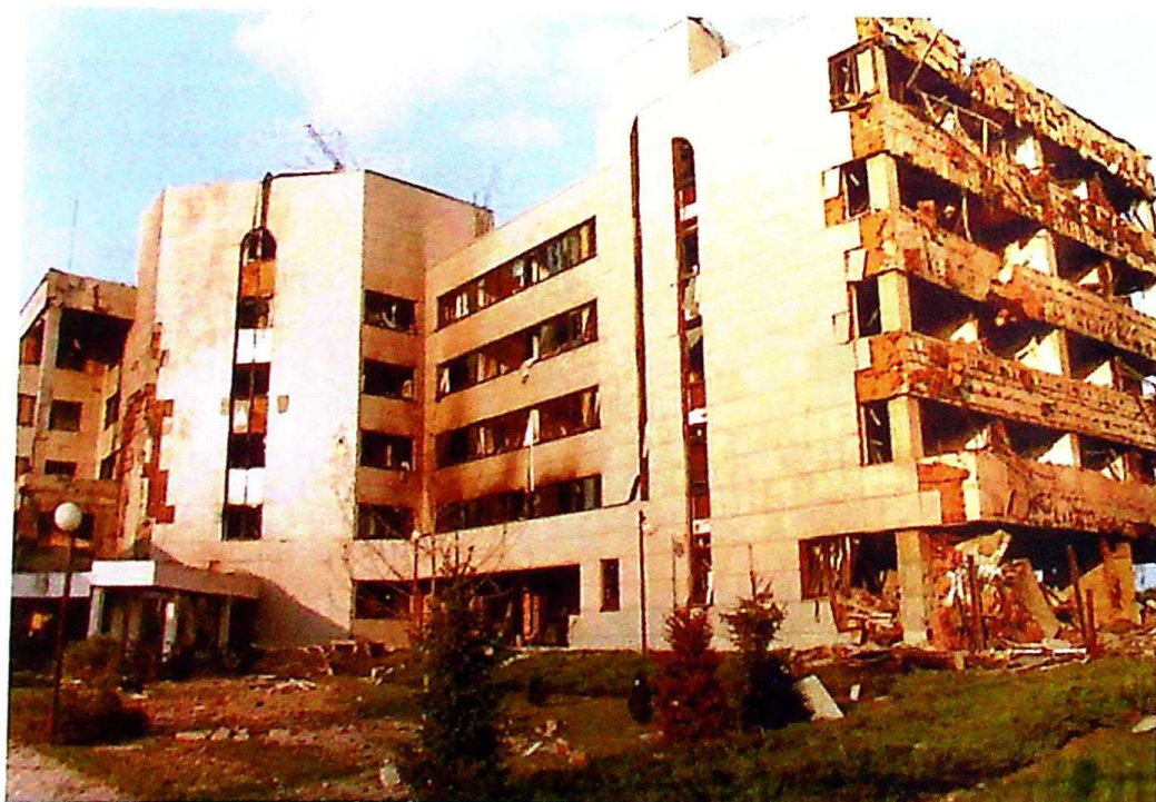
Photo 55 Embassy building – south-western side
