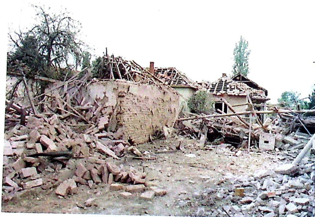
Photo 45 Demolished house of Zoran Avramović in the village of Medoševac, 29. novembra Street No. 9 – one of some 50 houses demolished or damaged in Medoševac on 7 May 1999
