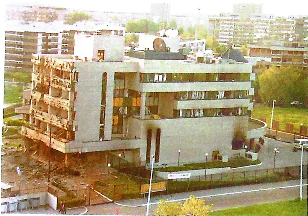
Photo 54 Close-up of the south-eastern side of the demolished building
