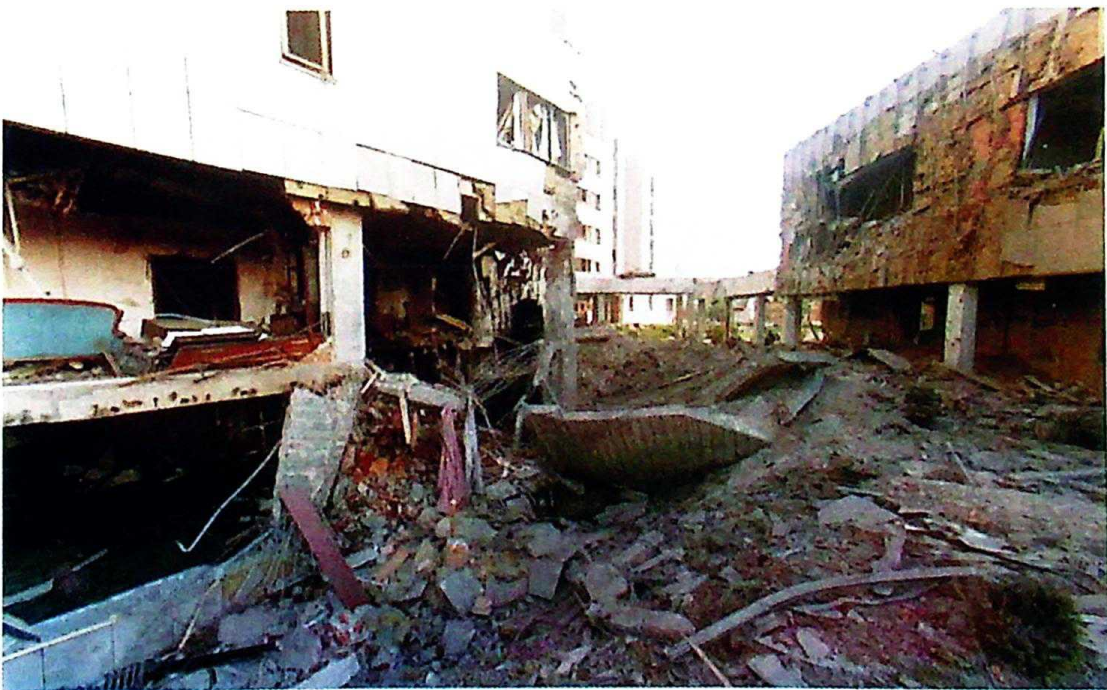
Photo 61 Close-up of the point of impact between the main building and an outbuilding
