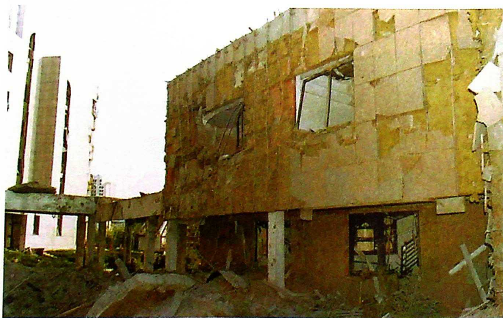
Photo 63 Destroyed part of the eastern wing of an outbuilding
