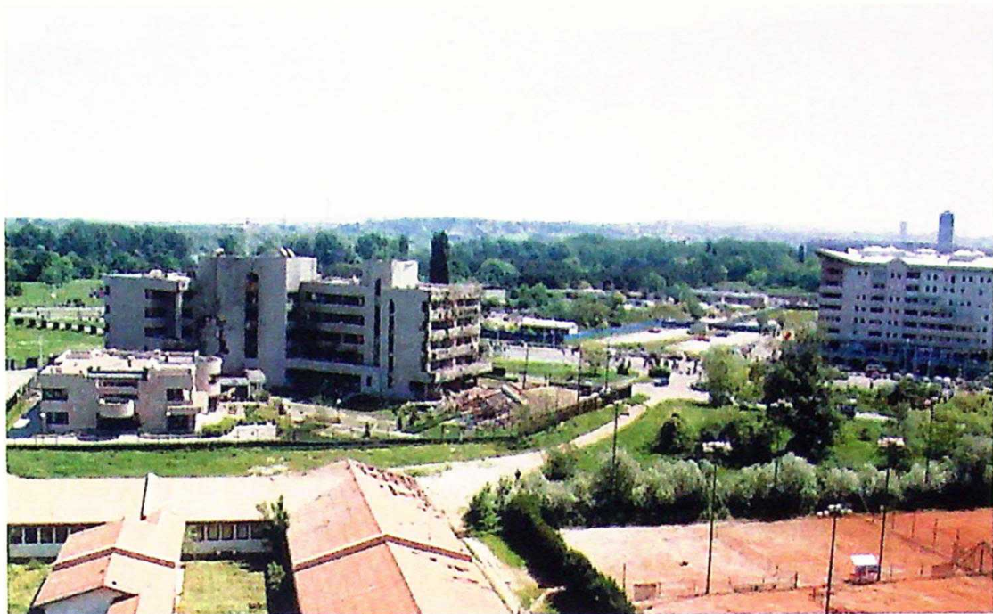
Photo 52 Broad view of the Embassy of the PR of China (main building and an outbuilding)
