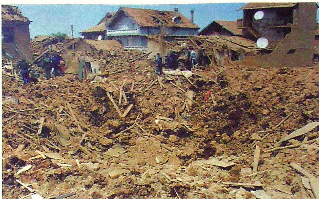
Photo 23 Totally demolished 4 houses of the Beriša family. Four members of the Beriša family were killed and 7 seriously injured
