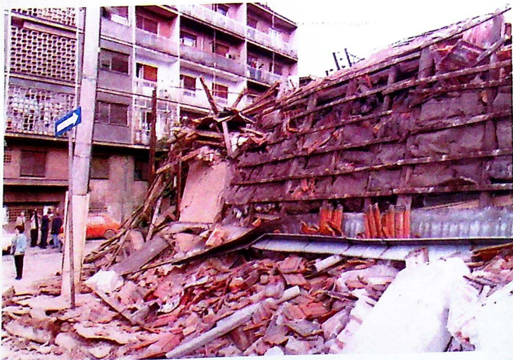
Photo 35 View of the demolished facilities from the opposite side
