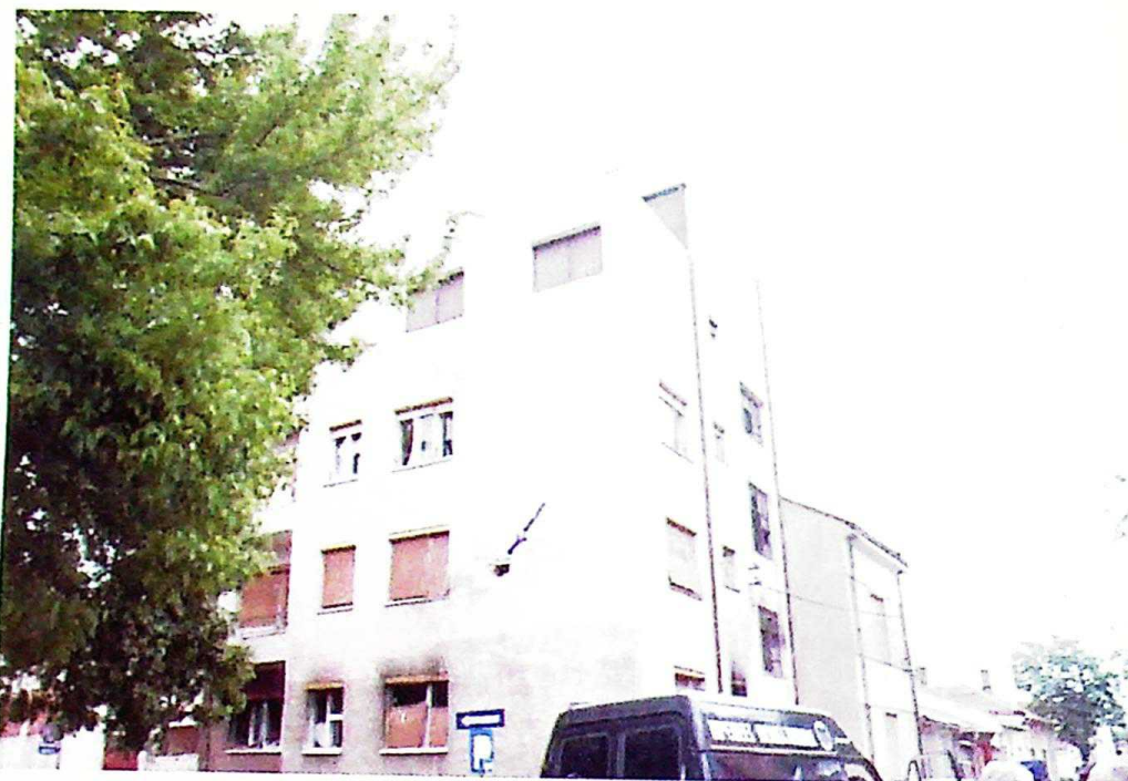
Photo 48 The building in Šumatovačka Street No. 9 with visible crater made by a cluster bomb
