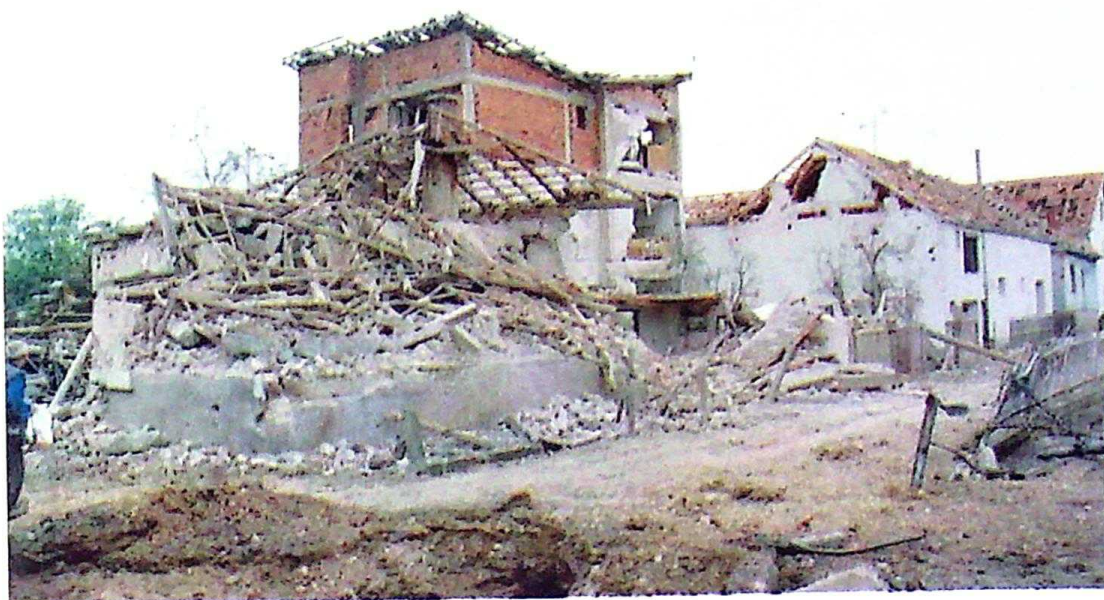
Photo 46 Demolished house of Sava Krstić in Medoševac, 29. novembra No. 8
