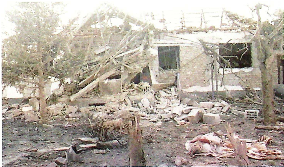
Photo 75 Demolished house on Kulinovačko Polje III Street No. 5 in Čačak, property of Velija Džemailović, in which the owner and Dragan Obrenić were killed on 10 May 1999
