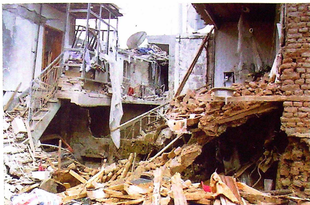
Photo 15 Demolished houses at Nos. 31 and 33 Podrimska Street, owned by Masar Gaši and Ramadan Gaši – Prizren, 28 April 1999
