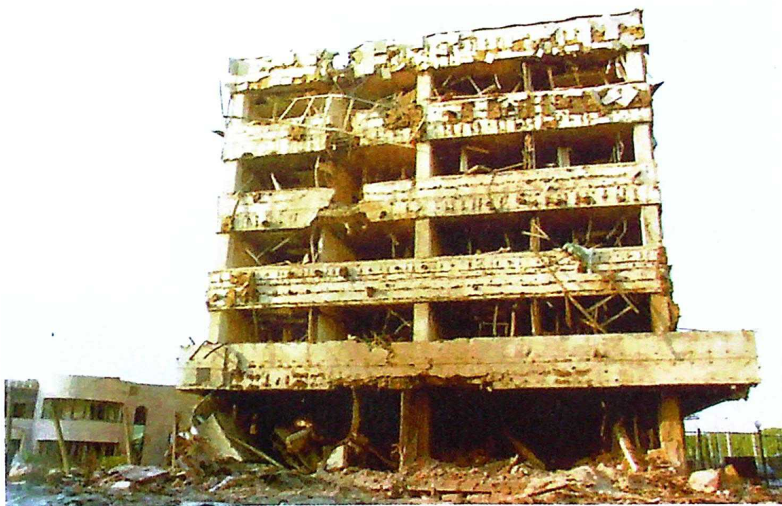
Photo 57 Close-up of the demolished southern facade of the Embassy building
