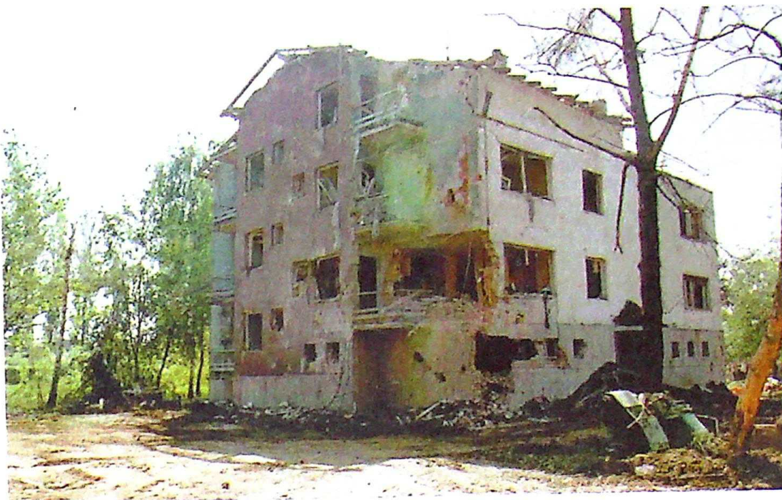
Photo 41 The demolished apartment building consisting of 12 apartments at No. 18 Milorad Pavlović suburb – Valjevo, 2 May 1999
