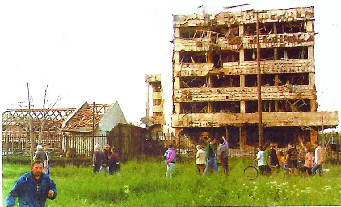
Photo 56 Demolished southern facade and an outbuilding
