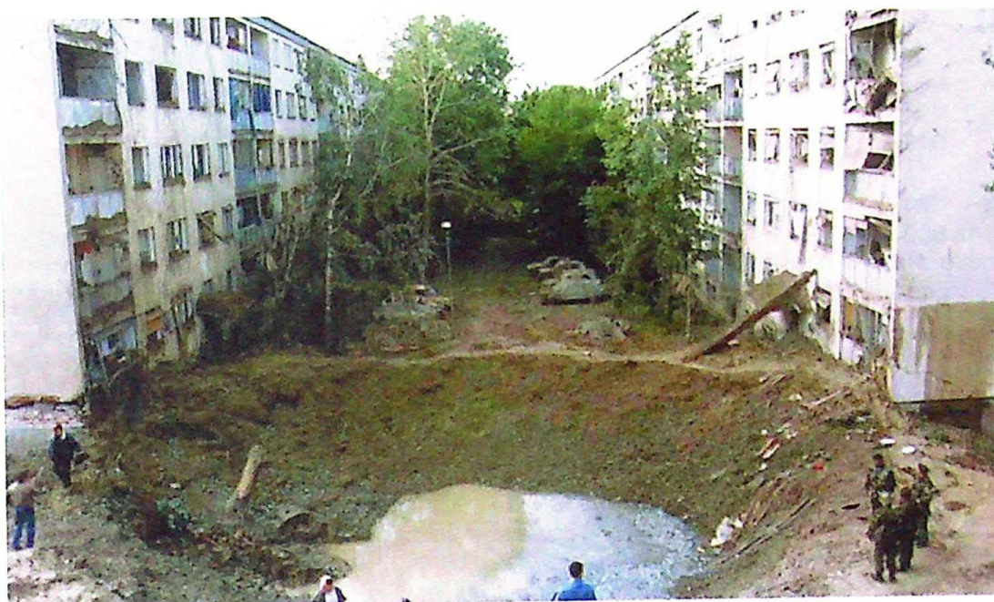
Photo 43 Crater made by a NATO bomb located between apartment buildings in Đule Molnara Street, Detelinara Estate in Novi Sad, 6 May 1999 (about 100 apartments damaged)
