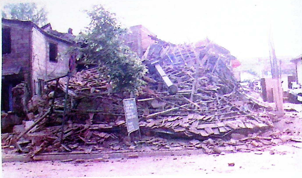
Photo 34 Demolished family house, 57 Maksima Gorkog Street, Belgrade, hit by a missile. The restaurant "Zlatni ovan" and a number of surrounding flats were destroyed, 30 April 1999
