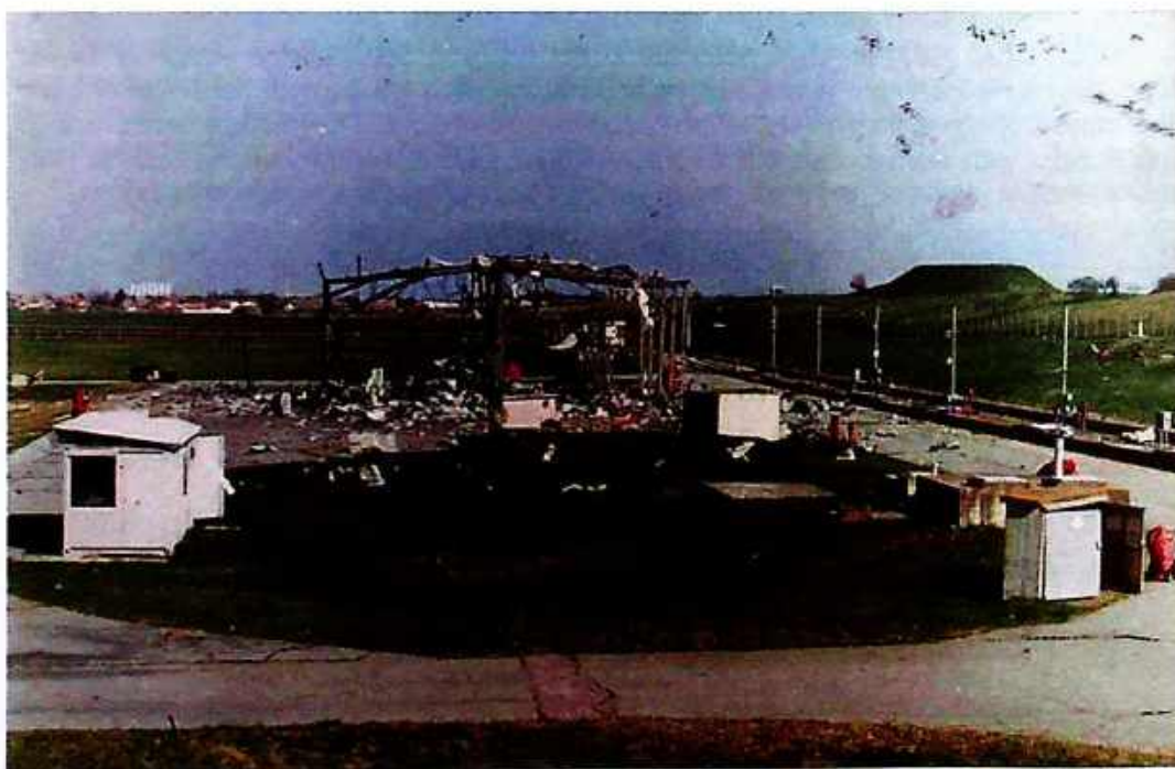
Photo 6 Damaged installations of "Naftagas" on the Čonoplja-Kljajićevo road, municipality of Sombor, first attack 4/5 April 1999
