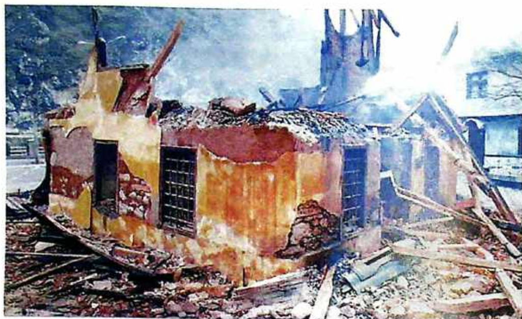
Photo 6 Close-up of the demolished Prizren League building
