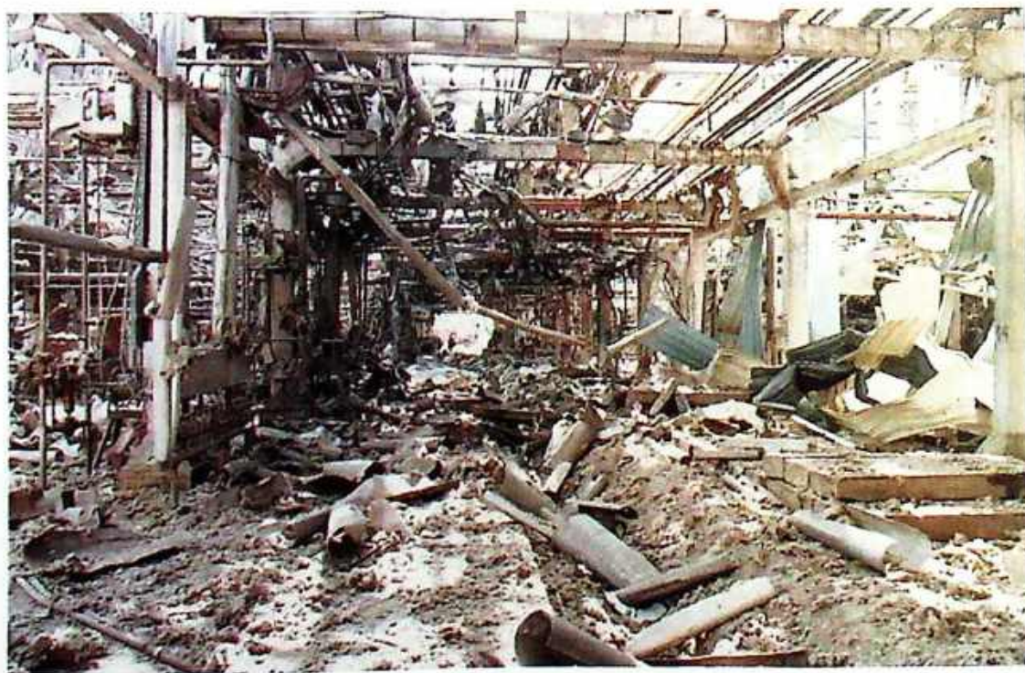
Photo 19 Close-up of demolished secondary plant installation
