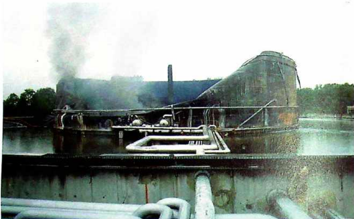
Photo 29 Destroyed crude oil storage tank
