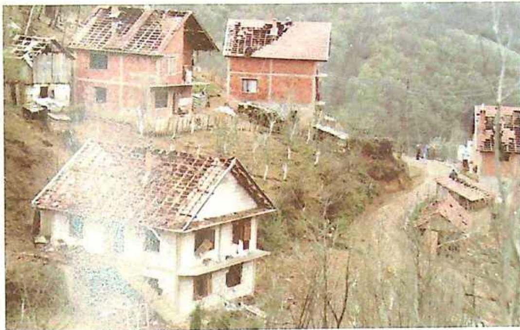
Photo 74 A few of the score of houses damaged on April 20, 1999 in the village of Dolovi, Novi Pazar
