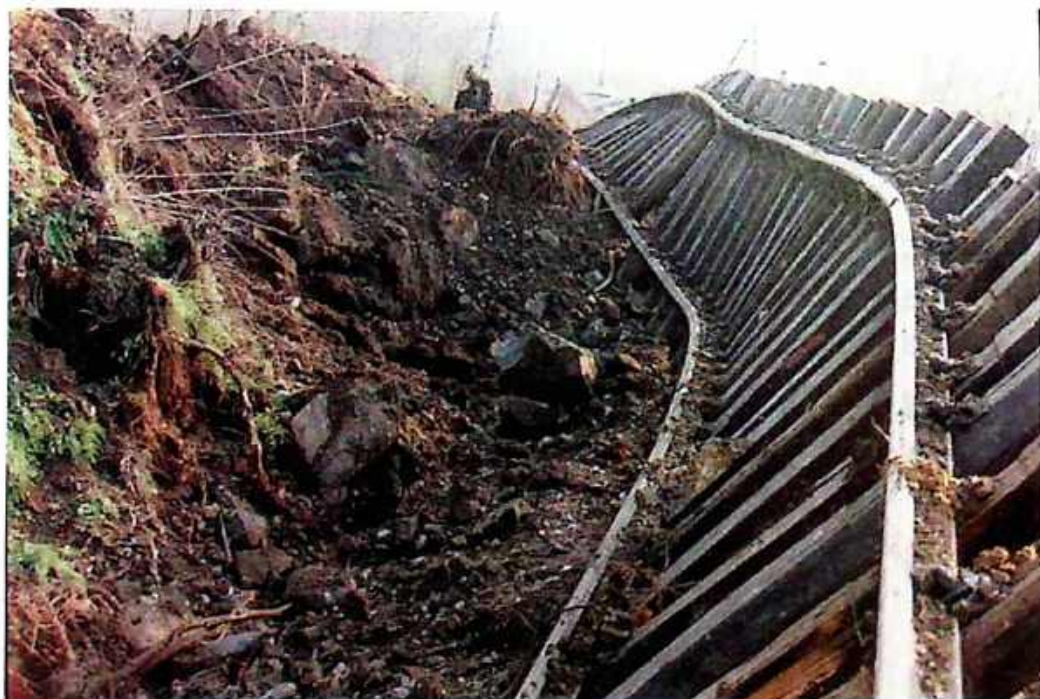
Photo 27 View of the demolished railway
