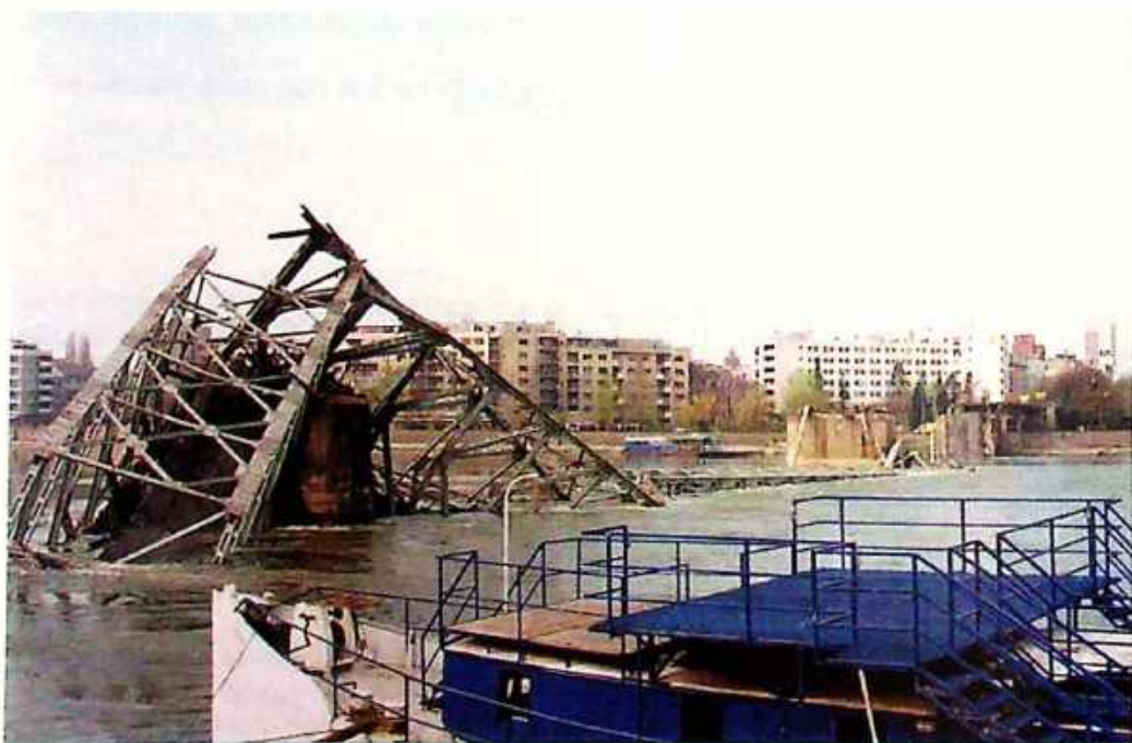
Photo 2 A part of demolished Varadin Bridge structure in Novi Sad
