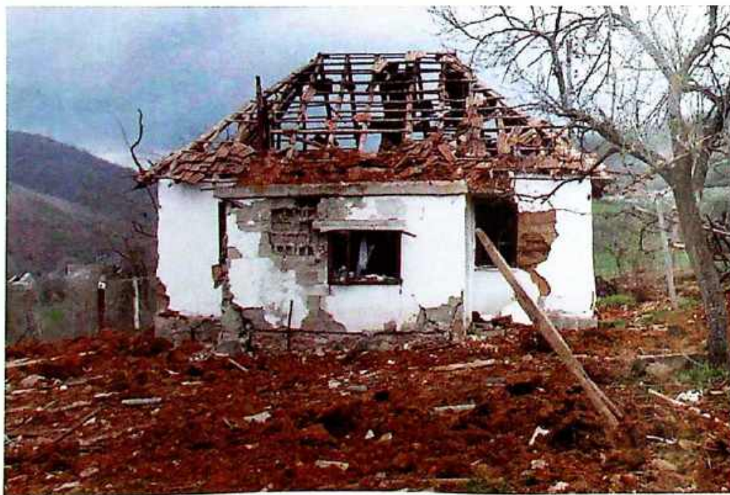
Photo 46 Close-up of one of the demolished houses
