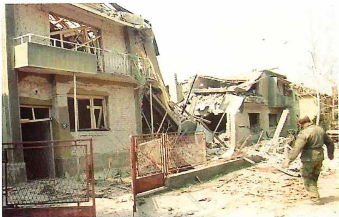
Photo 24 Demolished houses on Vuk Karadžić St. in Aleksinac
