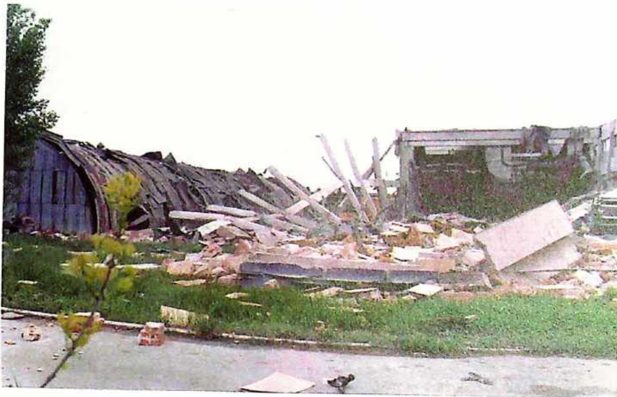
Photo 48 Destroyed PVC and EPS production plant
