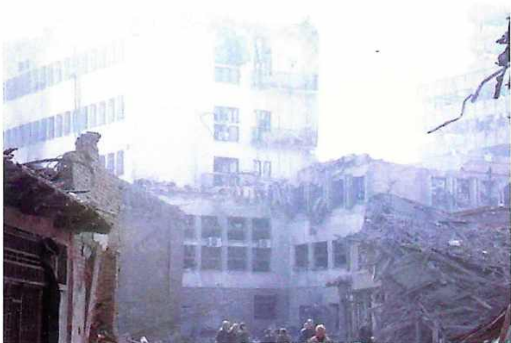
Photo 29 View of the damaged post office building
