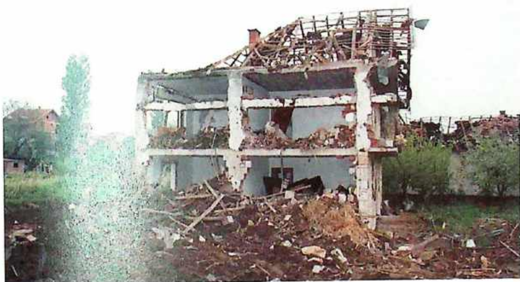
Photo 71 Demolished house of Svetolik Mladenović, 7b Bujmirska Street
