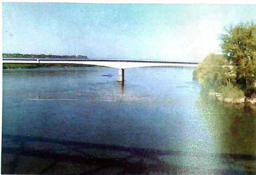
Photo 19 Road bridge across the Danube in Bogojevo, Sombor Municipality
