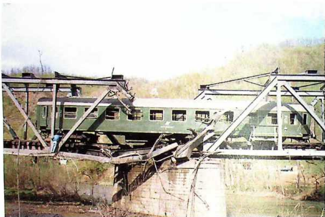
Photo 39 View and damage of the bridge and the fourth carriage
