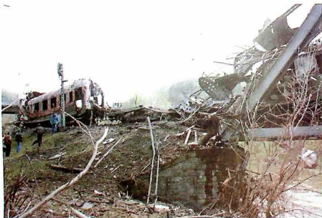
Photo 36 Close-up of damage of the second and third carriages
