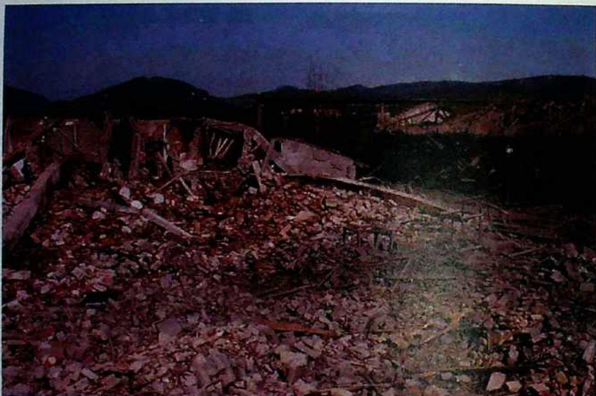
Photo 19 Demolished PVC manufacturing plant, "Milan Blagojević" Chemical Plants in Lučani
