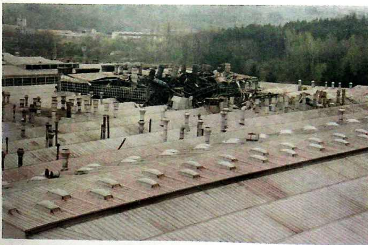
Photo 21 Broad view of damaged "Zastava" car factory in Kragujevac
