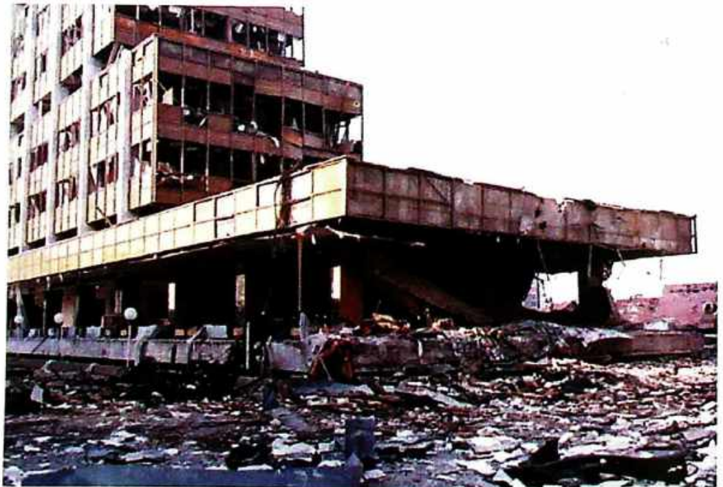
Photo 30 Damaged building of the National Bank in Priština, April 7, 1999
