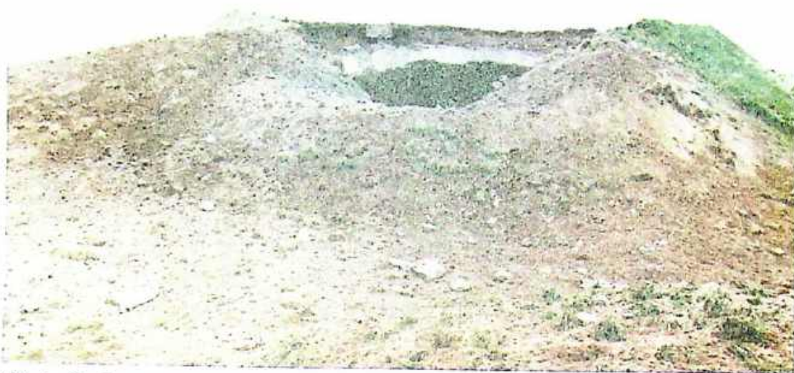
Photo 20 Destroyed oil storage tank No. 7 within the compound of NAP in Čonoplja, Sombor, 12/13 April 1999
