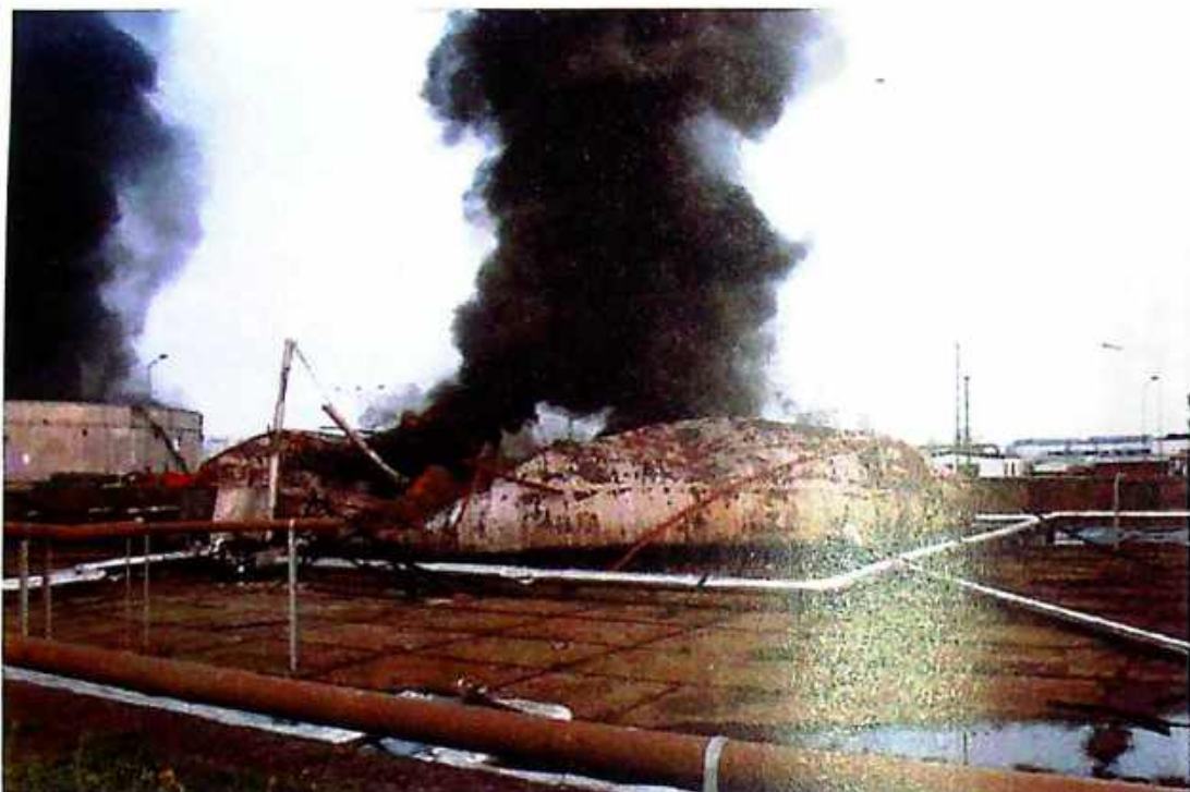
Photo 12 Burned oil storage tanks – "Beogradske elektrane", Novi Beograd
