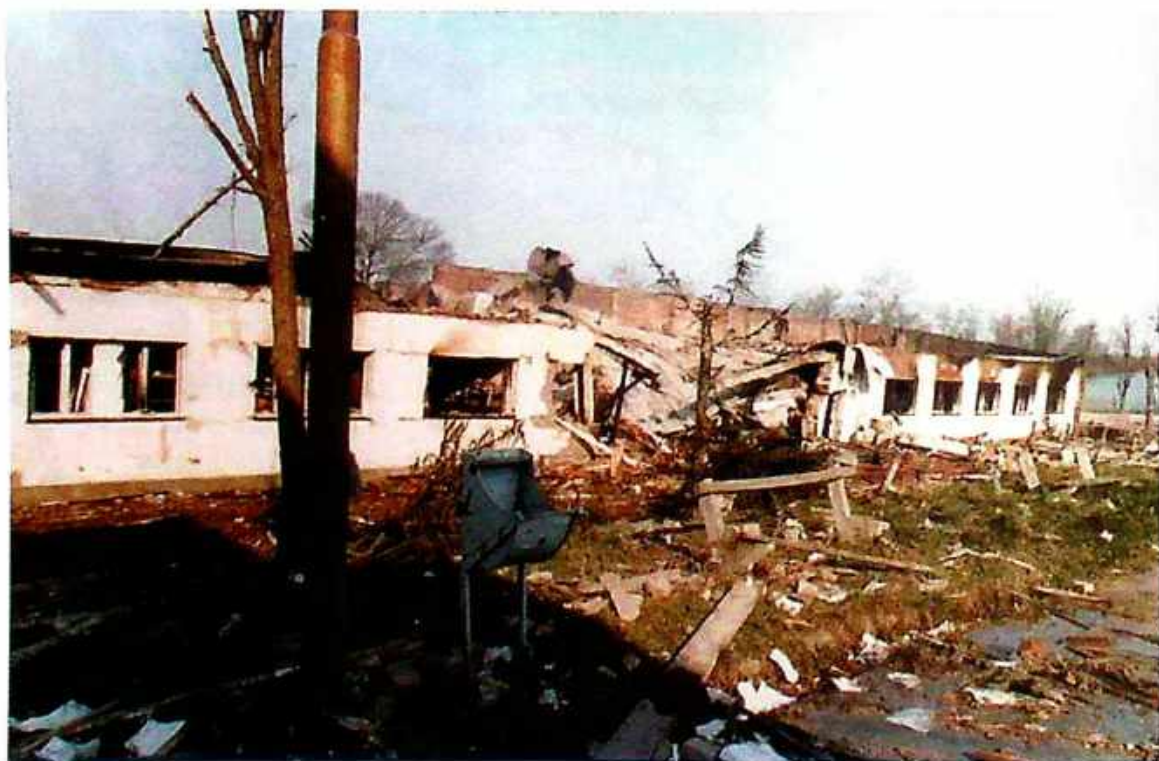
Photo 30 Damaged "Fuel 2" facility (stabilization furnace, atmospheric furnace and vacuum furnace)
