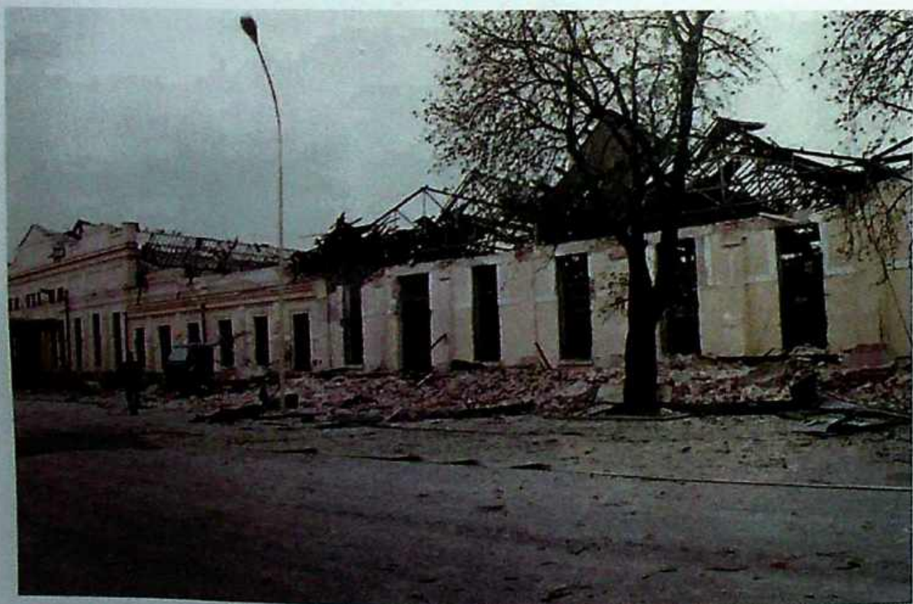
Photo 31 Demolished mechanical treatment plant "Zastava - Trucks"
