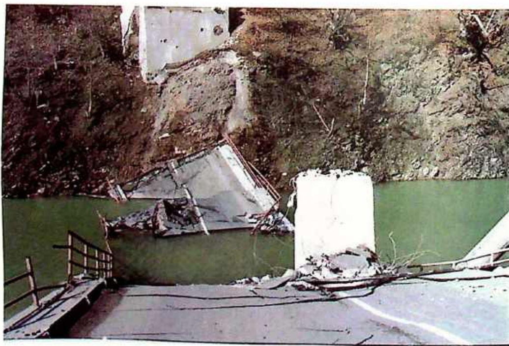
Photo 12 Close-up of the demolished bridge
