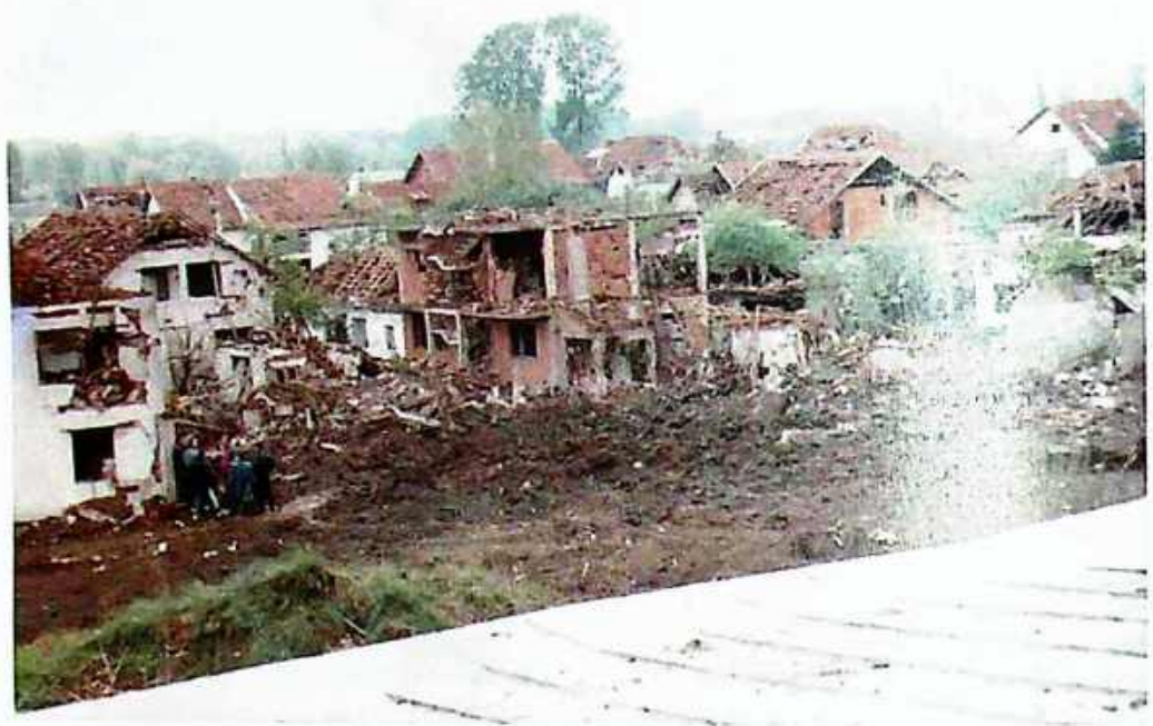
Photo 69 A view of the bombed civilian facilities in Šaka Estate in Niš, Bujmirska Street, where many houses were demolished on 19 April 1999
