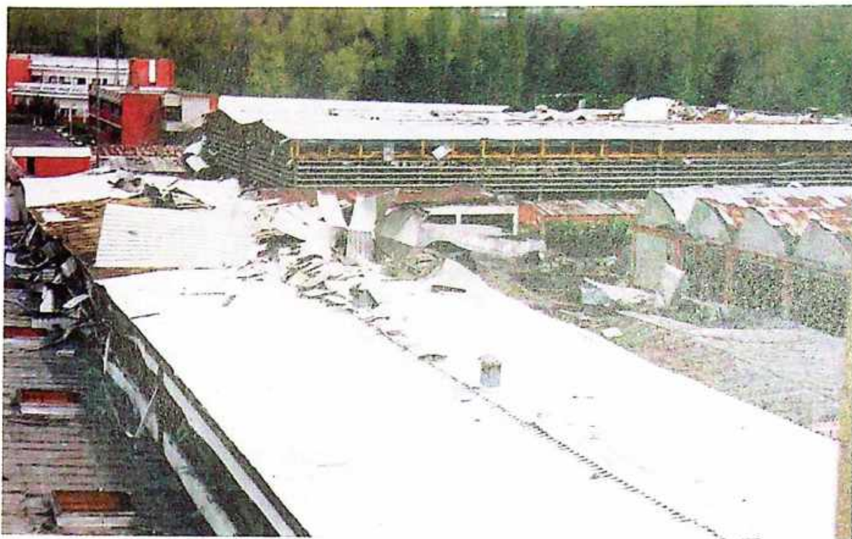
Photo 38 "Krušik" textile machines factory, point of impact on the roof, 14 April 1999
