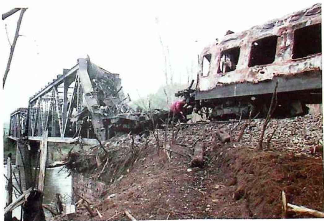
Photo 38 Close-up of damaged second and third carriages
