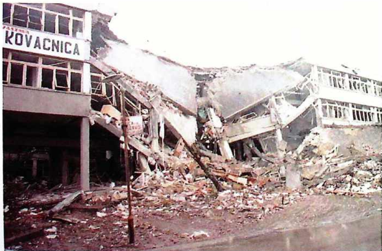
Photo 27 Demolished forging plant in "Zastava"
