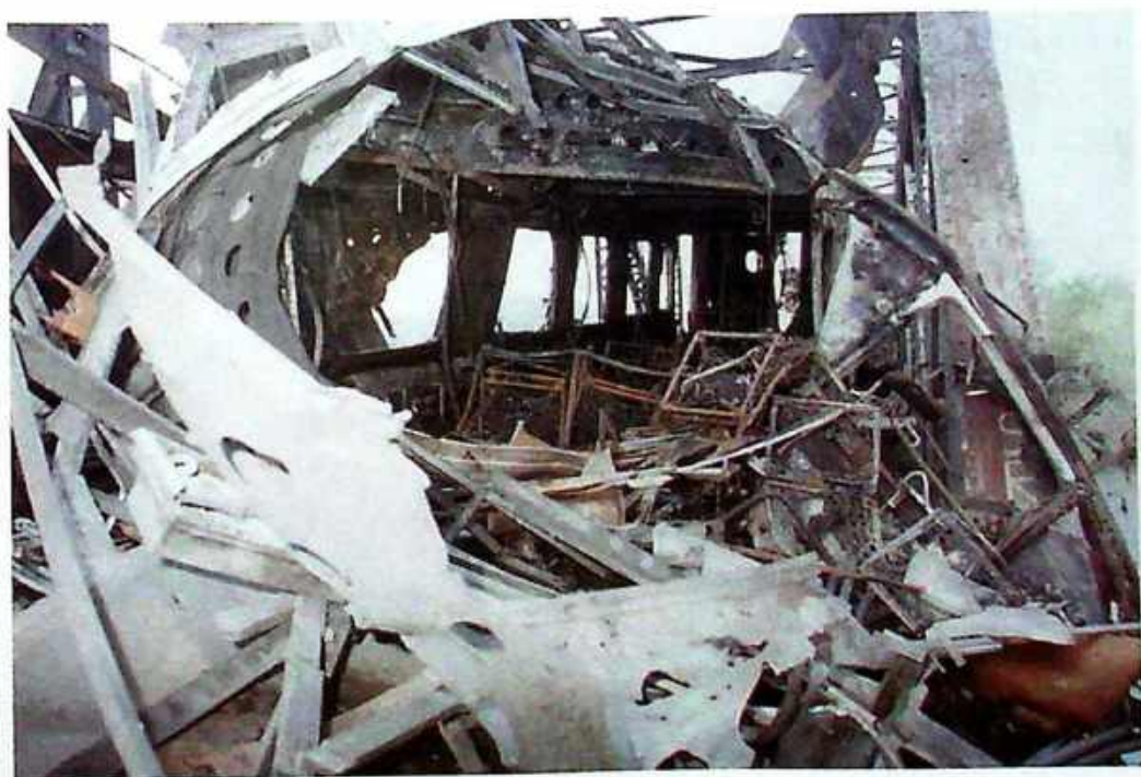
Photo 46 View and damage of the interior of the second carriage
