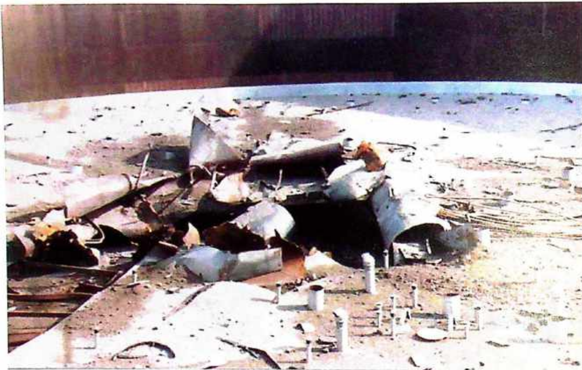
Photo 25 Crater made by airplane bomb in oil storage tank P-27
