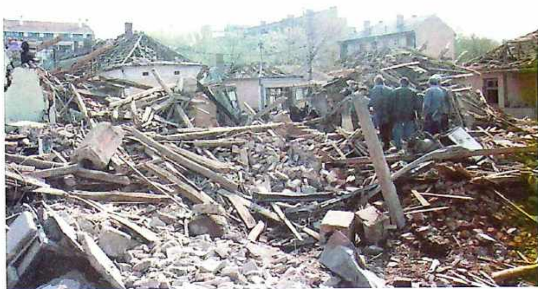
Photo 19 Close-up of damage on Dušan Trivunac St. in Aleksinac
