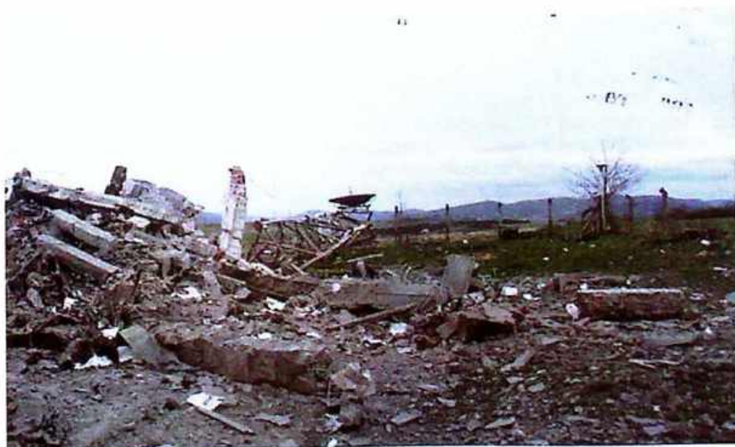
Photo 15 Destroyed PTT repeater on Gazimestan - Priština, 13 April 1999
