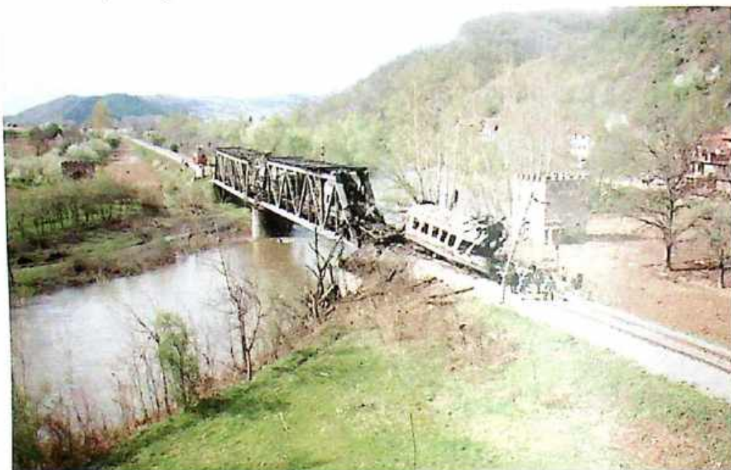
Photo 35 Broad view of the railway bridge and passenger train No. 393 attacked by NATO bombers
