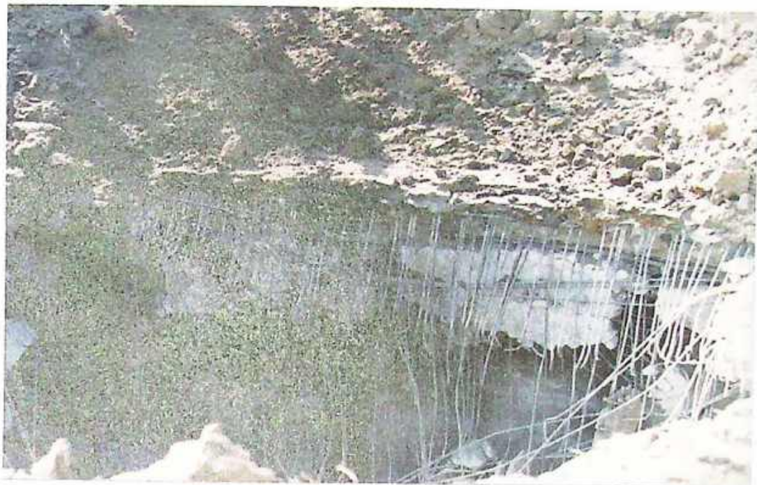
Photo 7 Crater made by a missile which hit the installations of NAFTAGAS - Čonoplja-Kljajicevo, 5/6 April 1999
