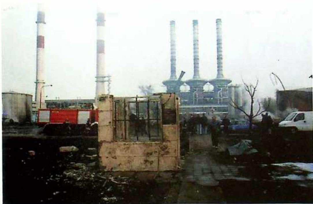
Photo 7 Destroyed guard's house and damaged heating plant "Beogradske elektrane" – Novi Beograd
