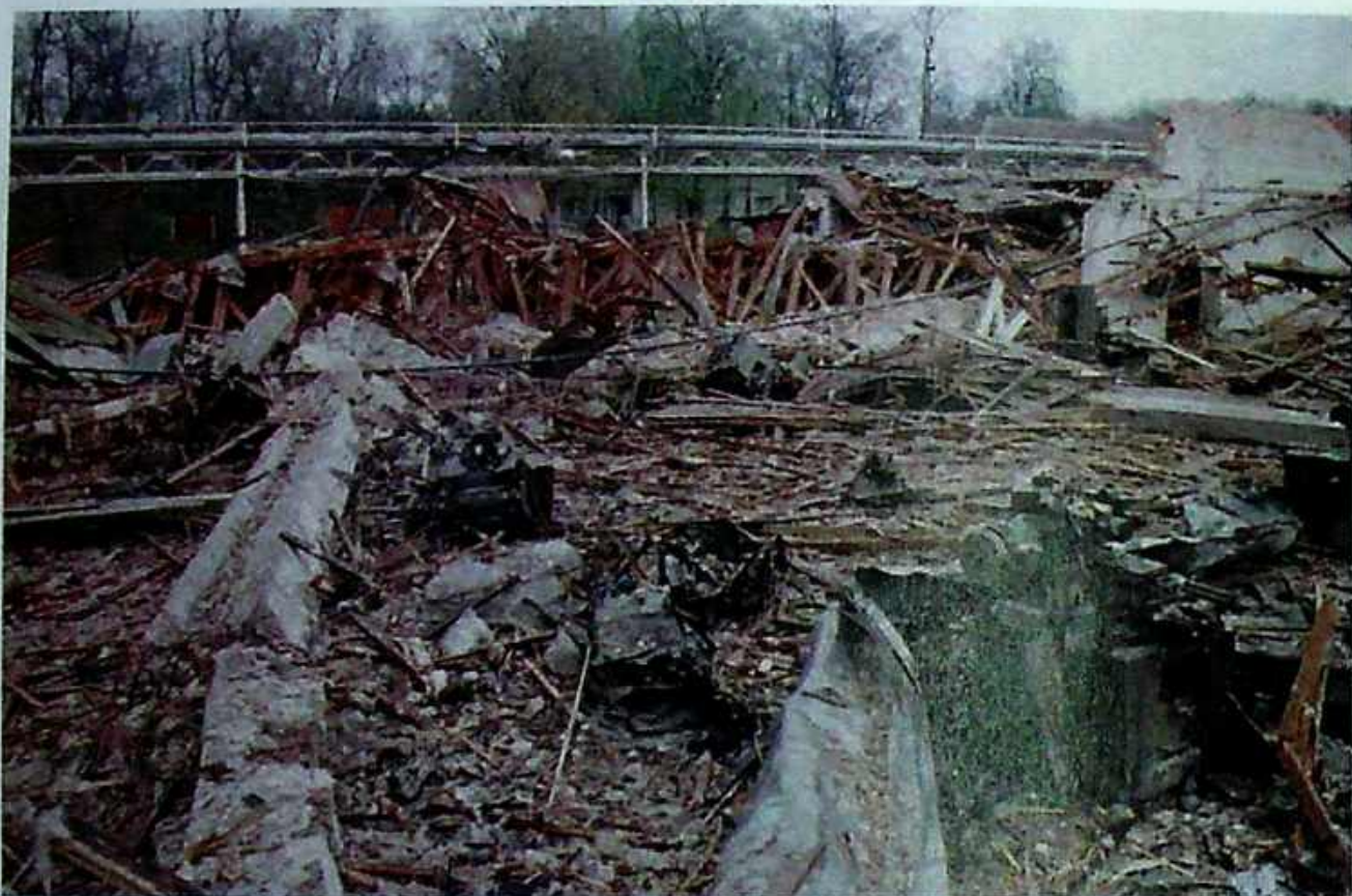
Photo 30 Close-up of the demolished "Tools" factory
