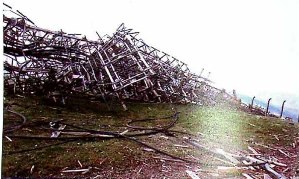
Photo 16 Demolished repeater aerial
