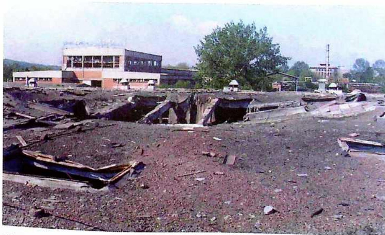
Photo 45 Point of impact on the roof of the Fittings and Fixtures Factory
