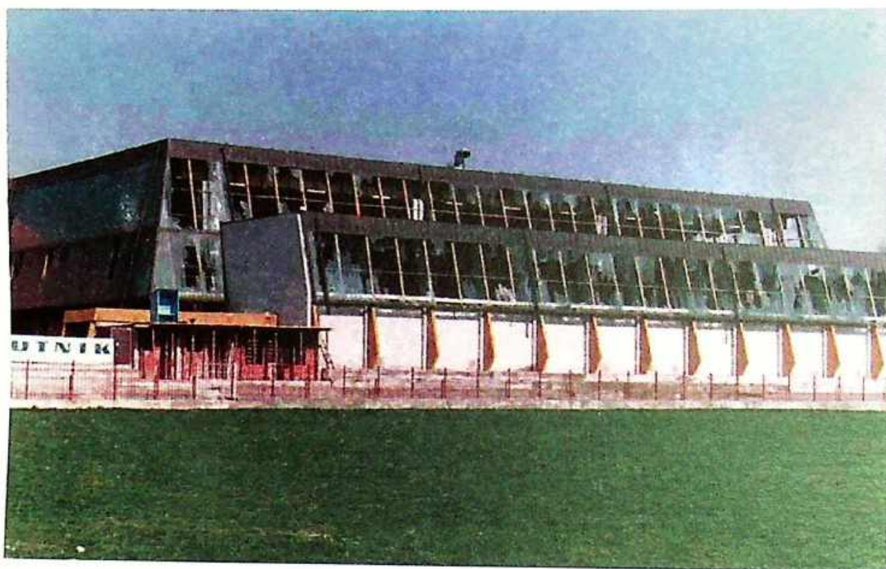
Photo 11 Damaged sports hall in Raška
