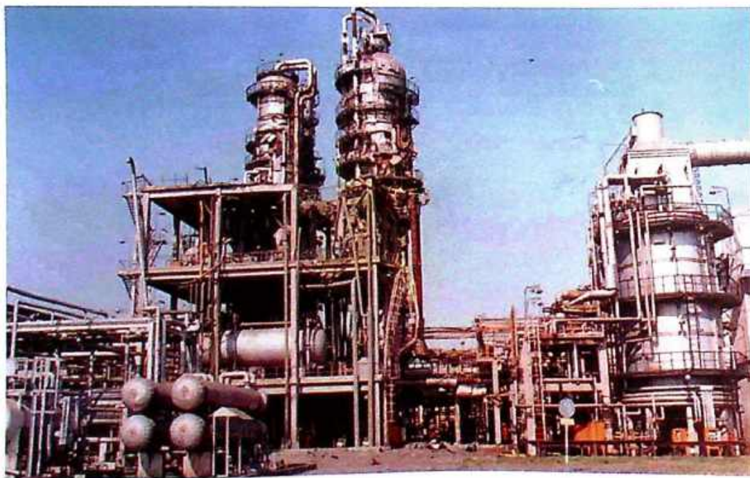
Photo 13 Damaged processing and non-processing installations in NIS, Novi Sad
