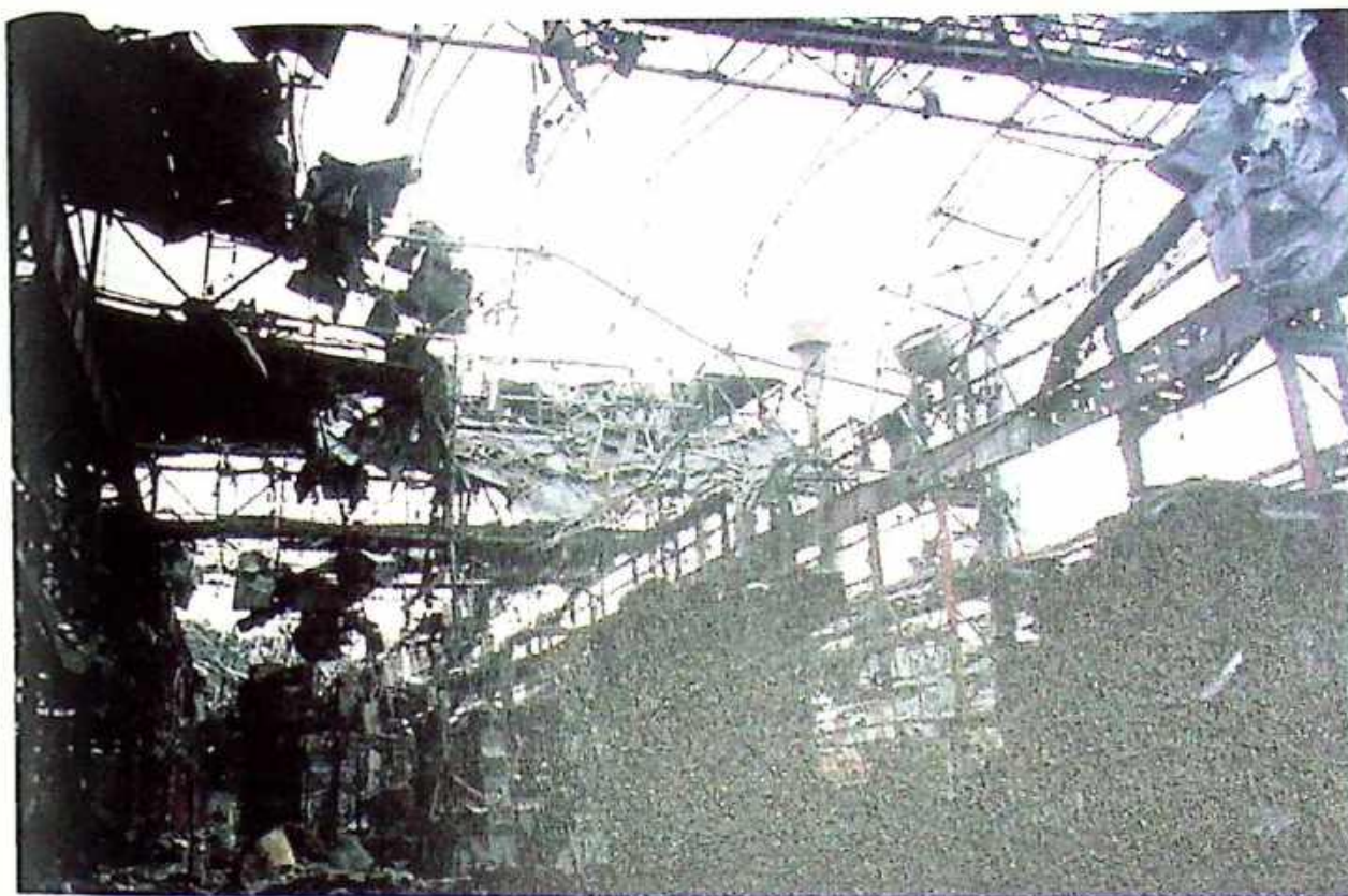
Photo 28 Inside view of the demolished forging plant
