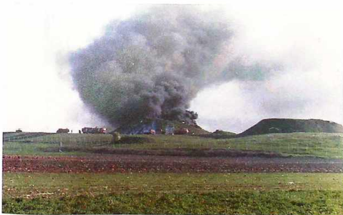
Photo 8 Targeted oil storage tank No. 3 of "Naftagas promet" in Čonoplja, Sombor, 6/7 April 1999
