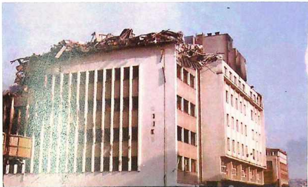
Photo 31 Damaged building of the provincial and municipal insurance company in Priština, April 7, 1999
