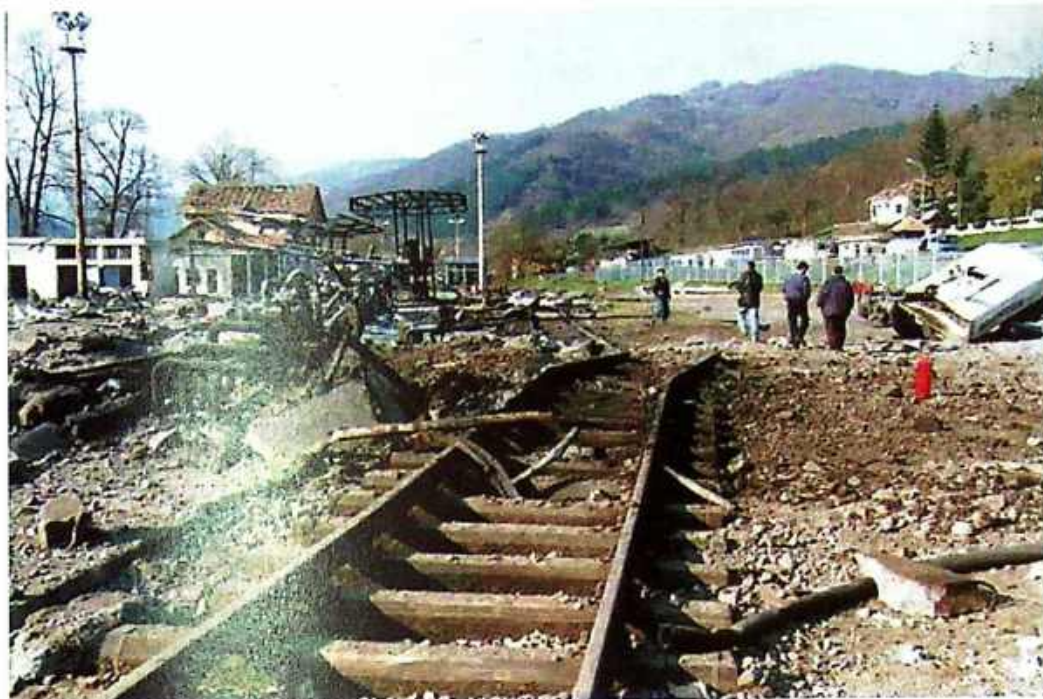
Photo 25 Damaged railway tracks, railway station and Beopetrol pumping station in Bogutovac, Kraljevo Municipality
