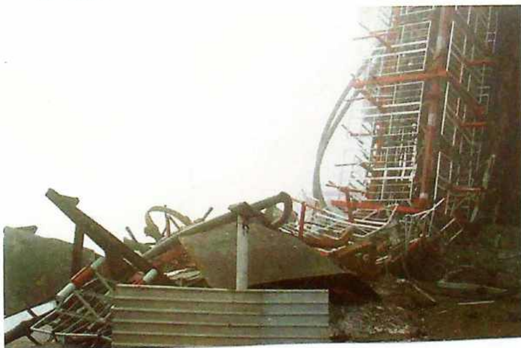
Photo 11 Destroyed relay station on Mt. Jastrebac
