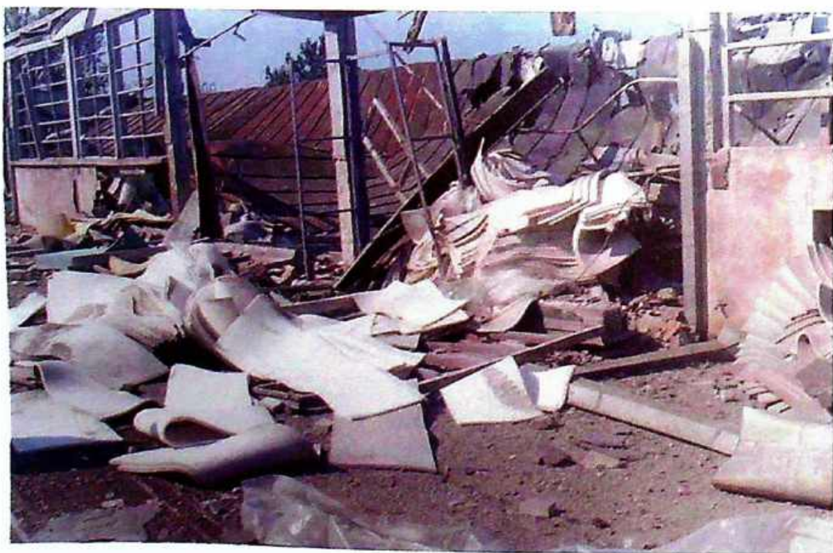
Photo 47 Demolished production plant of the Polyurethane Factory
