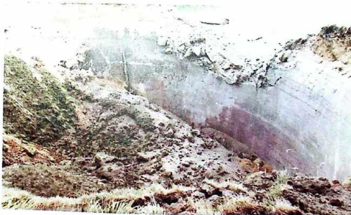
Photo 21 Close-up of destroyed oil storage tank No. 7
