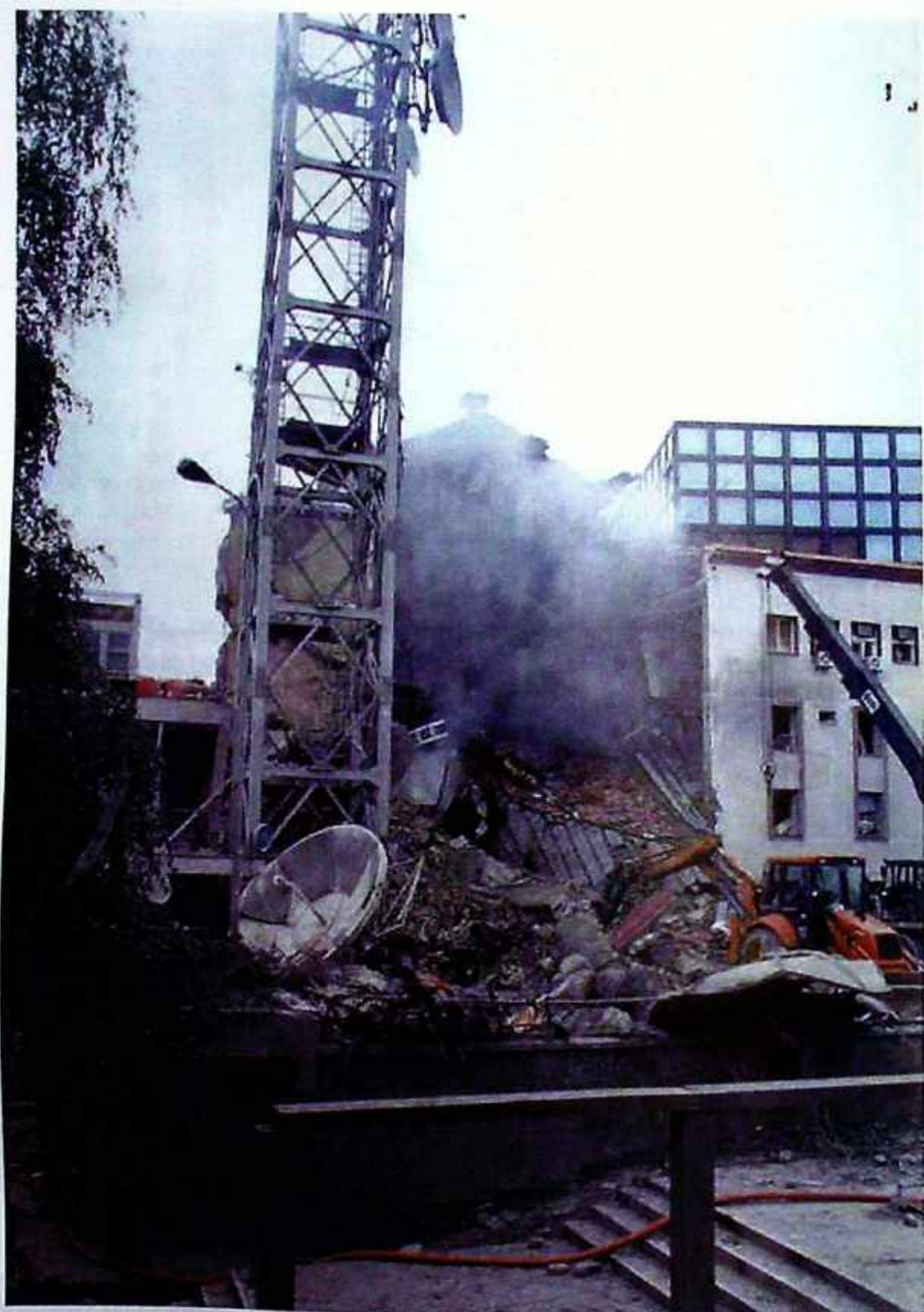
Photo 34 Close-up of RTS demolished office building seen from the direction of "Duško Radović" theater
