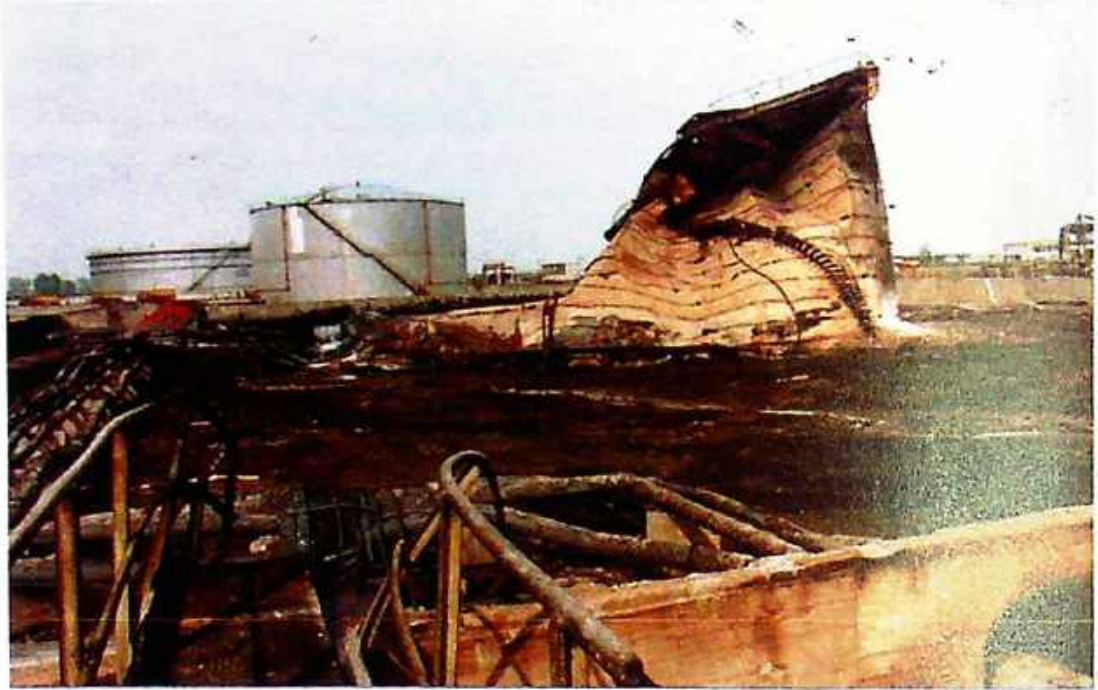
Photo 15 Damaged facilities of NIS "Jugopetrol", Smederevo
