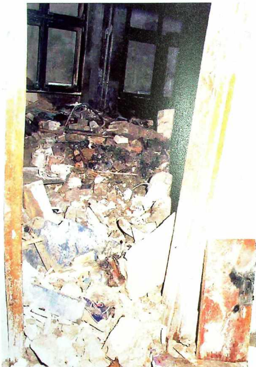
Photo 37 View of demolished make-up room
