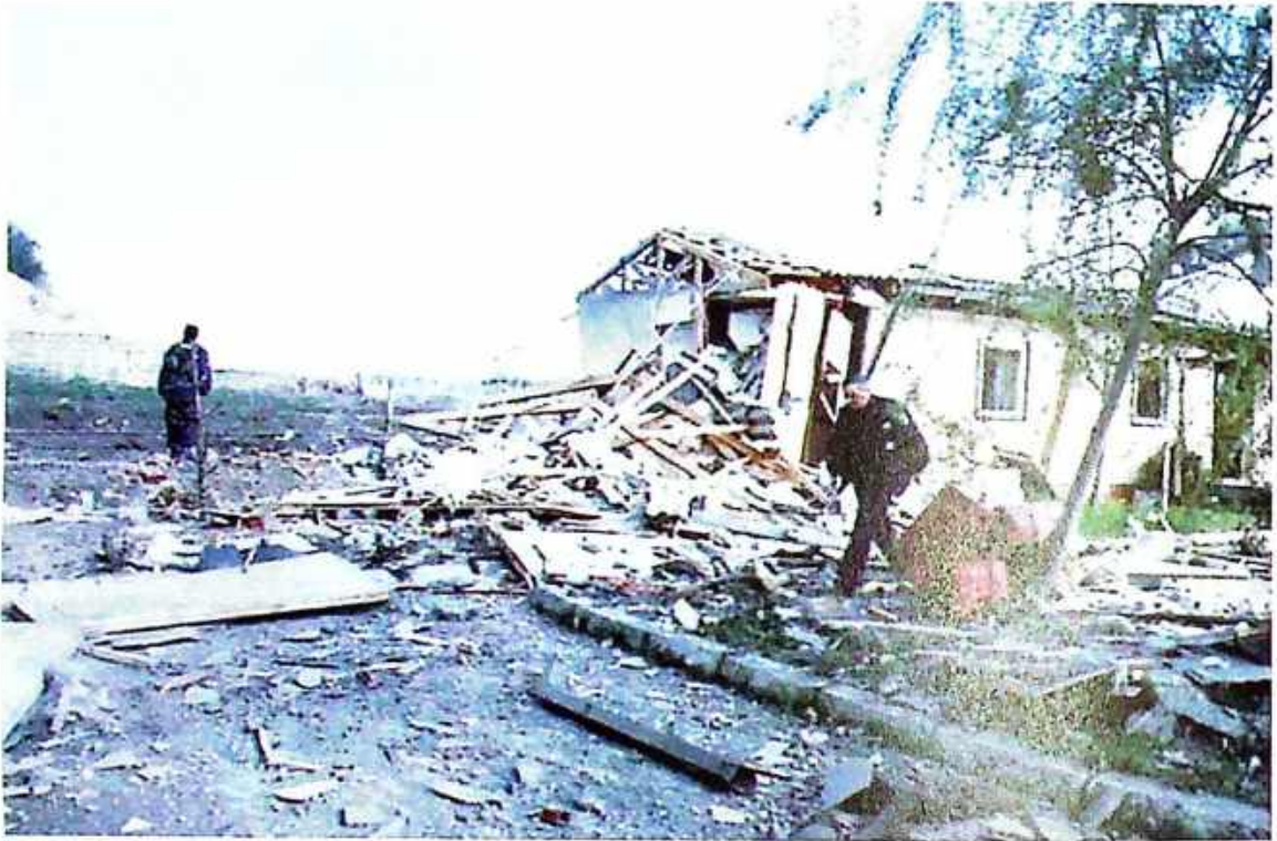
Photo 37 Demolished "Magistrala" road maintenance enterprise in Priština, 13 April 1999
