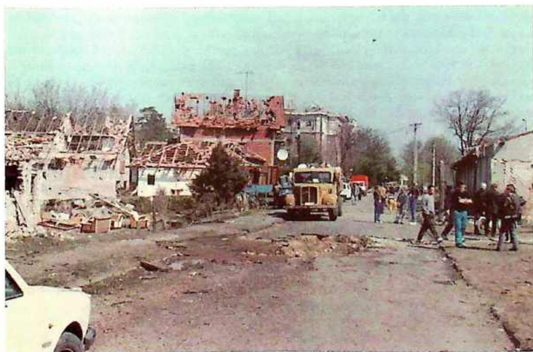
Photo 43 Damaged houses, Bulevar vojske Jugoslavije St. in Čuprija
