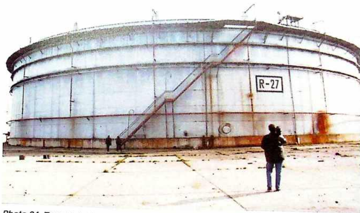
Photo 24 Targeted oil storage tank P-27 NIS "JUGOPETROL" in Smederevo, 13/14 April 1999
