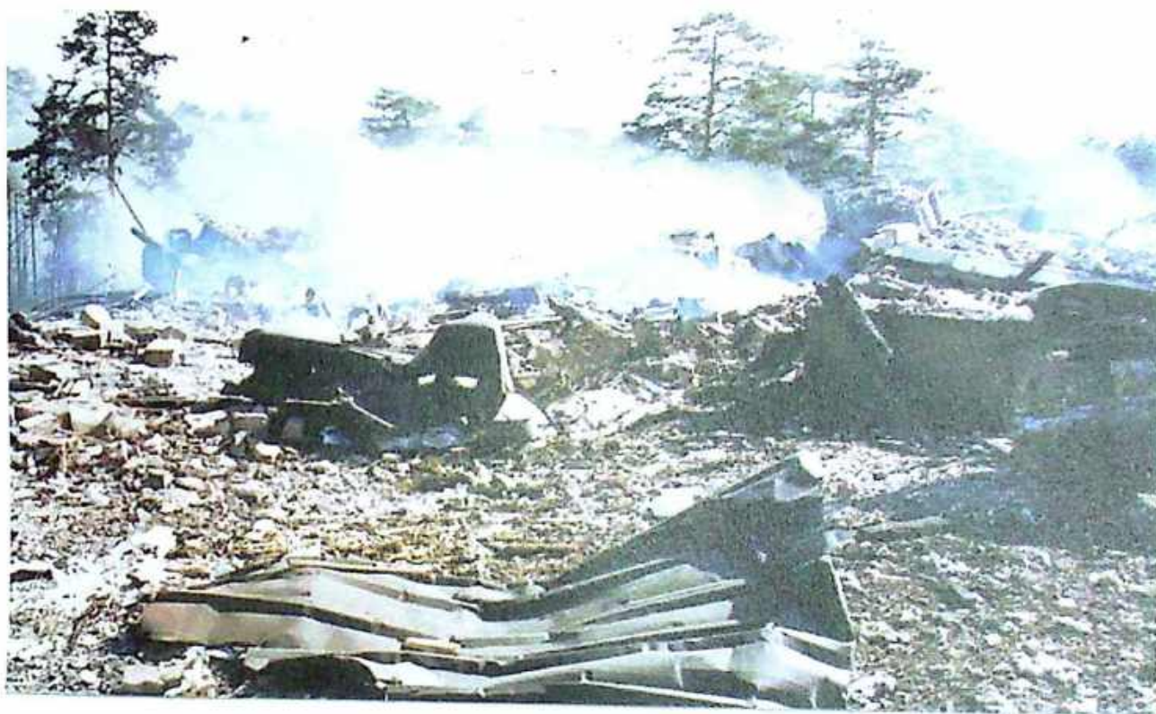
Photo 4 Site of burned Children's Rehabilitation Center (60 beds) and a three-storey hotel and restaurant
