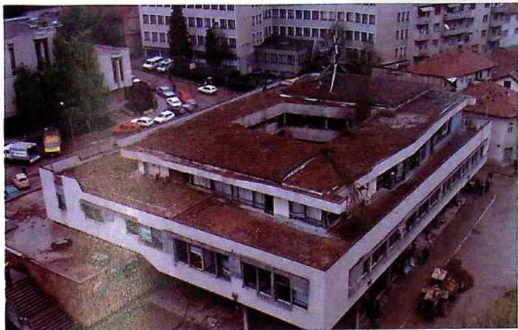
Photo 67 General view of the JP PTT and Telekom Serbia Building in Užice, hit by a missile through the central roof shaft on 22 April 1999
