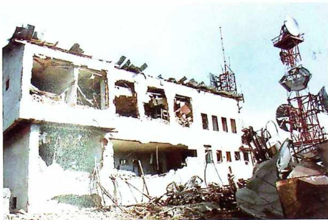
Photo 14 Demolished building of RTS repeater on Mt. Goleš - Priština, 9/10 April 1999
