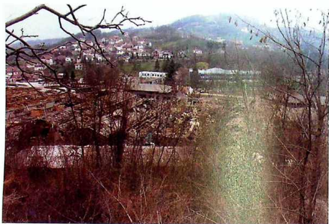
Photo 5 Broad view of the damaged "Sloboda" factory in Čačak
