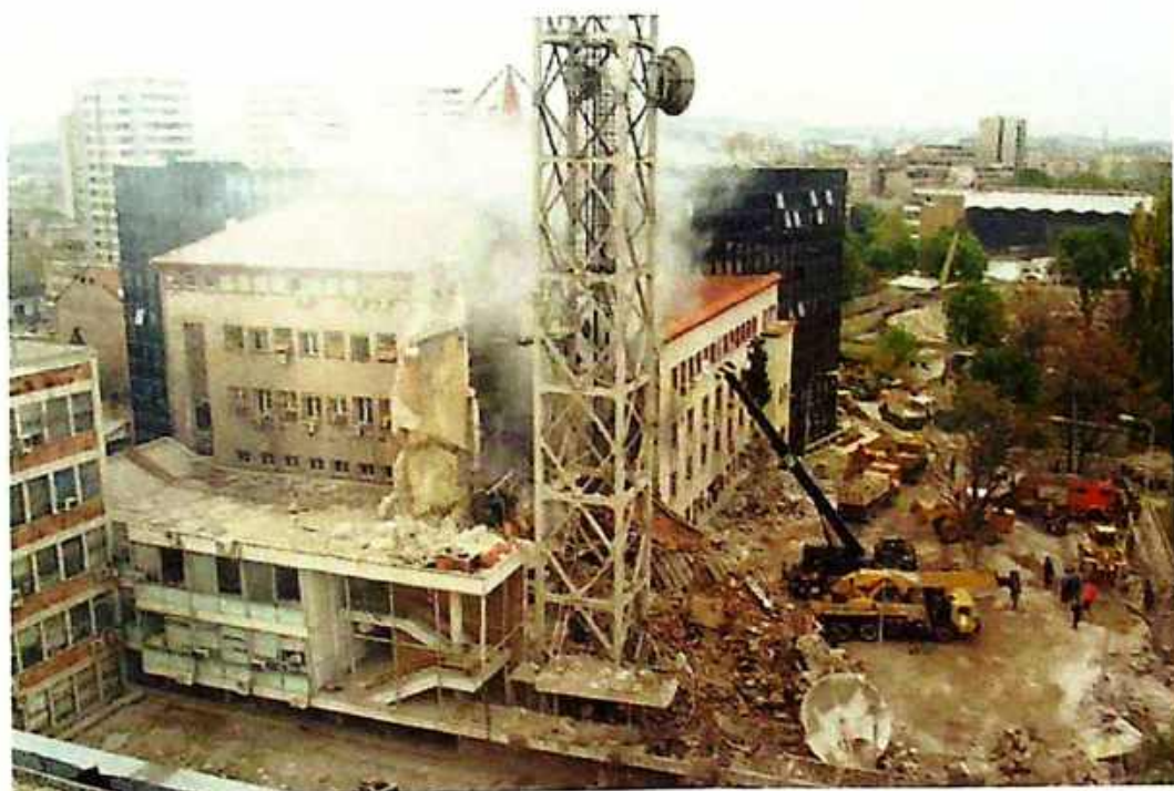
Photo 33 Broad view of demolished RTS office building at 1 Aberdareva Street, 23 April 1999
