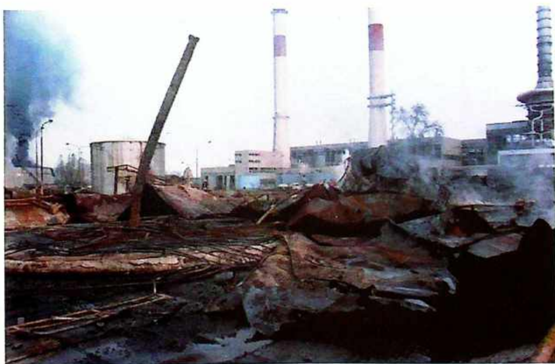
Photo 11 Burned oil storage tanks – "Beogradske elektrane", Novi Beograd
