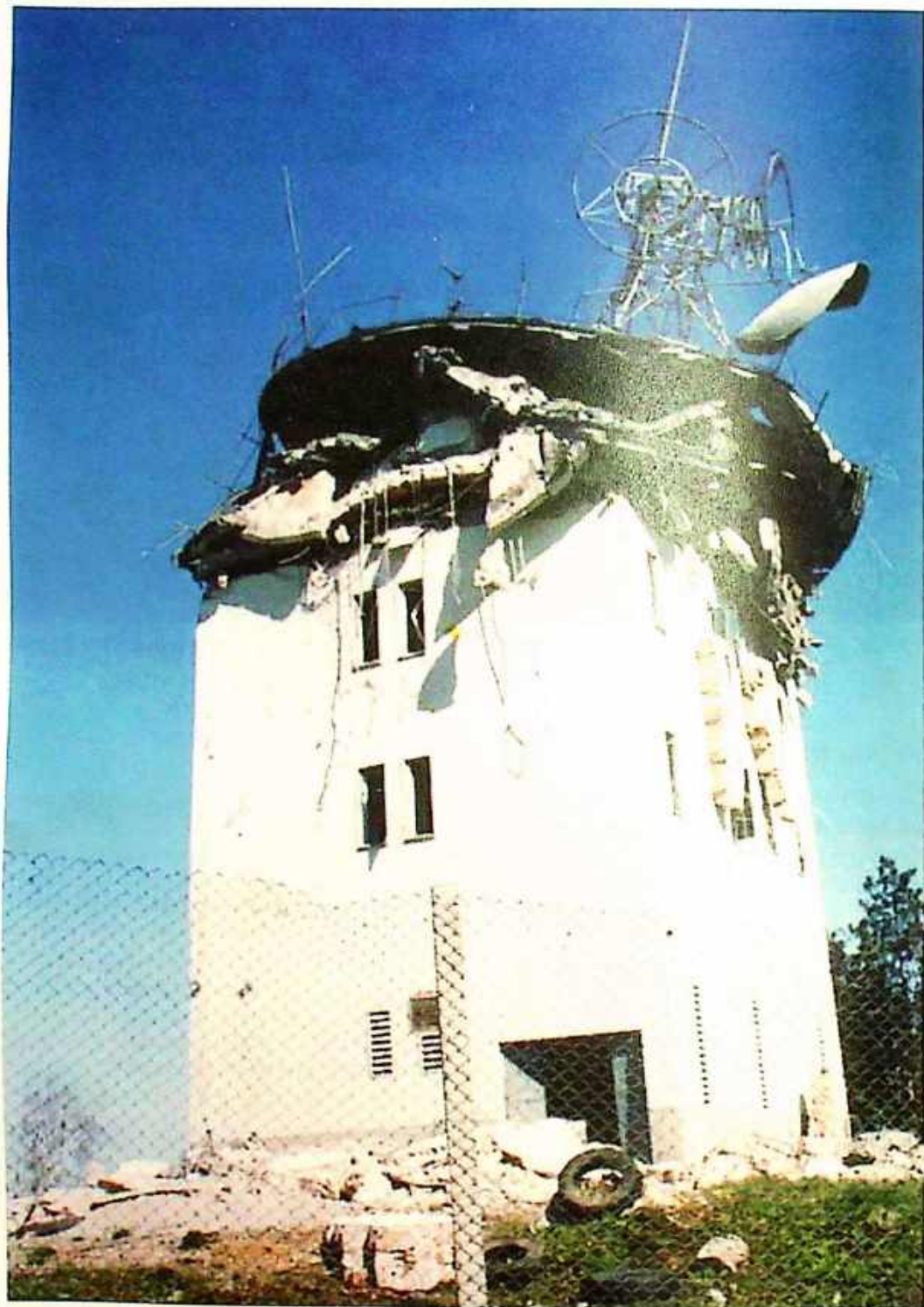
Photo 18 Demolished building and the transmitter antenna of Telekom Srbija on Mt. Jagodnja near Krupanj – Šabac, 15 April, 1999
