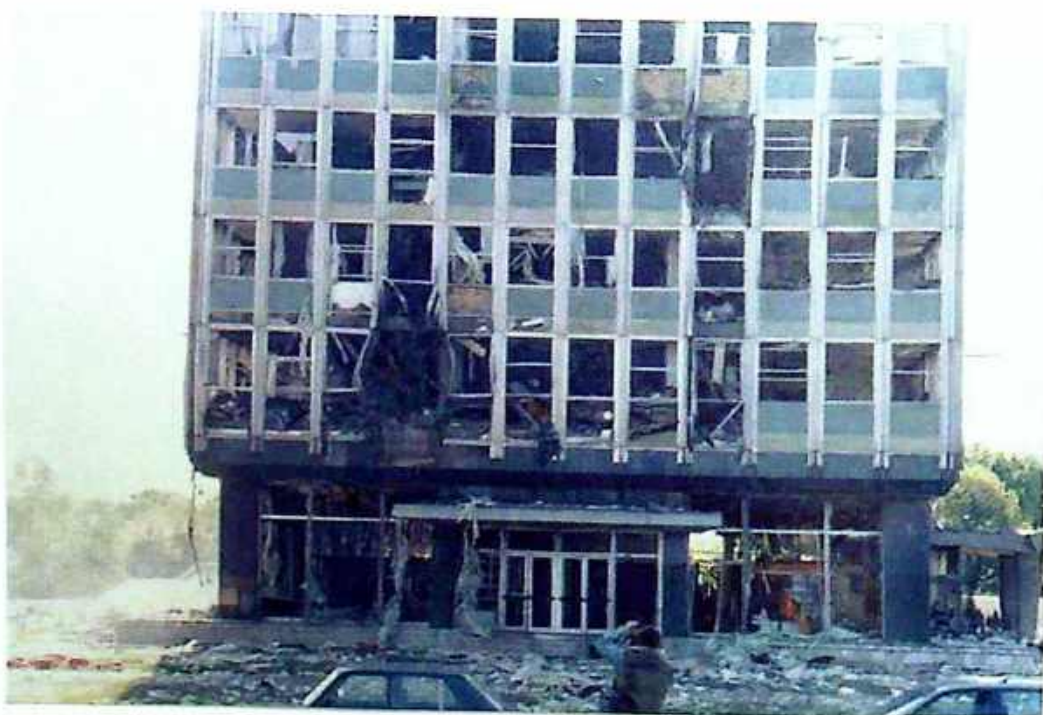
Photo 24 Sites on the first and fourth floors where the missiles landed
