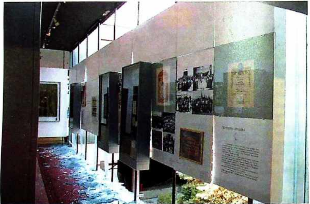
Photo 1 Damage in the exhibition area of the Vojvodina Museum in Novi Sad, 1 April 1999
