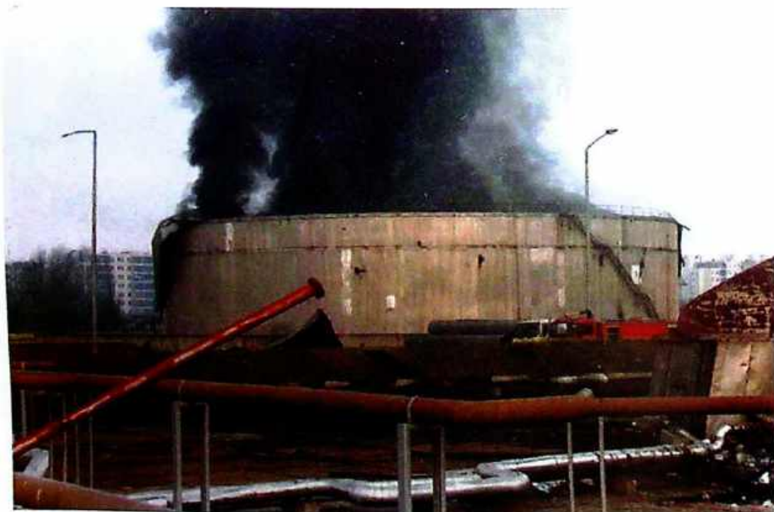
Photo 13 Damaged oil storage tank – "Beogradske elektrane", Novi Beograd
