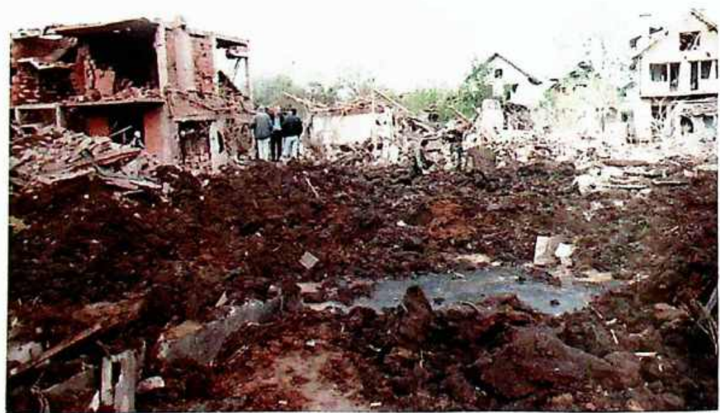
Photo 70 A close-up of the crater in Bujmirska Street
