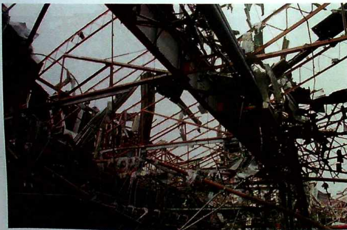
Photo 23 View of demolished paint shop
