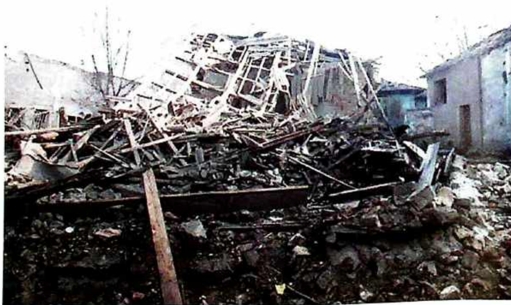
Photo 38 Completely destroyed house on Zanatska St.
