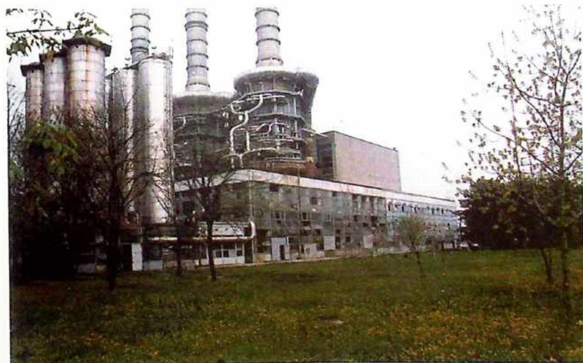
Photo 15 Lateral view of the damaged heating plant – "Beogradske elektrane", Novi Beograd
