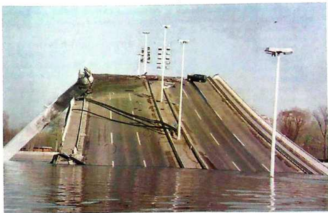
Photo 8 View of the sunken bridge from the Novi Sad side
