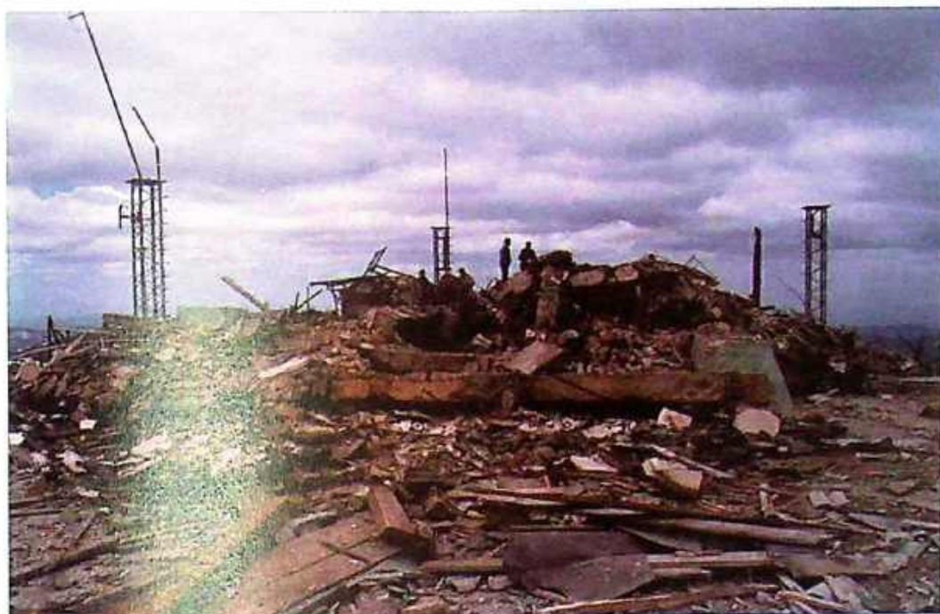
Photo 10 Destroyed relay stations on Ćigota, municipality of Čajetina
