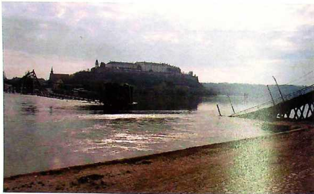
Photo 1 Demolished Varadin Bridge (facing the fortress)
