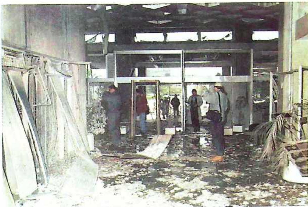
Photo 25 Demolished entrance to "Ušće" business center , 22 April 1999
