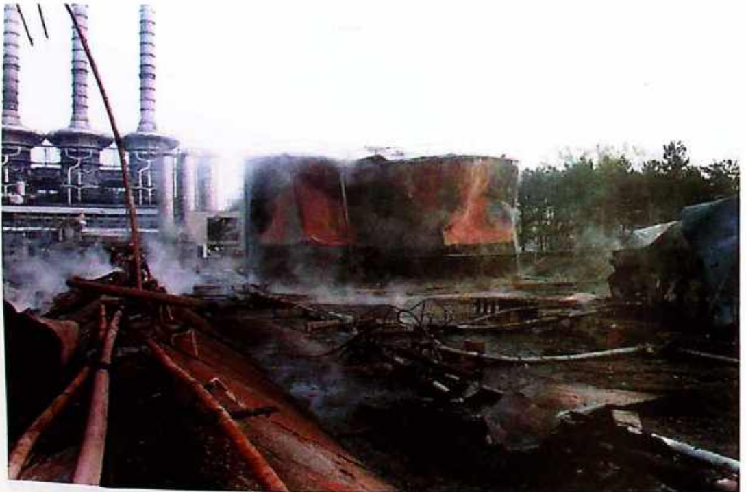
Photo 9 Burned oil storage tanks – "Beogradske elektrane", Novi Beograd
