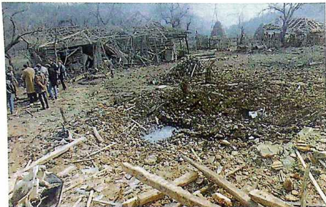
Photo 9 Missile crater and damaged auxiliary buildings owned by Veroljub Stevanović, Kuršumlija municipality
