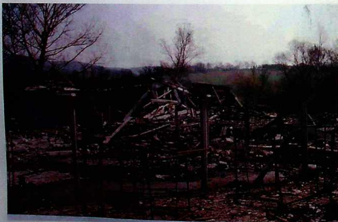
Photo 20 Demolished CIP workshop, "Milan Blagojević" Chemical Plants in Lučani
