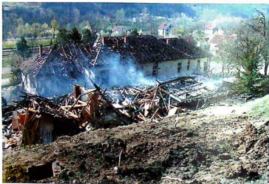
Photo 1 Demolished new school building and damaged old school building, Elementary School "Djura Jakšić", Bogutovac
