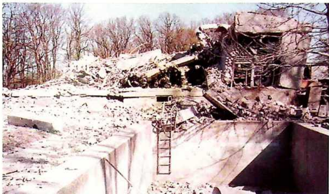
Photo 4. Close-up of damaged "Crveni Čot" TV transmitter facilities
