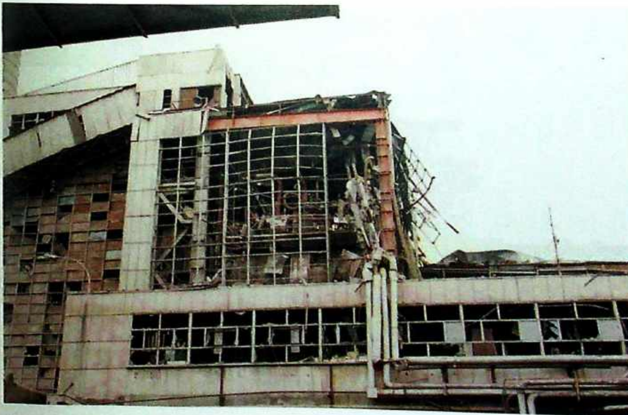
Photo 25 Demolished power plant in "Zastava"
