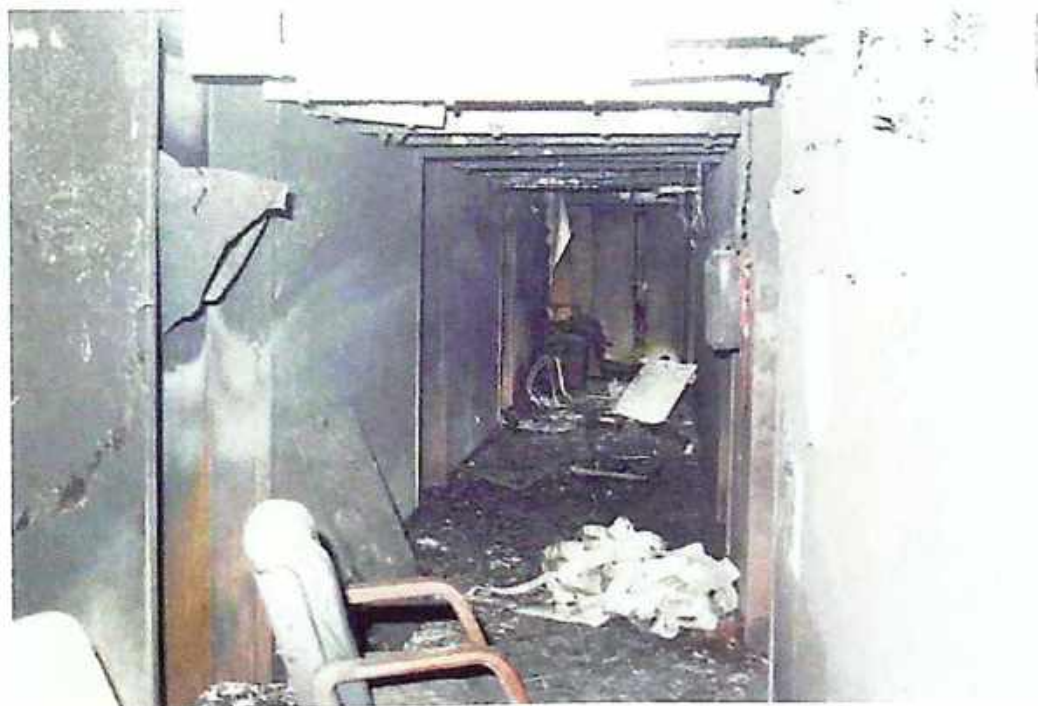
Photo 30 Demolished premises of RTV "Pink" on the 19th floor of "Ušće" business center
