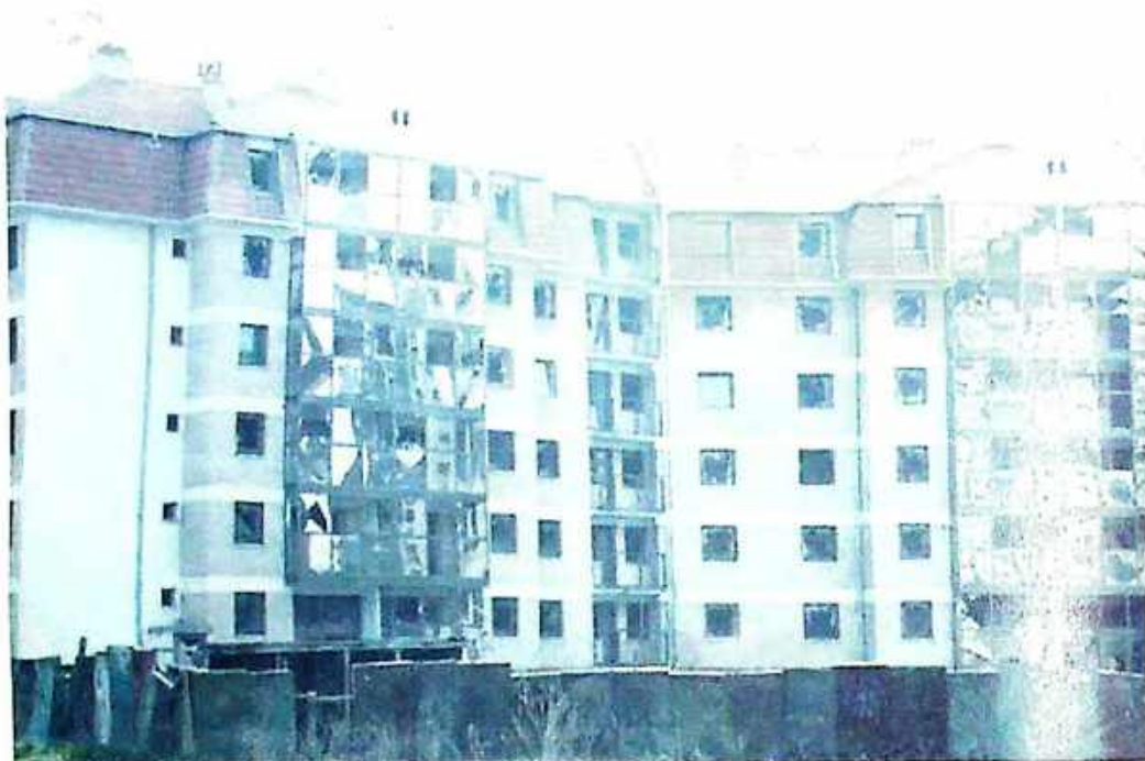
Photo 37 Damaged apartment buildings in Dardanija estate in Priština, April 13, 1999
