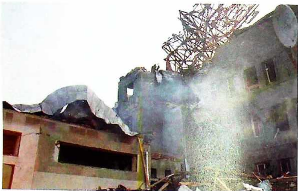
Photo 6 View of the demolished facility and aerial system
