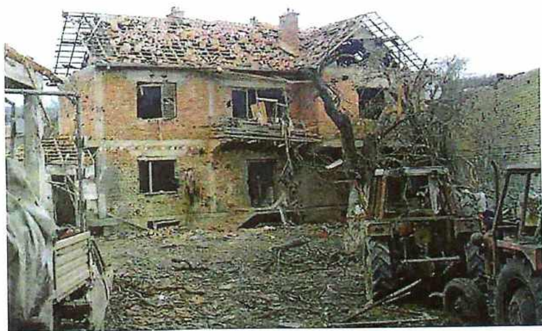
Photo 4 Demolished house, yard and farm machinery in the village of Nogovac where an unidentified woman's body was found
