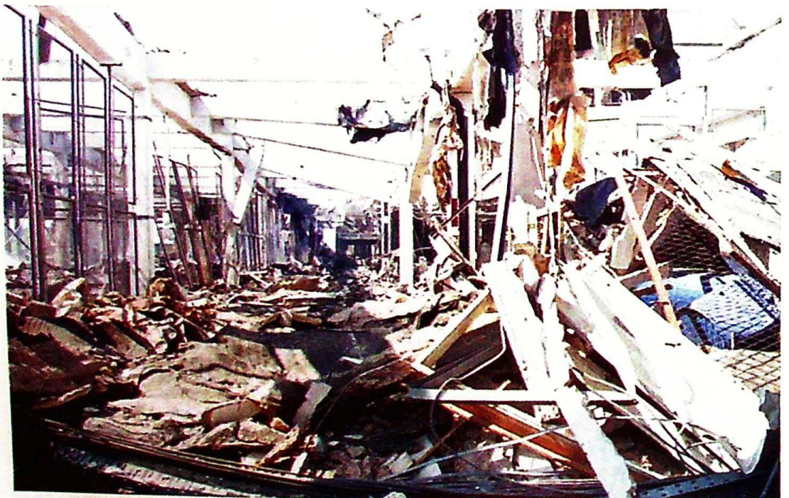
Photo 37 View of the destroyed "Blending Oil" facility of Novi Sad oil refinery, June 9, 1999
