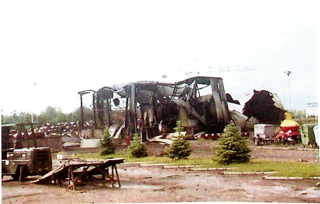
Photo 12 Close-up of the destroyed warehouses and oil storage tanks of NIS "Jugopetrol" Niš, May 11, 1999
