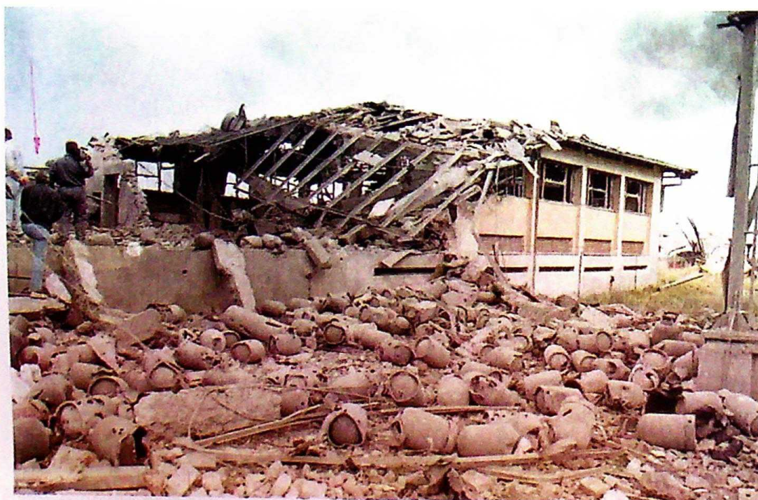
Photo 10 Demolished filling plant for TNG gas of NIS "Energogas"
