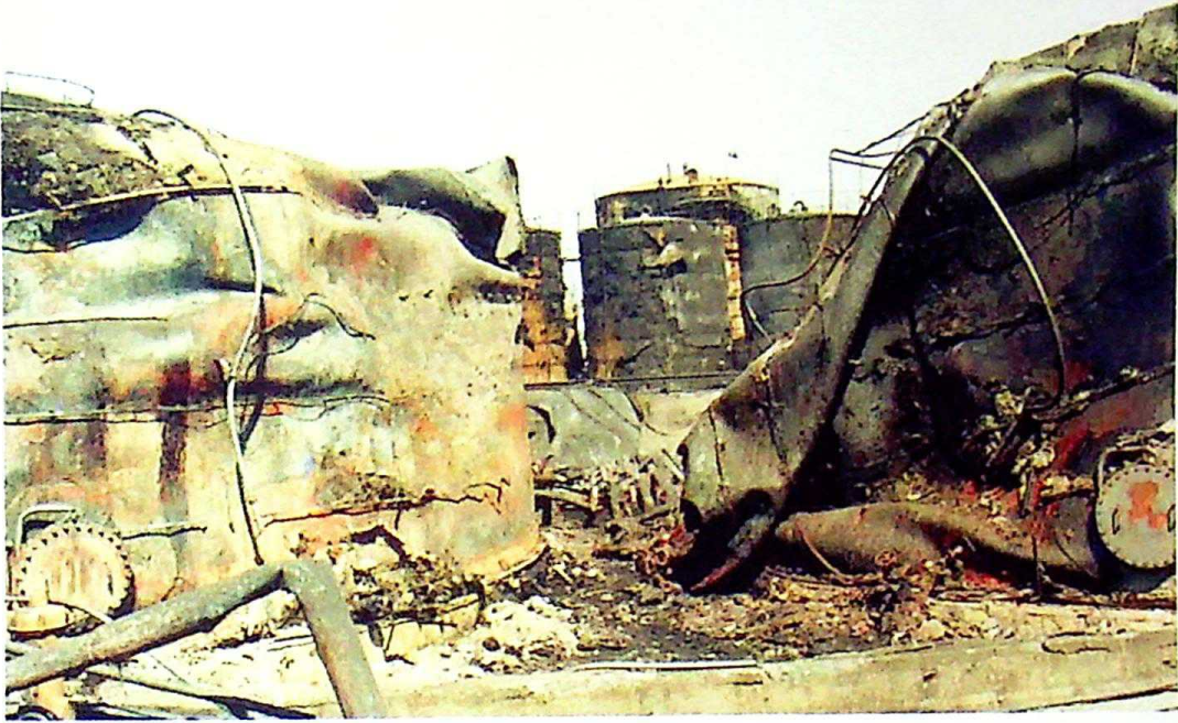
Photo 34 Close-up of the destroyed oil storagetanks of Novi Sad oil refinery, June 9, 1999
