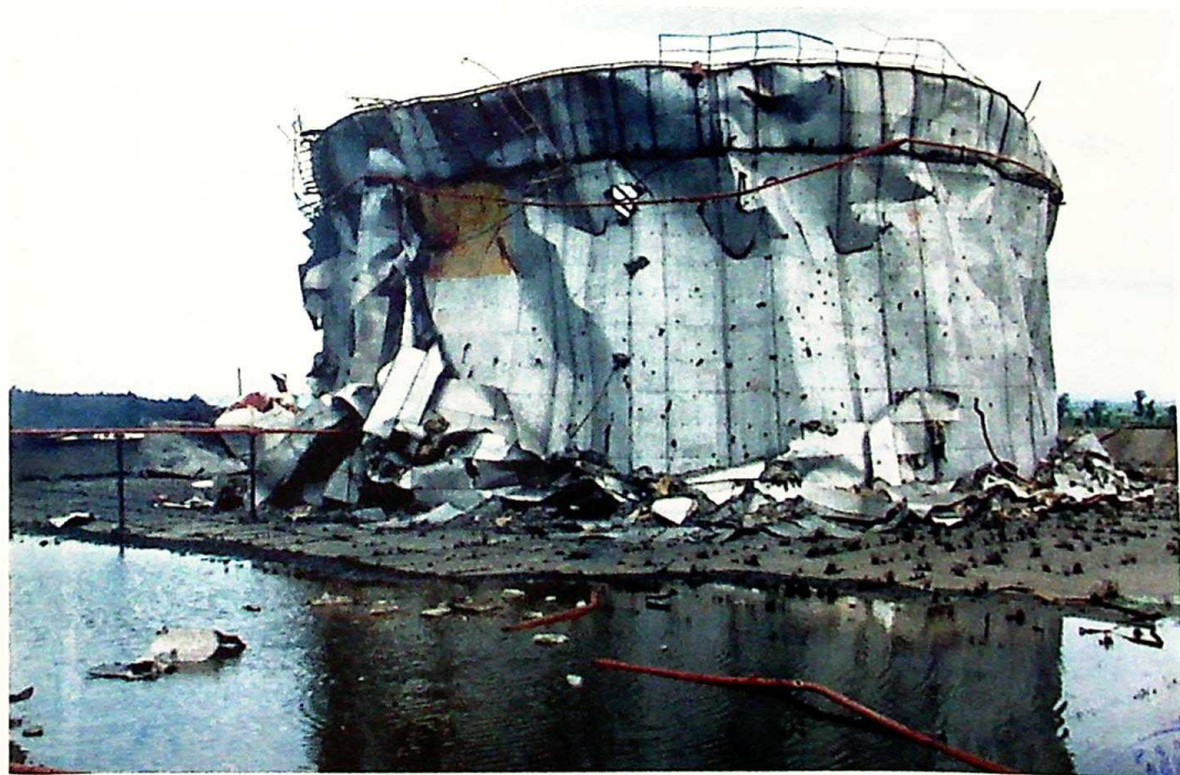
Photo 19 Destroyed oil storage tank R-6 of "Jugopetrol" – Beograd, Prahovo-Bor installation, May 17, 1999
