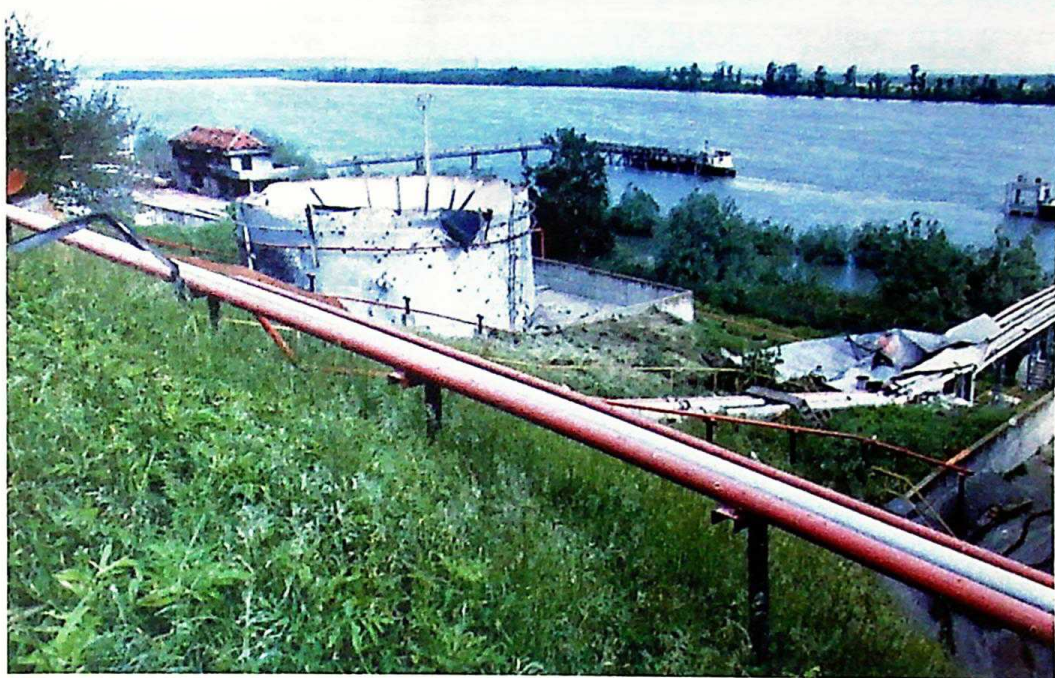
Photo 18 Destroyed oil storage tanks of "Jugopetrol" – Beograd, Prahovo-Bor installation, May 17, 1999 (2nd attack)
