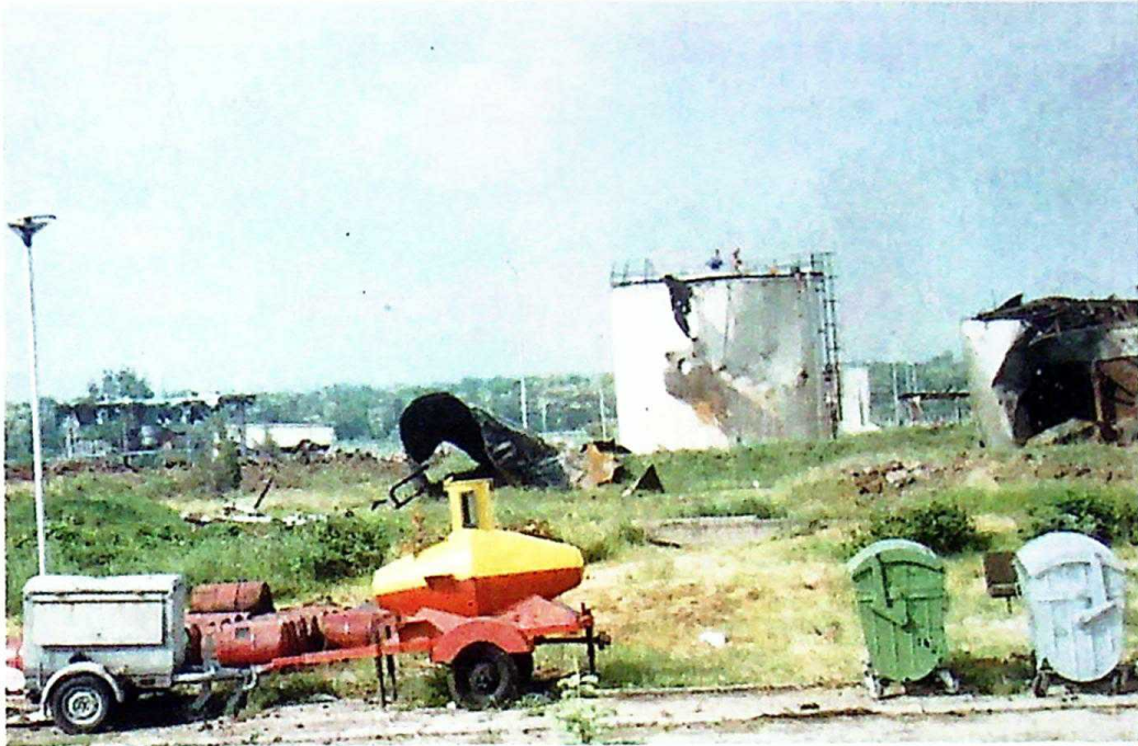
Photo 11 Broad view of the demolished fuel storage tanks of NIS "Jugopetrol" – Niš, May 11, 1999
