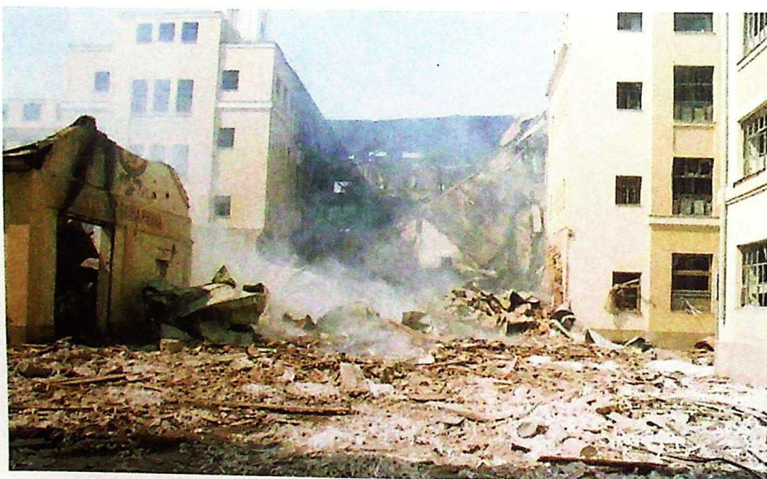
Photo 58 Demolished section of the old factory and auxiliary workshops of Niš Tobacco Industry
