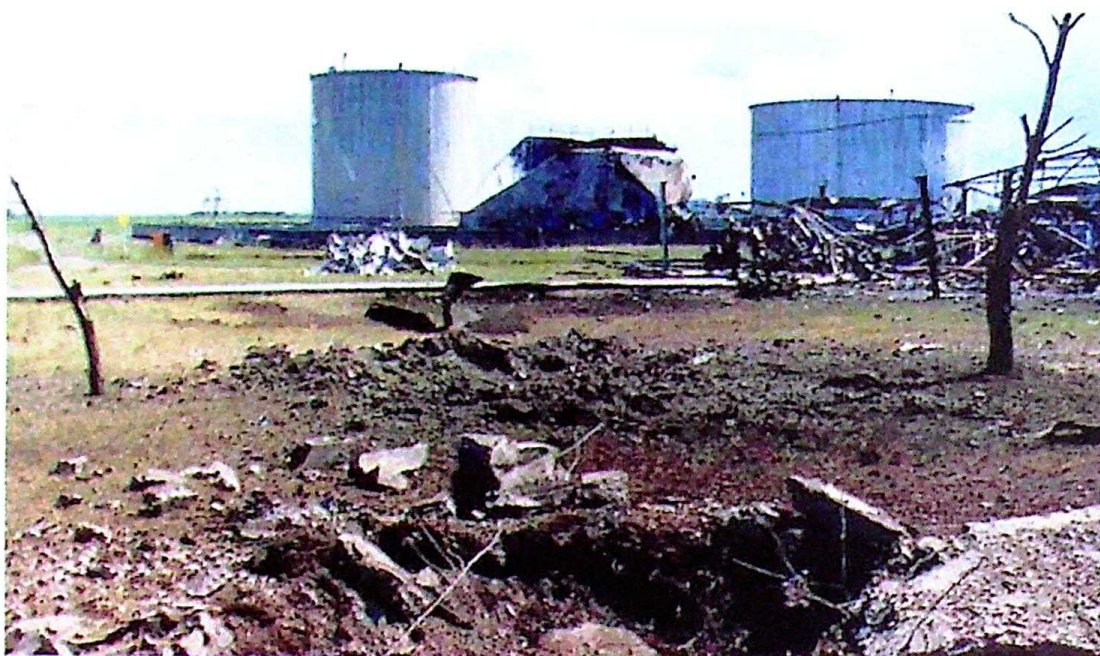
Photo 24 A crater surrounded by the destroyed pump station, vehicle reloading point and oil storage tanks in the storage area of NIS "Naftagas promet" in Sombor, May 21, 1999 (repeated attack)
