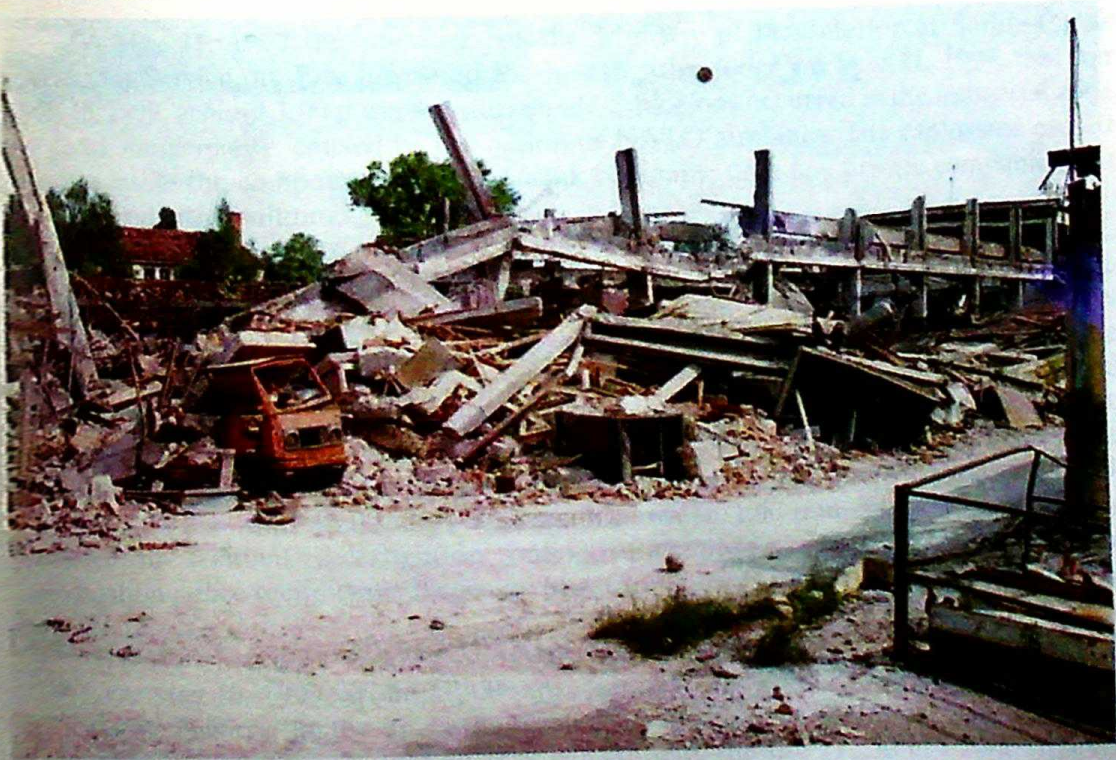
Photo 14 View of the demolished blacksmith's workshop of "Cer" factory
