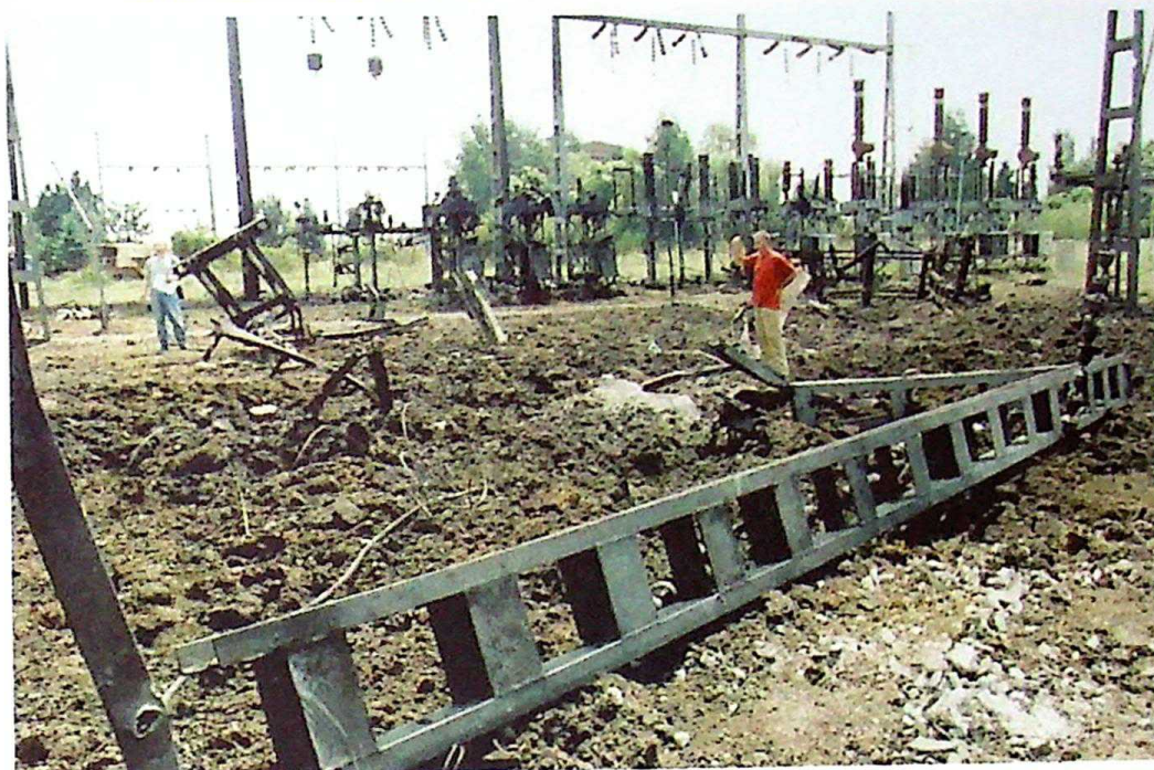
Photo 59 Destroyed transformer station installation on Rimski šančevi, May 31, 1999
