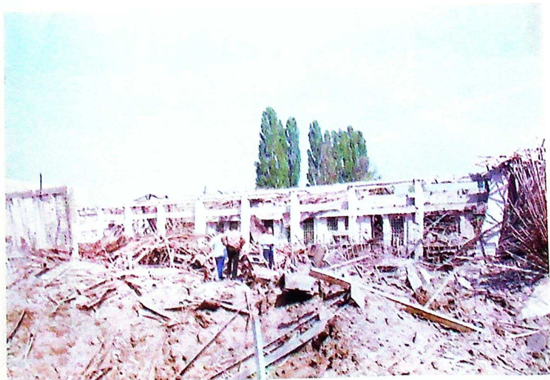
Photo 8 Demolished steel material warehouse of HK "Krušik", Valjevo, May 2, 1999
