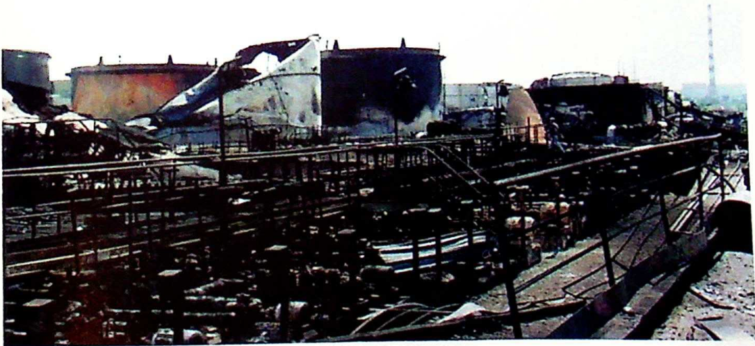
Photo 35 Destroyed pipeline installation and oil storage tanks of Novi Sad oil refinery, June 9, 1999
