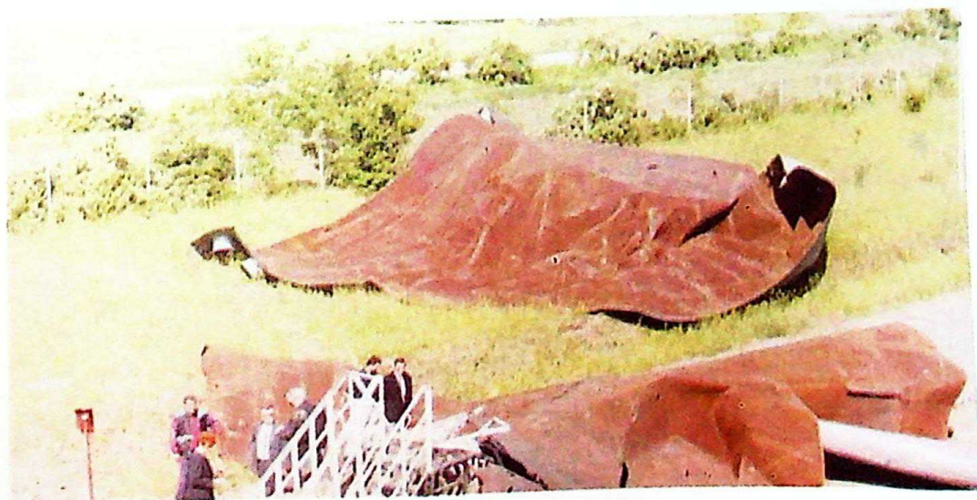
Photo 23 Projected pieces of the oil storage tank No. 3 from the storage area of "Naftagas promet" in Sombor
