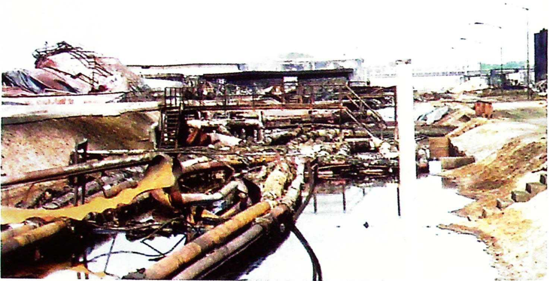
Photo 36 Close-up of the destroyed pipeline installation of Novi Sad oil refinery
