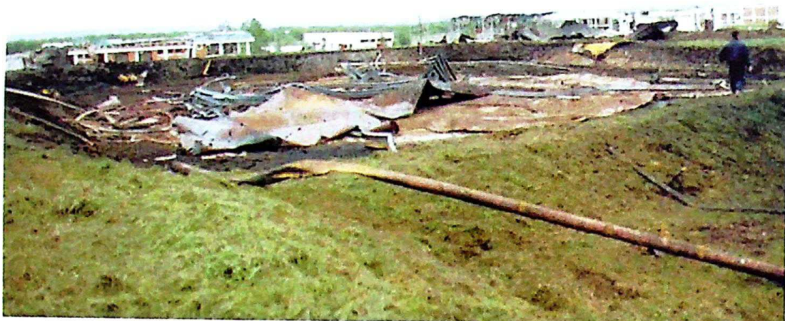
Photo 5 Demolished oil storage tank R-7 of NIS "Jugopetrol" in Niš, May 5, 1999
