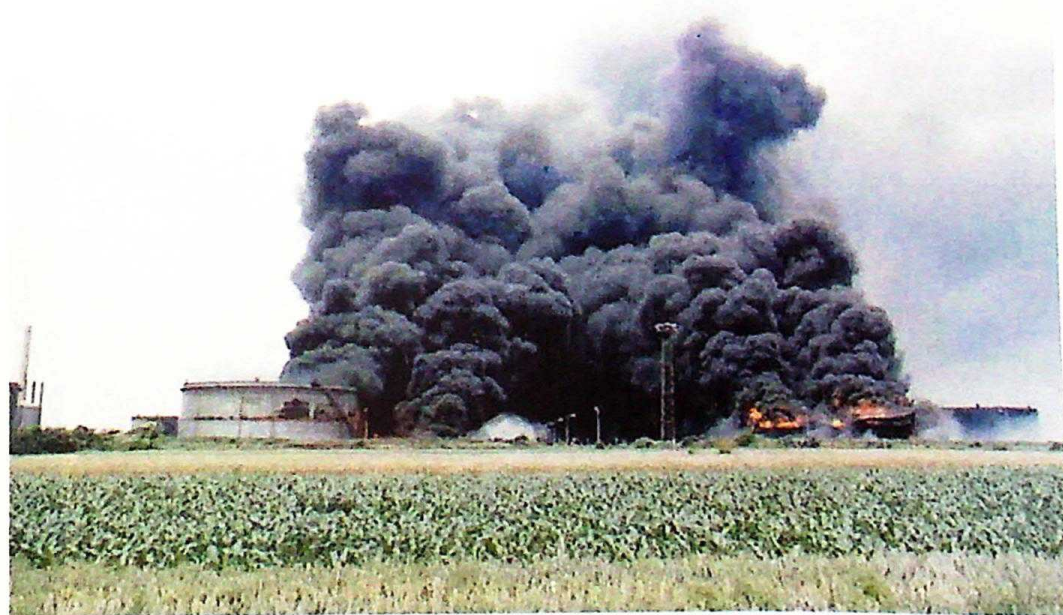
Photo 31 Pančevo oil refinery-oil storage tanks bombed on June 8, 1999
