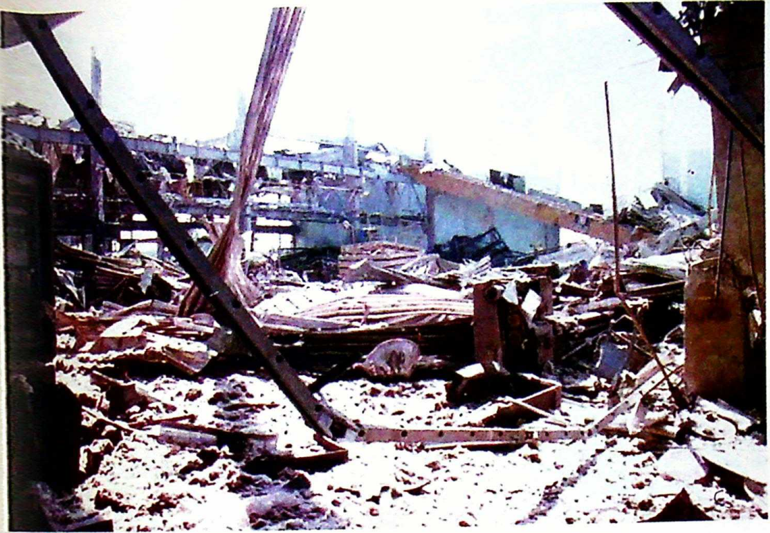
Photo 13 View of the destroyed mechanical treatment workshop of "Cer" factory
