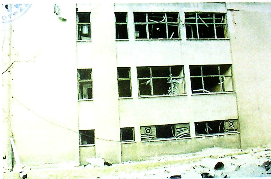
Photo 18 Broad view of the damage on No. 3 transformer station building within the compound of RTB Bor, May 15, 1999
