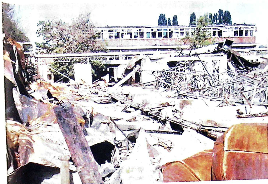
Photo 11 Destroyed "Stara mašinska" unit of DD "Krušik", Valjevo, May 4, 1999
