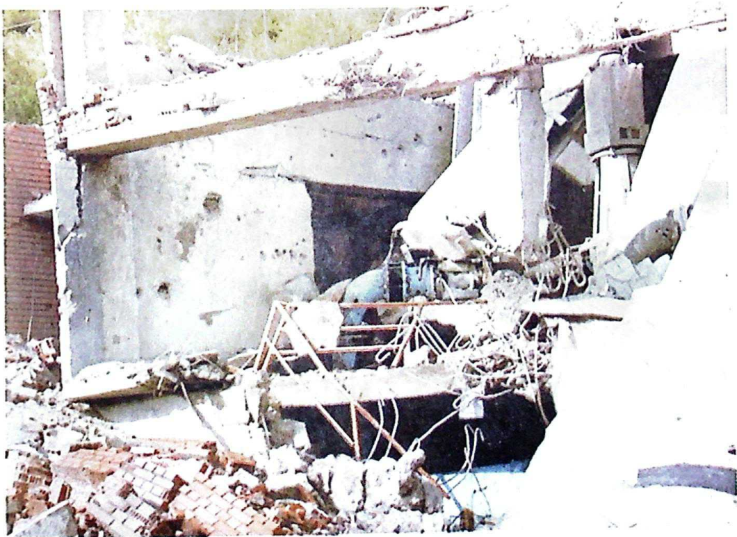
Photo 1 Destroyed water-pumping station "Badovac" in the village of Badovac – Priština, May 2, 1999
