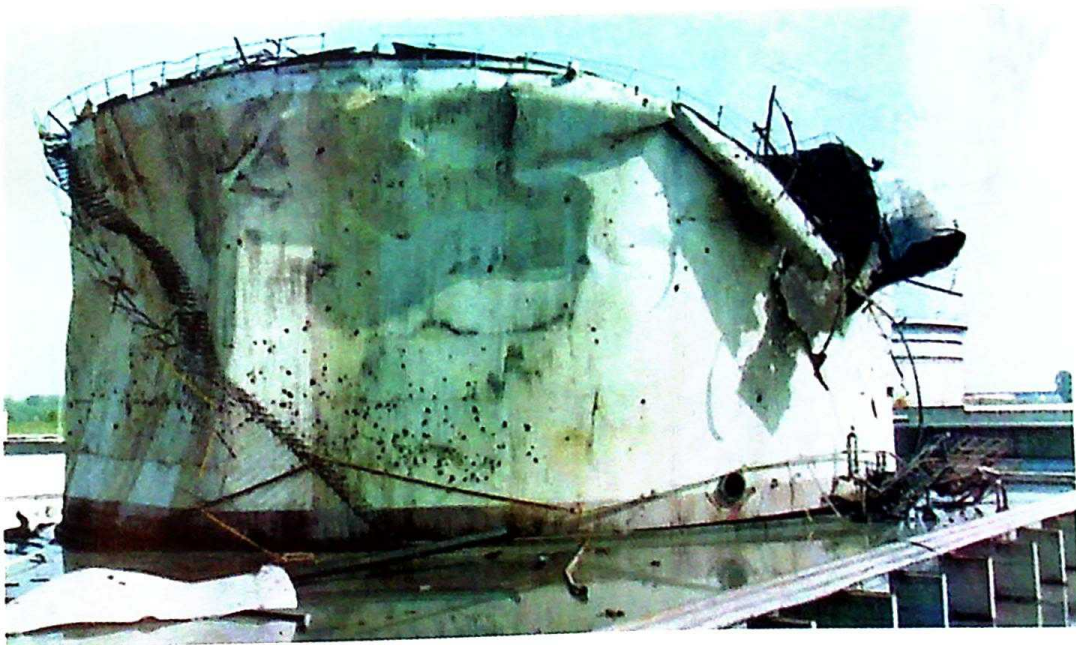
Photo 2 Destroyed oil storage tank R-24
