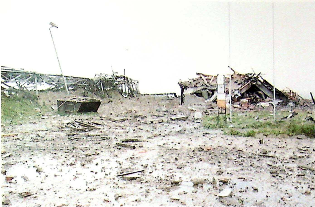
Photo 7 Demolished fuel oil pump station and transformer station of "Jugopetrol" – Beograd, Prahovo-Bor installation, May 7, 1999 (1st attack)
