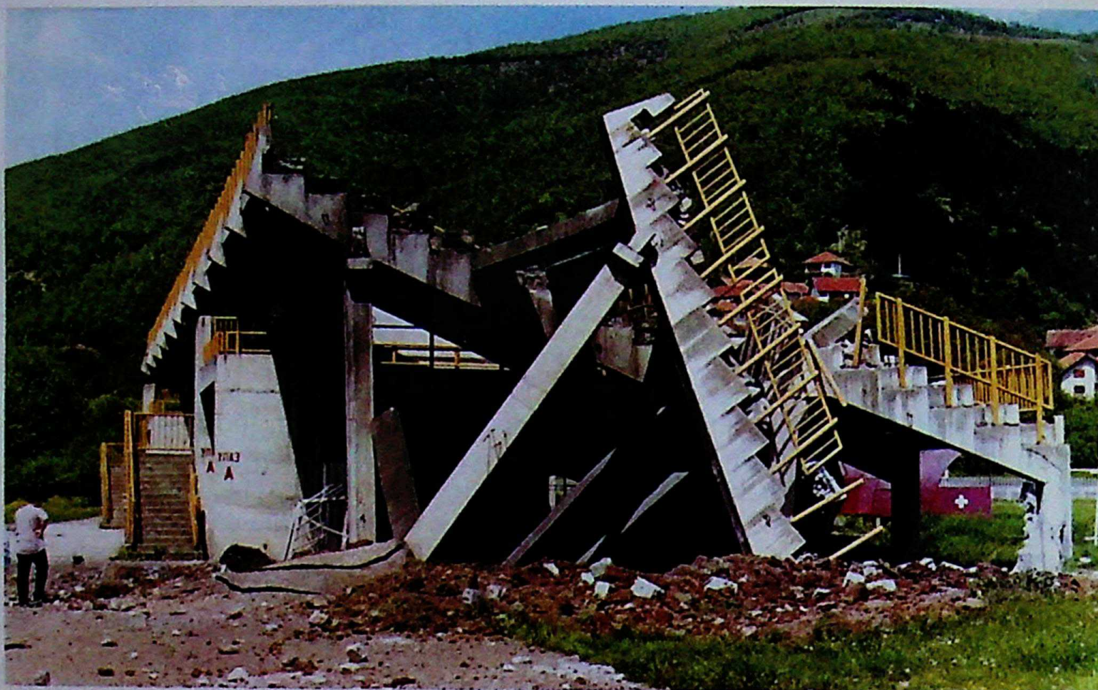
Photo 5 Sports stadium in Prijepolje after the bombing of May 11, 1999, at approximately 12:40 p.m.
