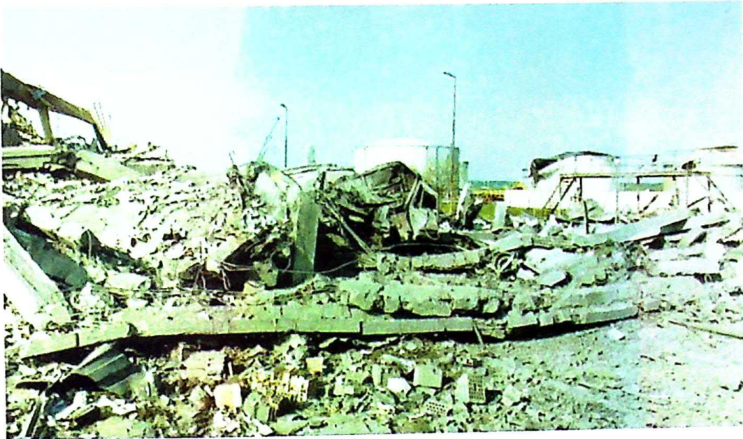
Photo 1 Destroyed administration building and maintenance shop of NIS Jugopetrol – "Instalacija" Smederevo, April 29, 1999
