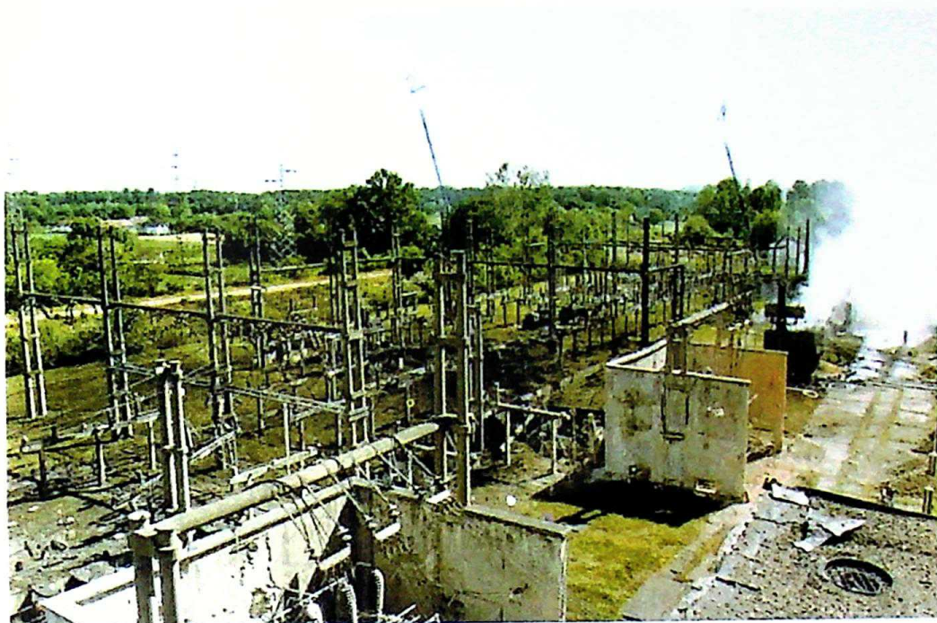
Photo 41 Demolished high-voltage installation of "Veliki Crljeni" power plant, Lazarevac, May 22, 1999
