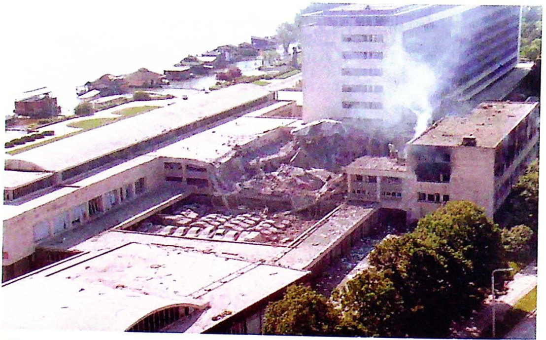
Photo 1 Demolished building of "Jugoslavija" Hotel, No. 3 Bulevar Nikole Tesle, May 8, 1999
