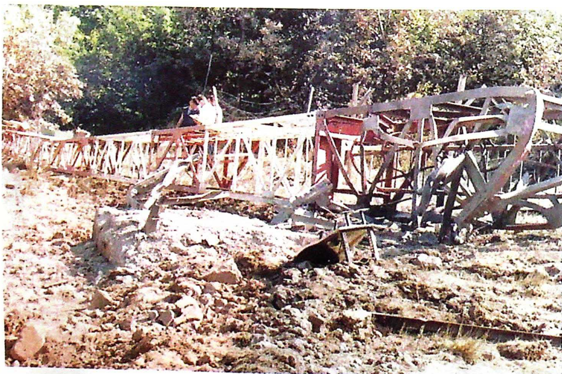
Photo 36 Toppled antenna pole of the repeater of TV Kraljevo, Electric Power Company and Public Utility Company "Putevi" on "Borča" hill in the village of Sikča, Kraljevo municipality, June 3, 1999
