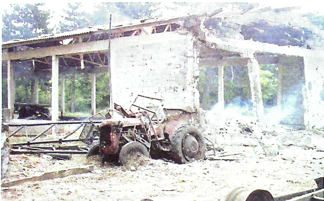
Photo 65 Demolished hay storage "E" on the farm in the village of Podgorac, where workers Nebojša Srbulović, Milija Andrejević and Slavka Trikanović were killed
