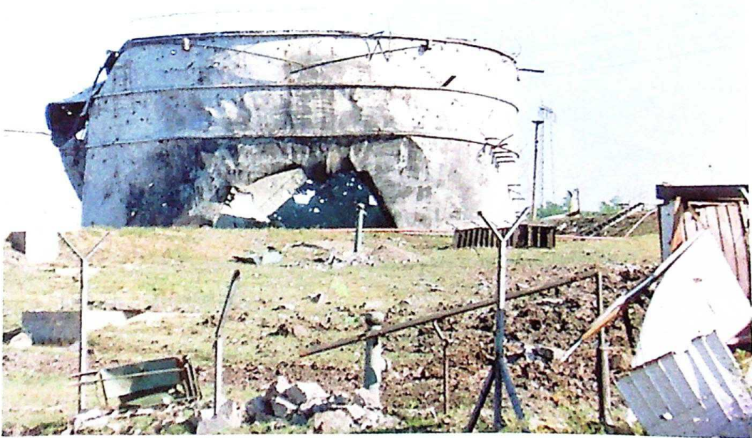
Photo 27 View of oil storage tank No. 5 in the storage area of "Jugopetrol" Bor, hit on May 27, 1999
