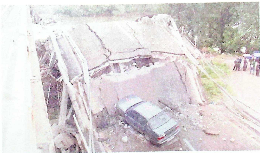
Photo 44 Close-up of the destroyed bridge and the car of the make Daewoo A6 03KDF, owned by the Romanian Red Cross, which happened to be on the bridge and in which three Romanian humanitarian workers sustained minor injuries
