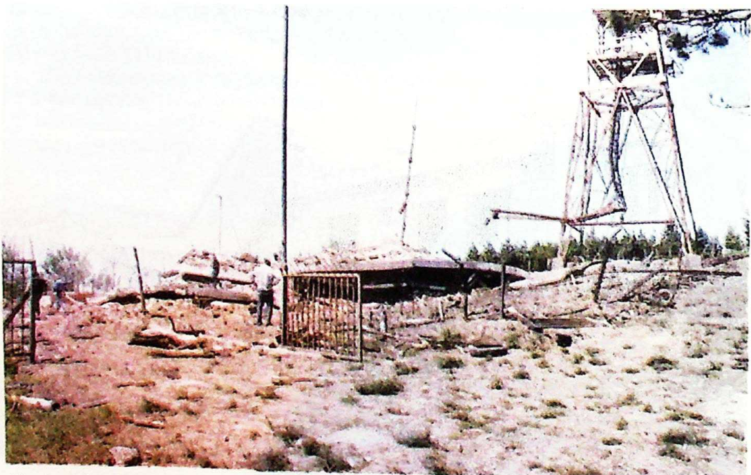
Photo 16 Close-up of the demolished building and damaged antenna pole on Mt. Cer, May 19, 1999
