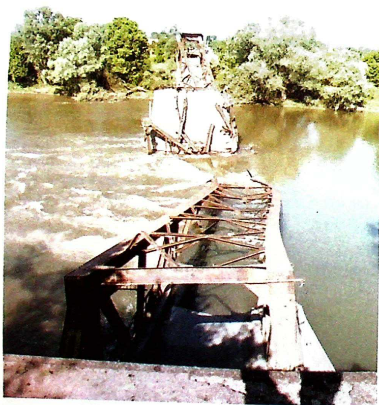
Photo 96 Close-up of the destroyed bridge in Varvarin 9 people lost their lives and 32 were injured
