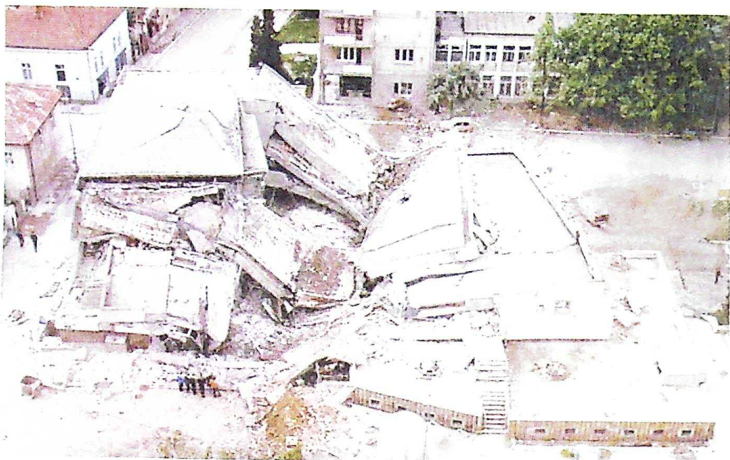
Photo 45 The destroyed building of the Užice Business Unit of the Public Enterprise of PTT Traffic and "Telekom Srbija", May 9, 1999 (after the second attack)
