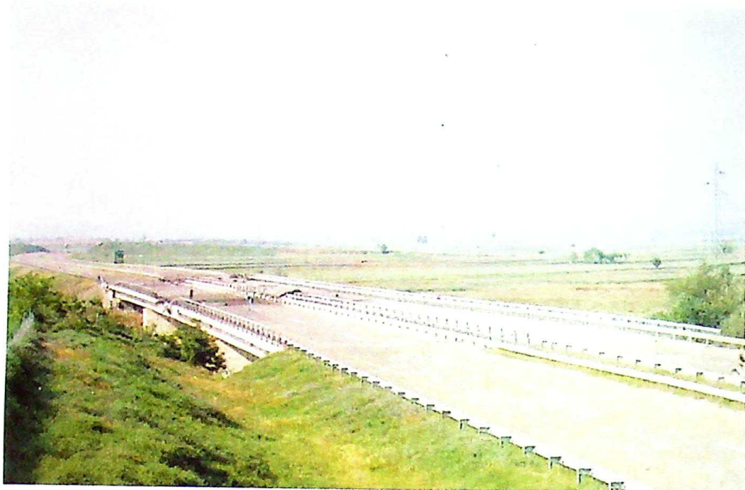
Photo 89 Damaged bridge over the river Nišava on the Belgrade–Niš–Leskovac motorway in the area of the village of Popovac, May 28, 1999
