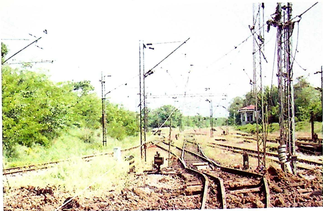
Photo 87 Damaged railway tracks and power line at the marshaling yard in the village of Popovac–Niš, May 27, 1999
