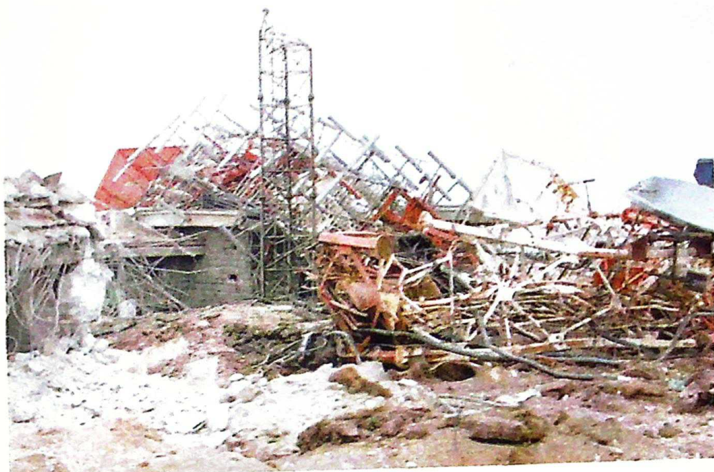
Photo 13 Completely destroyed RTS TV transmitter on the location called "Gobelja", Mt. Kopaonik, Kraljevo, May 19, 1999 (3rd attack)
