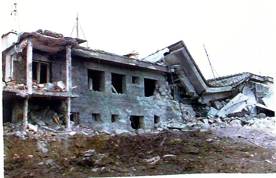
Photo 14 Demolished building of the RTS TV transmitter on "Gobelja", Mt. Kopaonik, Kraljevo, May 19, 1999
