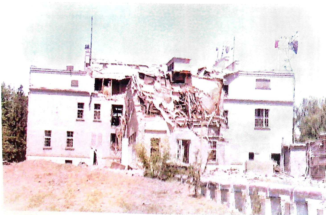
Photo 27 Demolished building of the Serbian Radio and Television – medium-wave and short-wave transmitters in the village of Zvečka-Obrenovac, May 30, 1999, Repeaters and Relays
