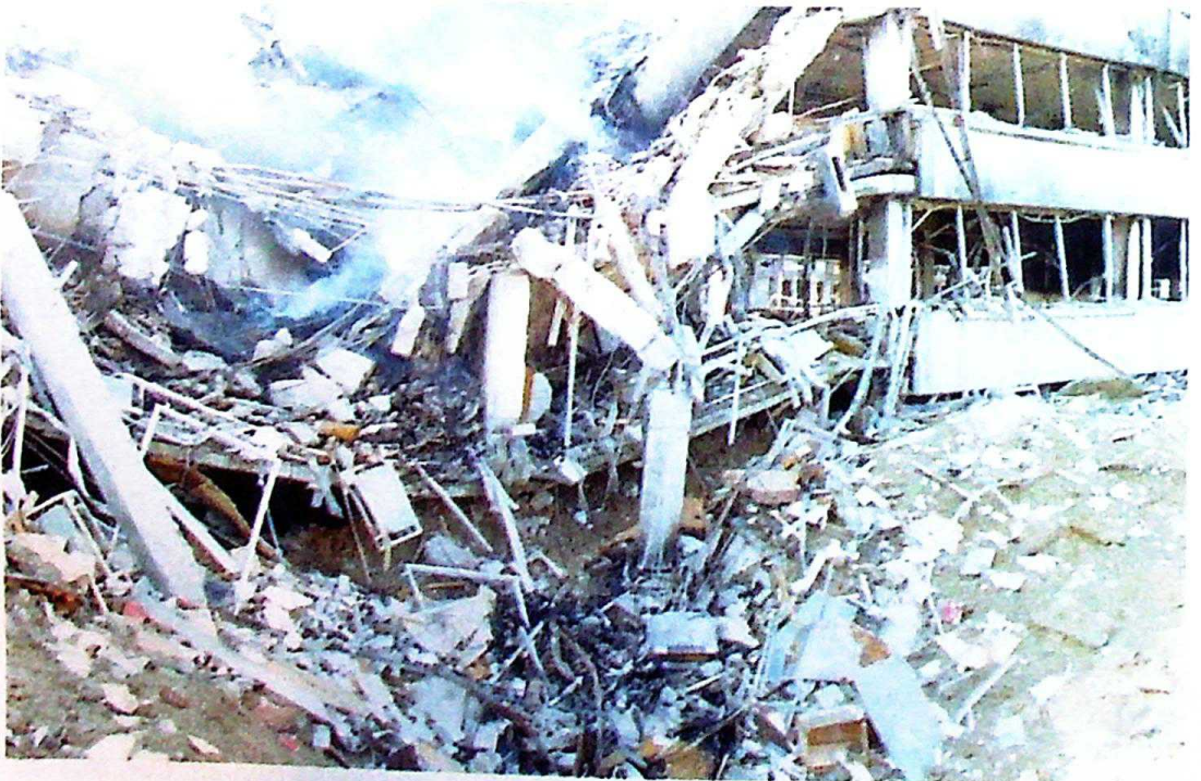
Photo 20 Close-up view of the destroyed RTS building of TV Novi Sad (3rd attack)
