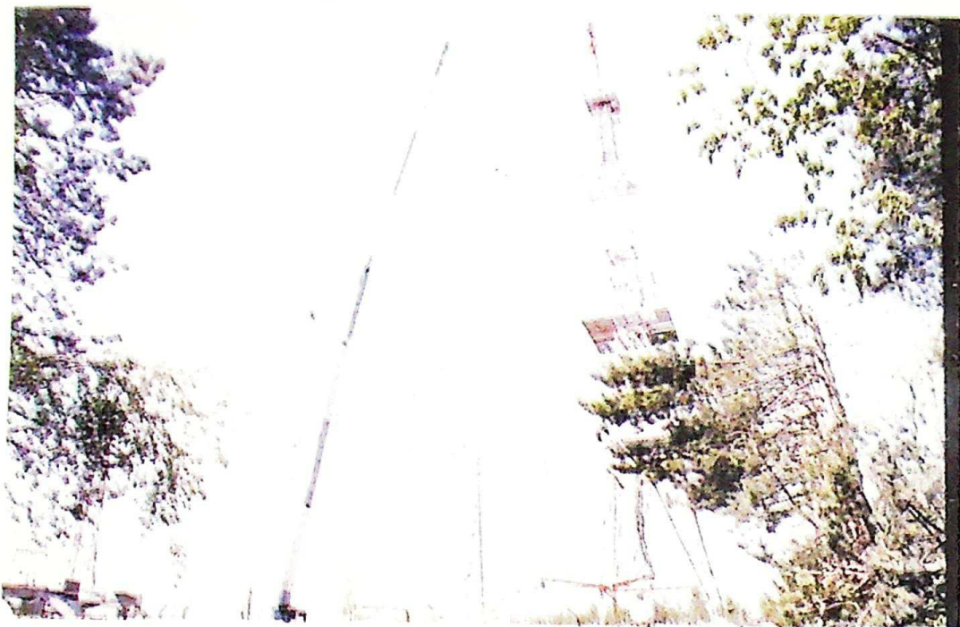
Photo 15 Bombed repeater of Telekom Srbija on Mt. Cer, Šabac, May 19, 1999 (5th attack)
