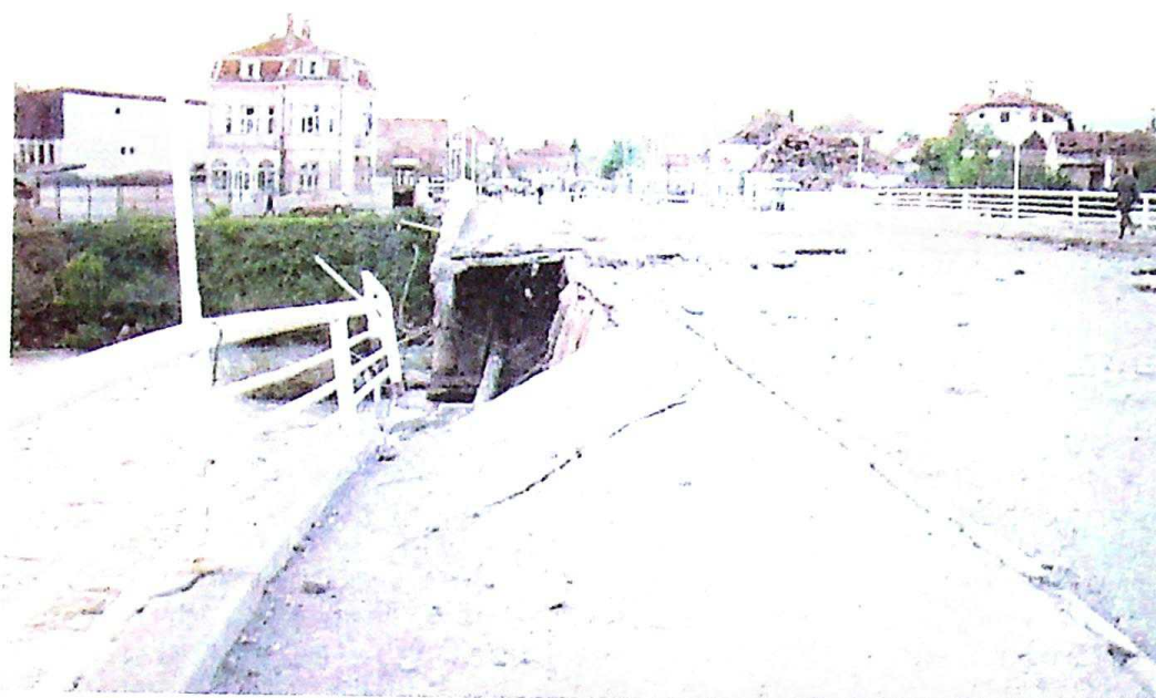
Photo 41 View of the demolished bridge on the river Nišava and the damaged building of the Greek Consulate in Niš, May 8, 1999
