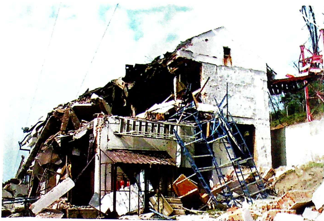
Photo 10 Destroyed building of the RTS repeater on Vršački breg in Vršac, May 11, 1999
