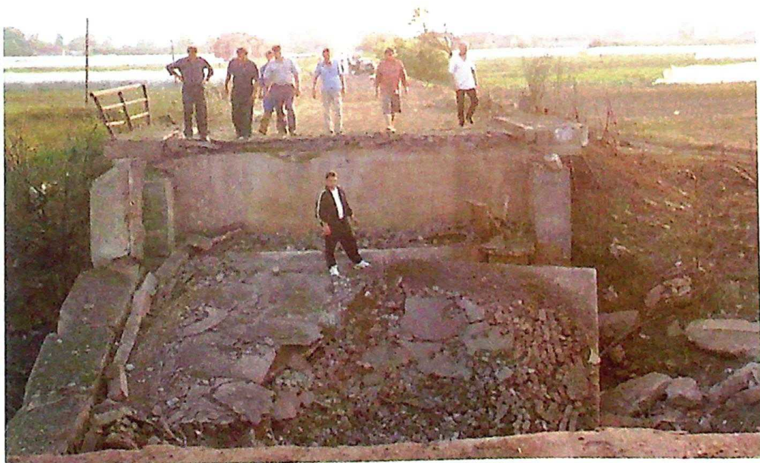
Photo 84 Close-up of the destroyed Čenovački bridge in the vicinity of which Stanoje Stojimenović (1941) from Čenovac was killed while working in the field with his wife and son, 29 May 1999
