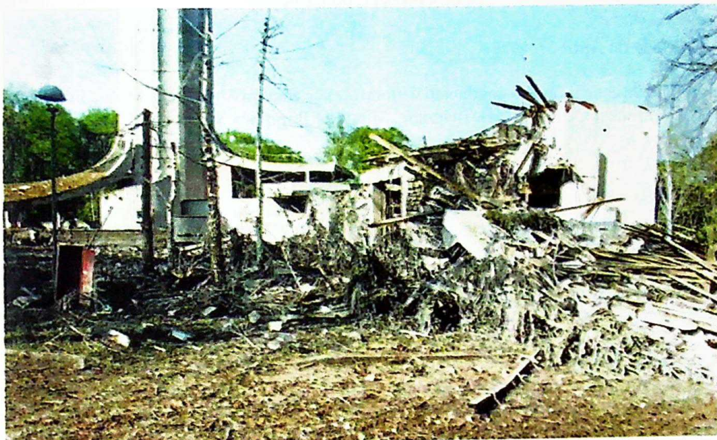
Photo 1 Demolished building at the foot of the Serbian Radio Television (RTS) transmitter tower on Iriški Venac, April 27, 1999 (1st attack)
