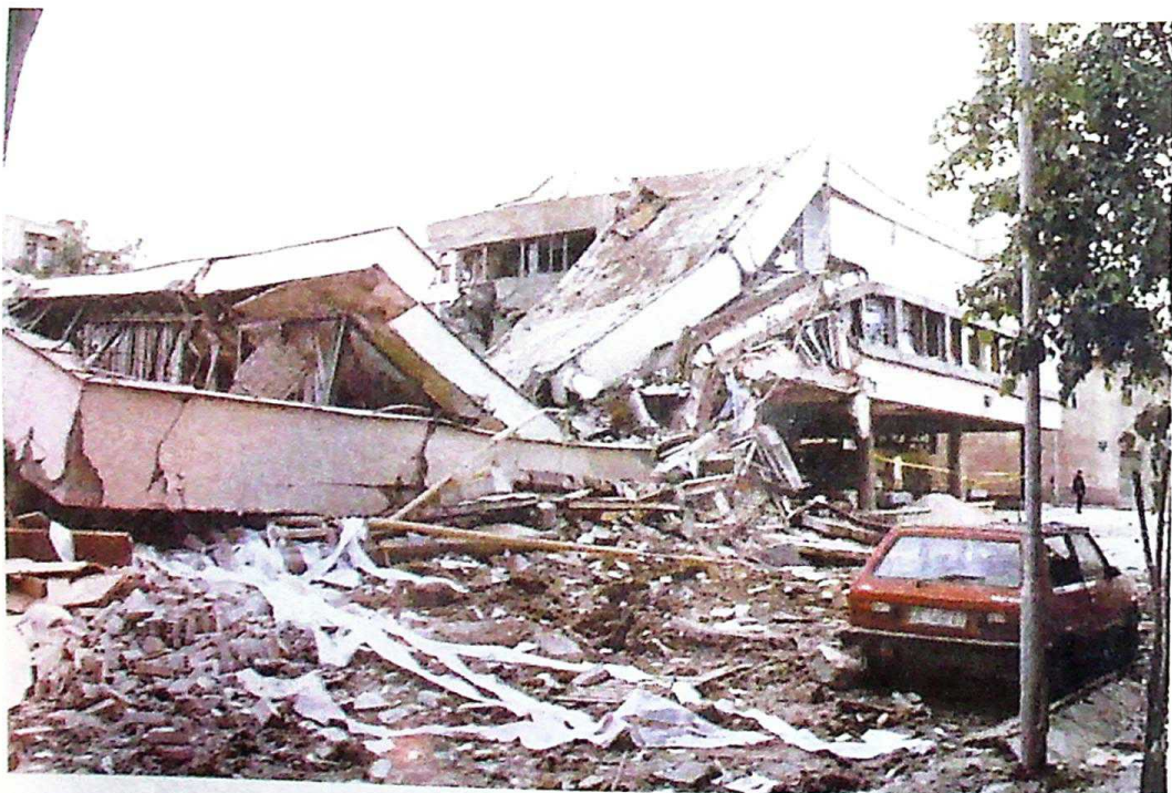
Photo 46 Close-up of the destroyed post office building in Užice, May 9, 1999
