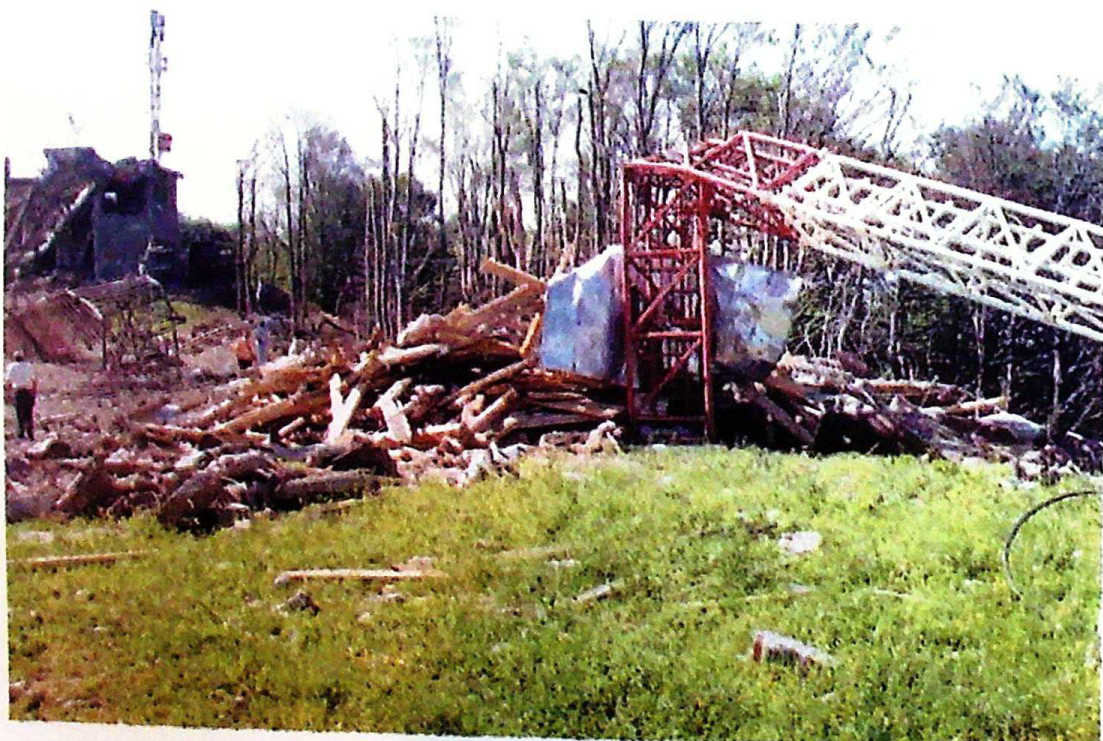
Photo 34 Destroyed RTV "Politika" and "Mobtel" repeater on Cvijićev Vrh peak on Mt. Rudnik – 3 June 1999
