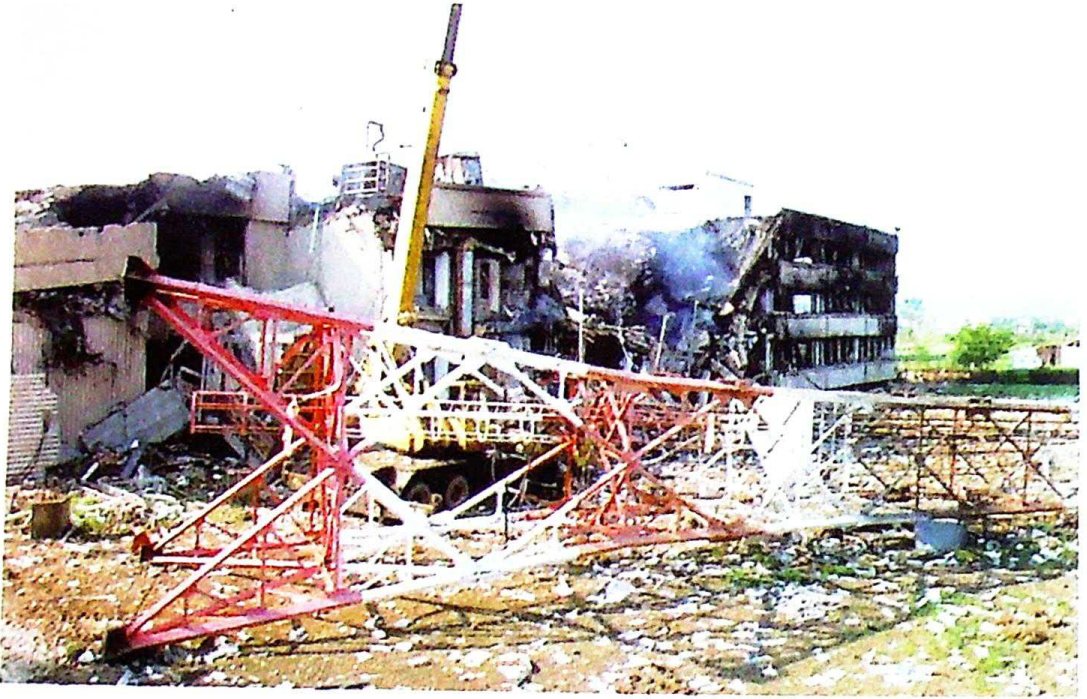
Photo 19 Repeated bombing of the RTS building in Petrovaradin, Novi Sad, 45 Kamenički put St., May 26, 1999 (3rd attack)
