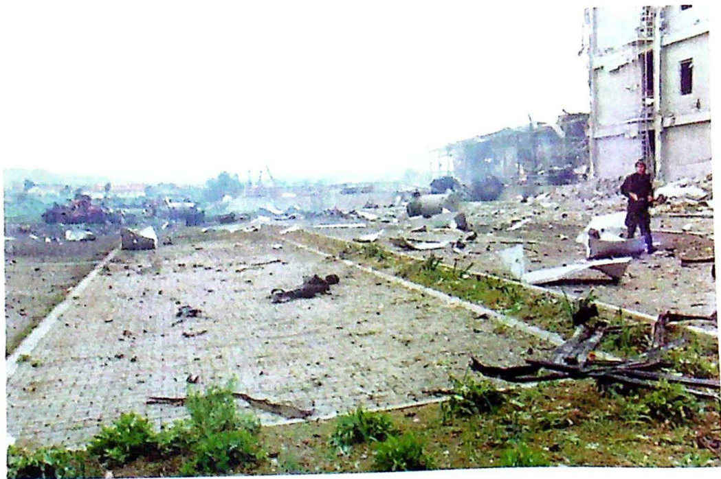
Photo 12 Broad view of the destroyed set props warehouse and mechanical workshop of RTS TV Novi Sad, May 13, 1999 (2nd attack)
