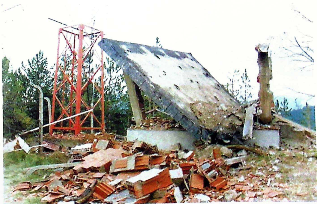
Photo 29 Demolished RTS repeater facility and aerial post in Kozji Do – Vranje
