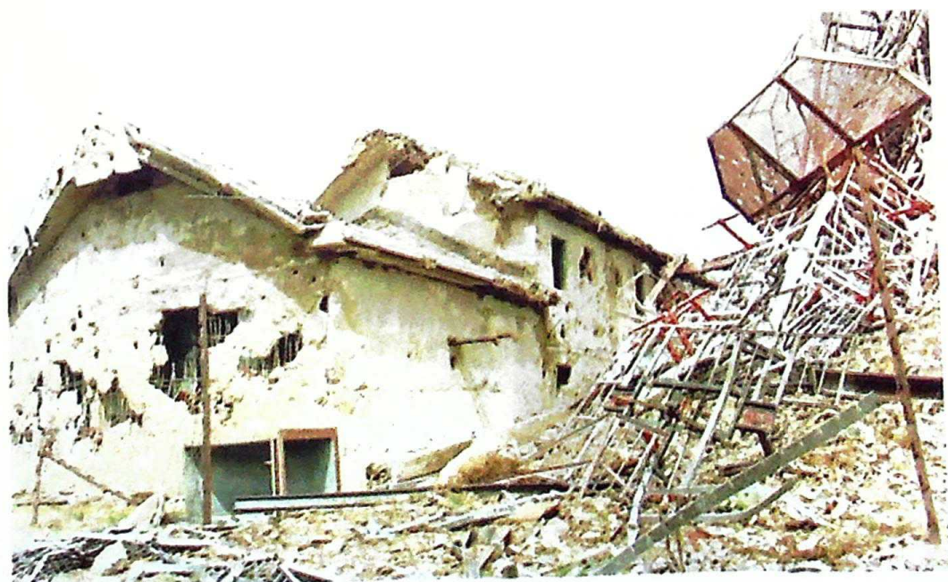
Photo 33 Destroyed RTS repeater facility and aerial post on Mt. Besna Kobilja, 3 June 1999
