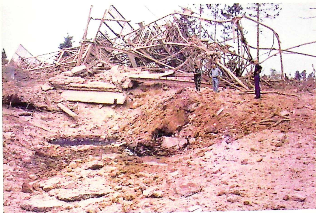
Photo 17 Destroyed Telekom Srbija repeater on Mt. Cer, Šabac, May 20, 1999 (6th attack)
