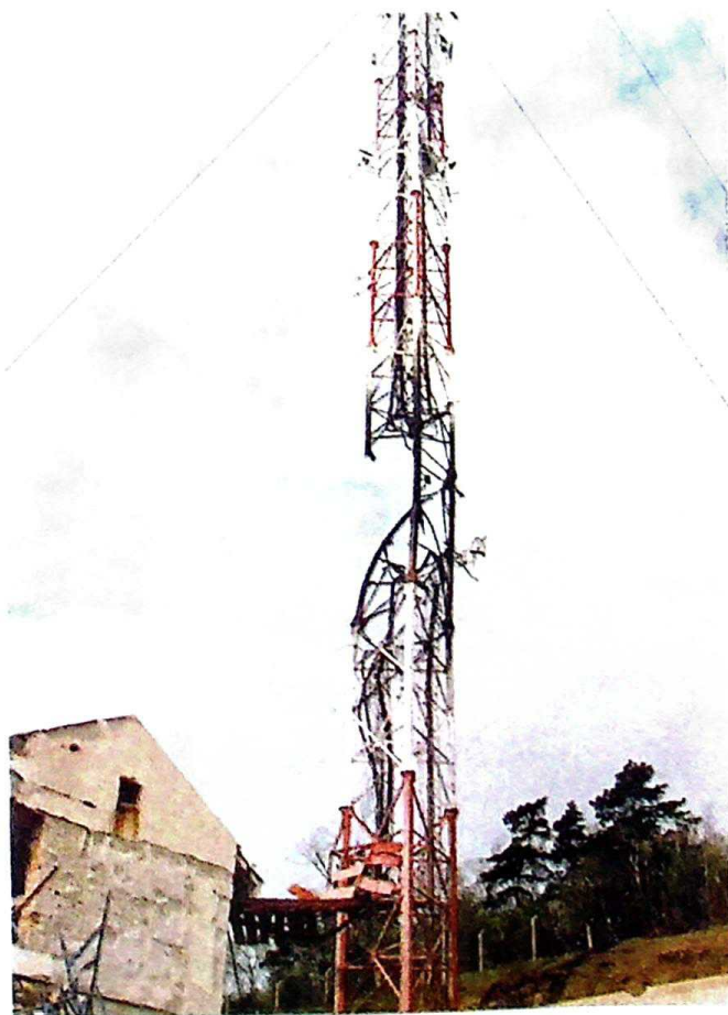
Photo 9 Demolished antenna pole of the repeater in Vršac
