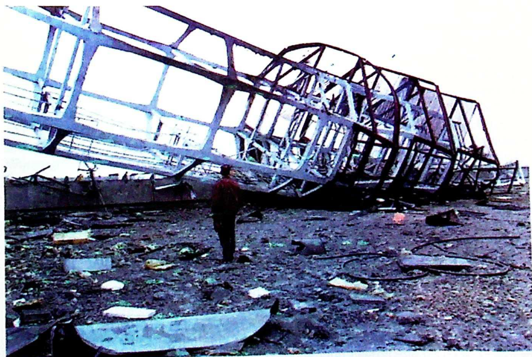
Photo 6 View of the toppled radio and TV tower of TV "Novi Sad" (1st attack)
