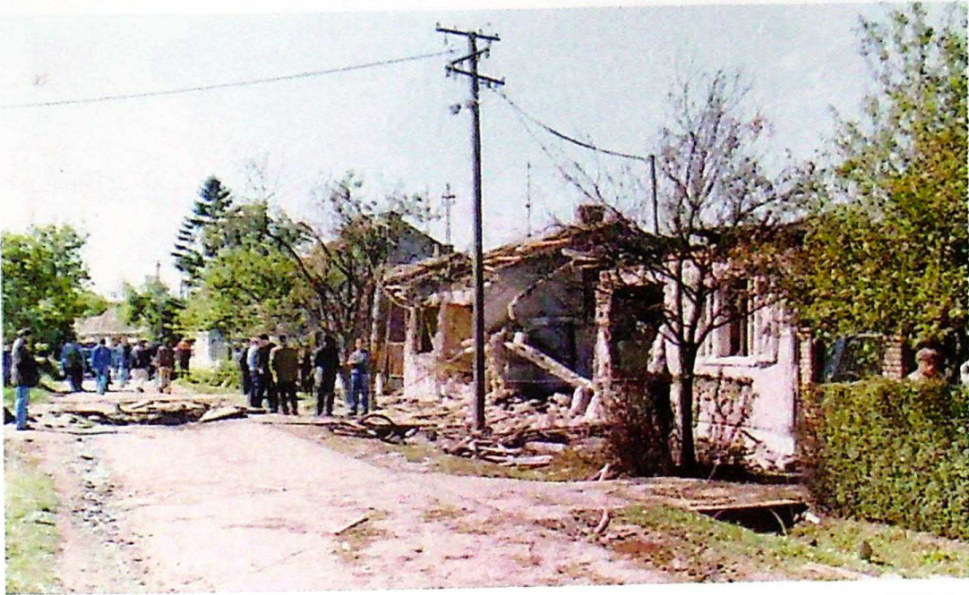
Photo 95 Destroyed houses on Vuka Karadžića Street, Sombor; one person was killed and several were injured. About 50 houses were destroyed or damaged on 21 May 1999
