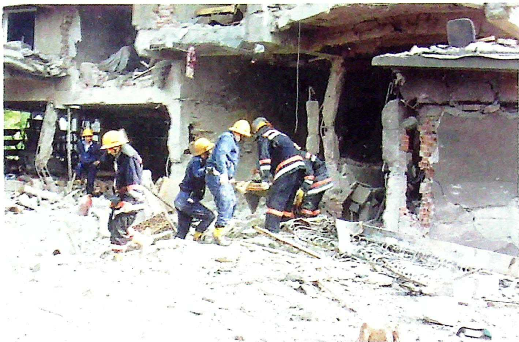
Photo 139 Pulling out of the victims from the rubble
