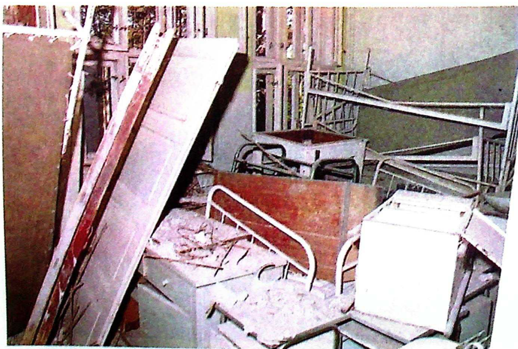
Photo 16 One of the demolished patients' rooms
