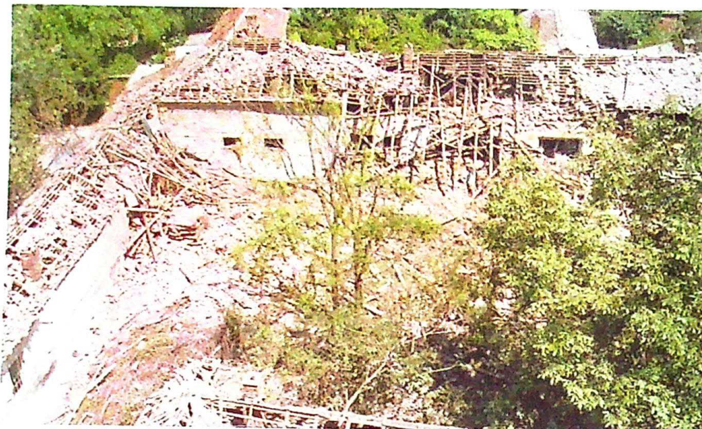
Photo 125 Destroyed houses on Dositejeva St., Nos. 3-15, in Ćuprija. In the bombing of the center of Ćuprija about 100 civilian buildings were destroyed or damaged (houses, flats, shops, etc.) and about 20 people were severely injured, 29 May 1999
