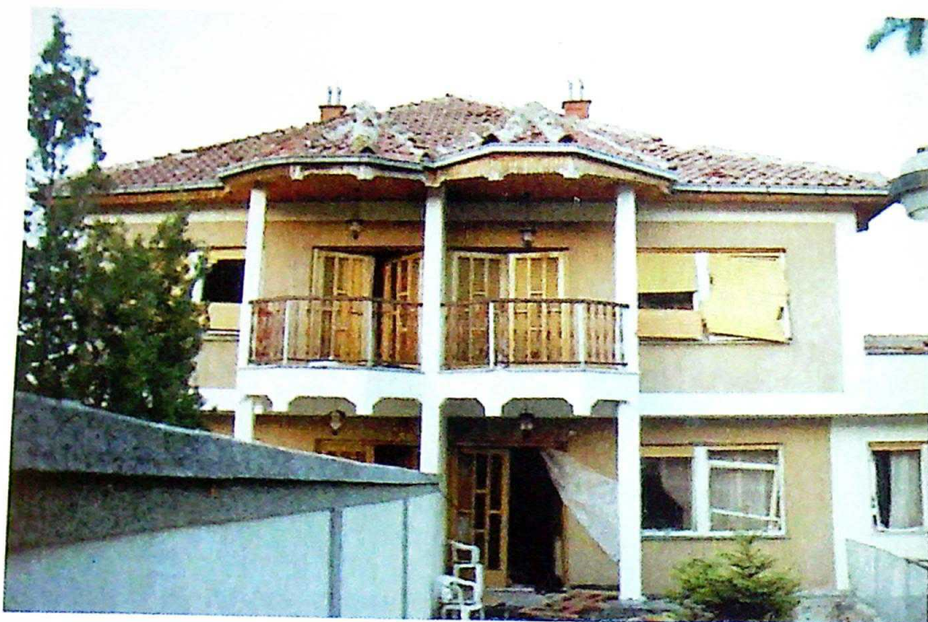
Photo 101 Damaged house in Djakovica in which its owner, Ibrahim Djoši, was killed, 21 May 1999
