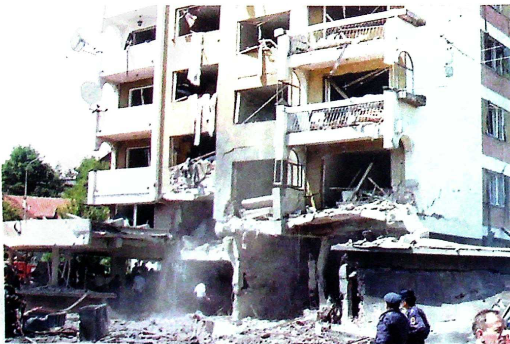
Photo 138 Close-up of the destroyed building at No. 74 Stevana Nemanje St.
