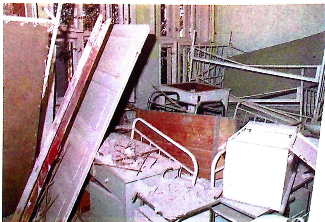
Photo 16 One of the demolished patients' rooms
