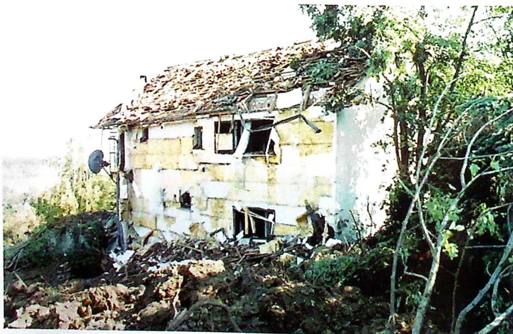
Photo 122 One of the destroyed houses in Petrovaradin, suburb of Ribnjak – Novi Sad, on 29 May 1999
