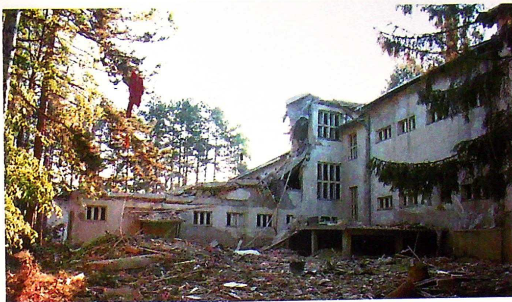
Photo 13 Special Lung Hospital "Sanatorium" in Surdulica, bombed on the night of 30/31 May 1999. In addition to hospital patients, the facilities of this hospital were used as a shelter for refugees from Croatia and as the Home for the Aged and Homeless
