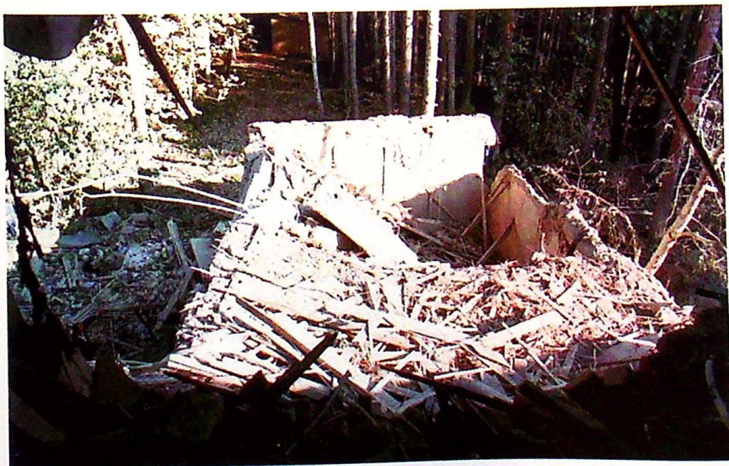
Photo 14 View of one of the demolished buildings. In "Sanatorium" facilities 19 persons were killed and 38 injured
