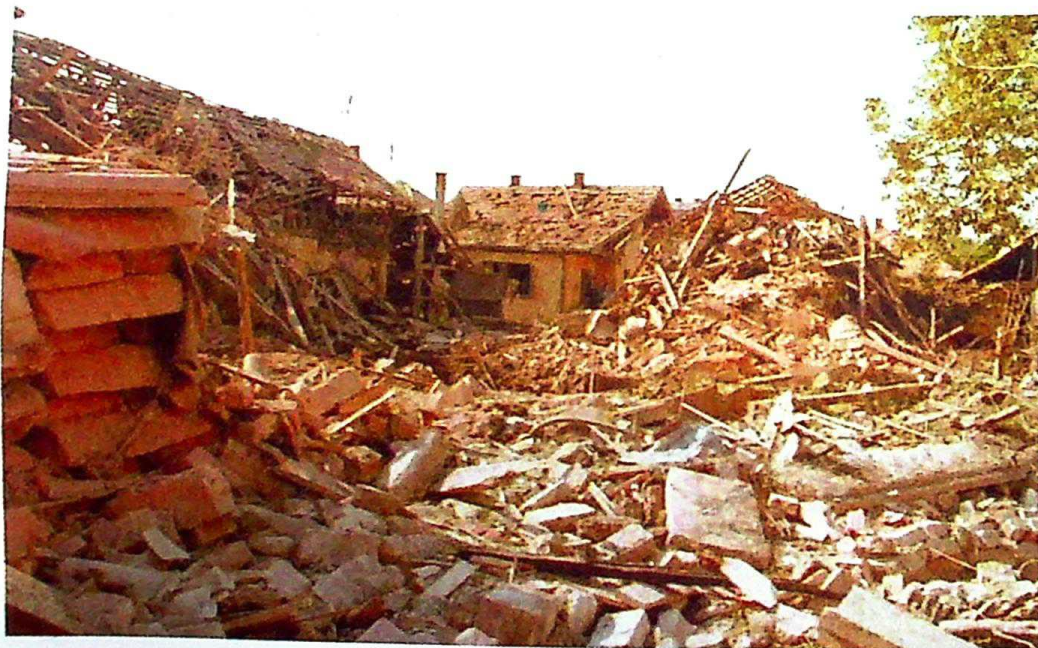
Photo 126 The site where a missile landed in the backyard of Slobodan Petrović and destroyed the house and all auxiliary buildings, No. 7 Dositejeva St., Ćuprija, 29 May 1999
