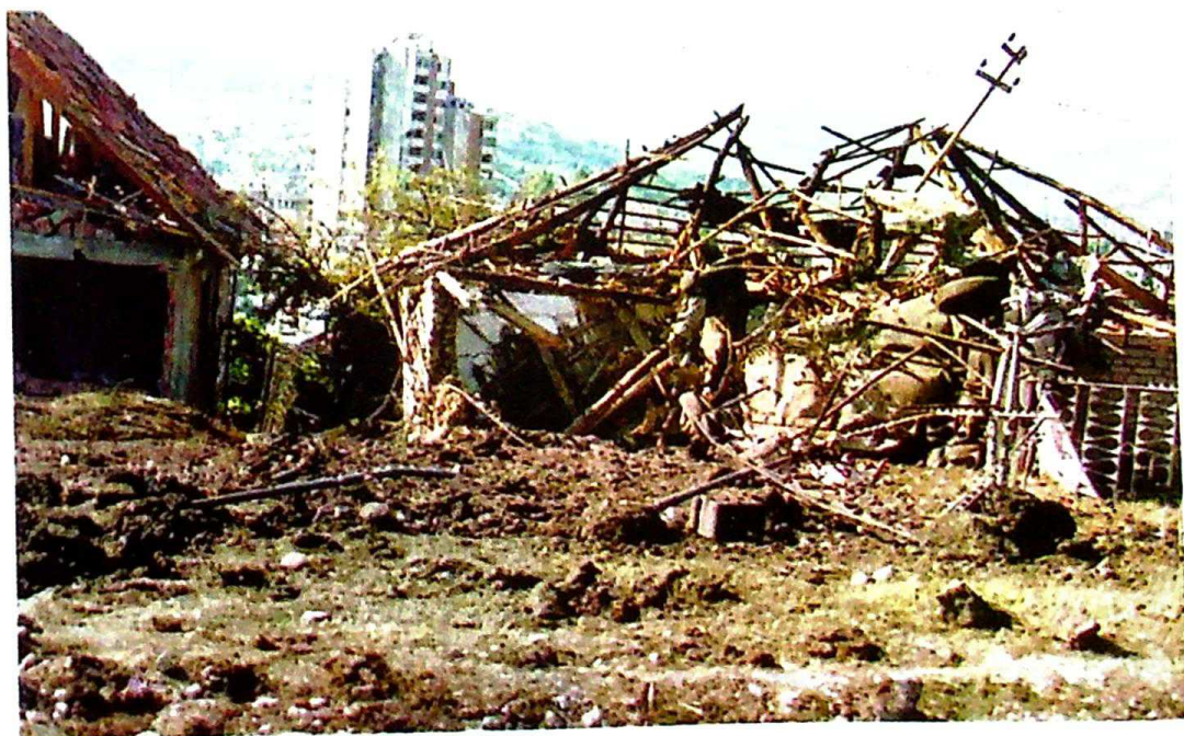
Photo 152 Close-up of the demolished house of Rade Filipović on Miodraga Jovanovića Street – Novi Pazar, 1 May 1999
