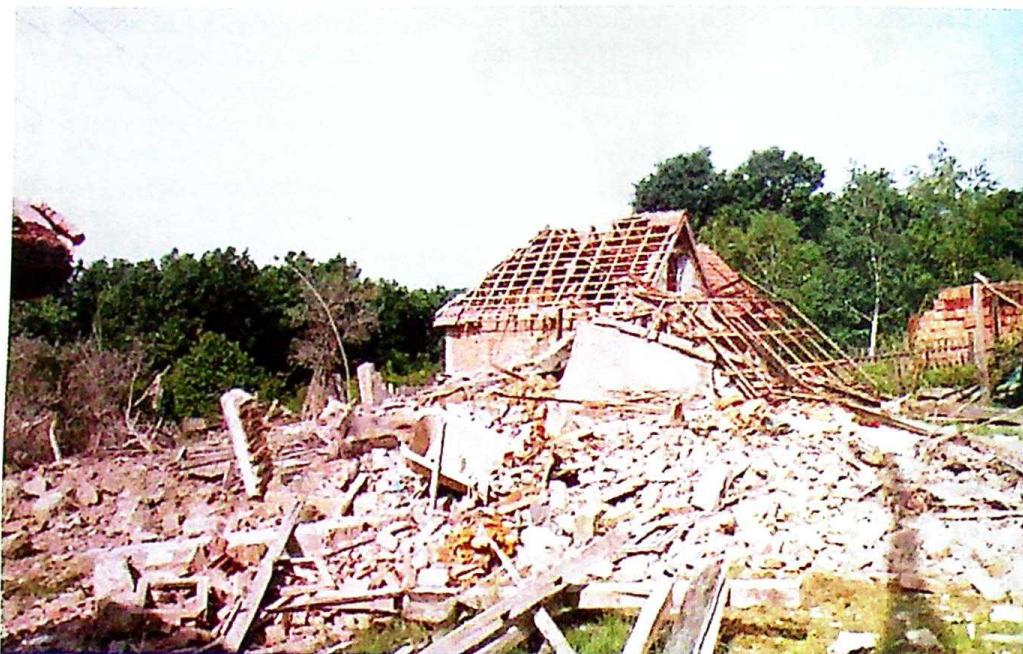
Photo 92 The destroyed household, house and auxiliary buildings in the village of Jasenica – Valjevo, belonging to Mileta Krunić, whose wife Milka Krunić was killed on 18 May 1999
