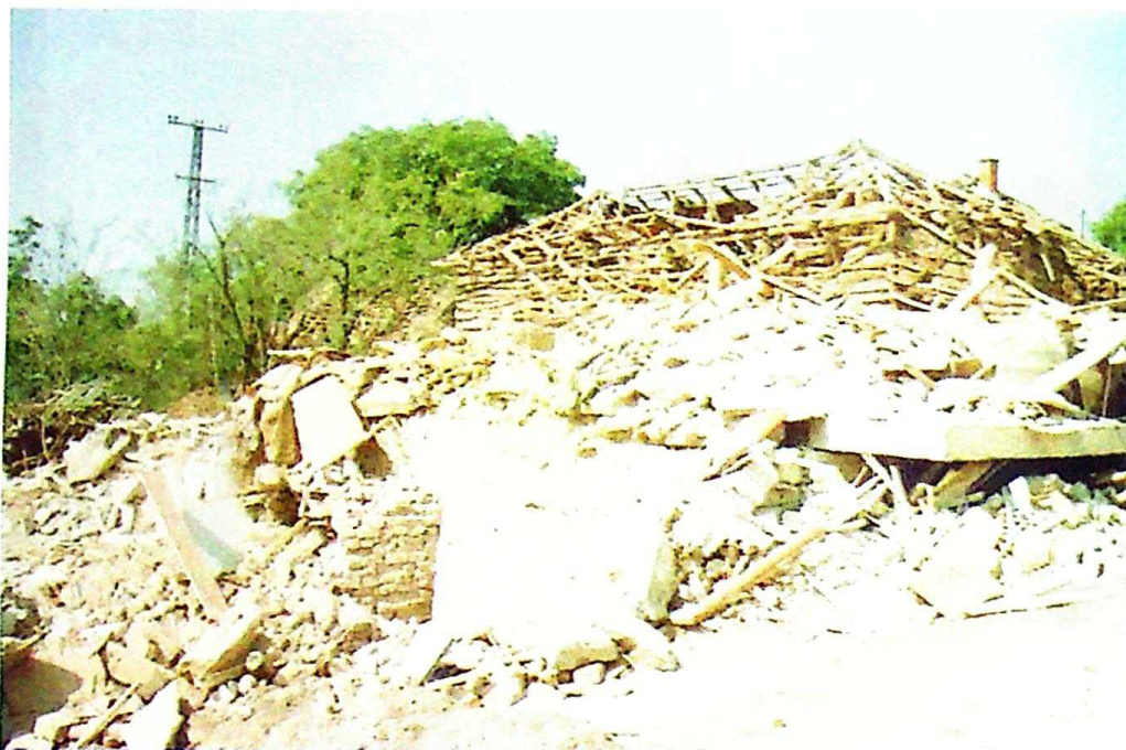
Photo 117 Totally destroyed house at No. 23 Niška St., in Aleksinac, in which its owner, Branko Mitrović, was killed on 28 May 1999
