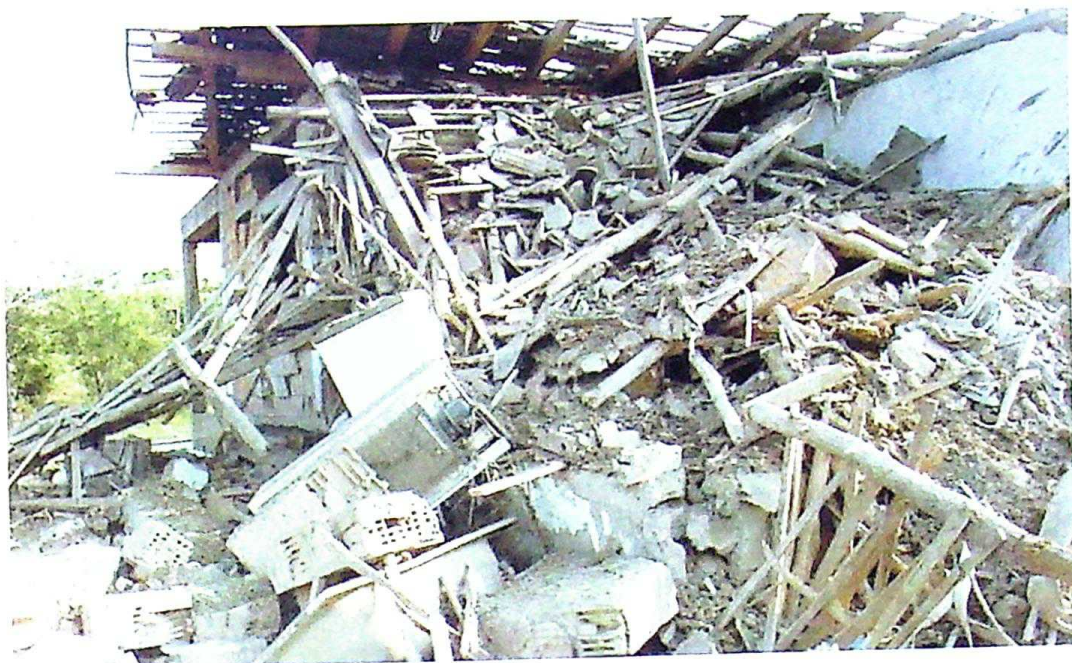
Photo 133 Destroyed house in Ripanj – Belgrade, No. 54a Put za Ivanoviće St., belonging to Miroslav Saitović, in which his wife Javorina (1957) and his son Boban (1982) were injured on 31 May 1999
