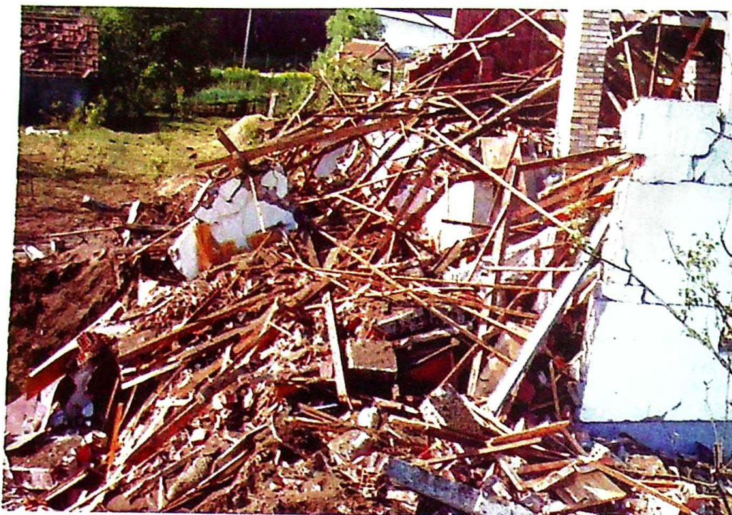
Photo 104 Demolished house and auxiliary buildings of Veroslav Barać, n.n. Mihaila Pupina St. in Novopazarska Banja. His wife, Olga Barać, and daughters, Milica and Dijana, were severely injured on 25 May 1999 (about 30 houses were damaged in Novopazarska Banja)
