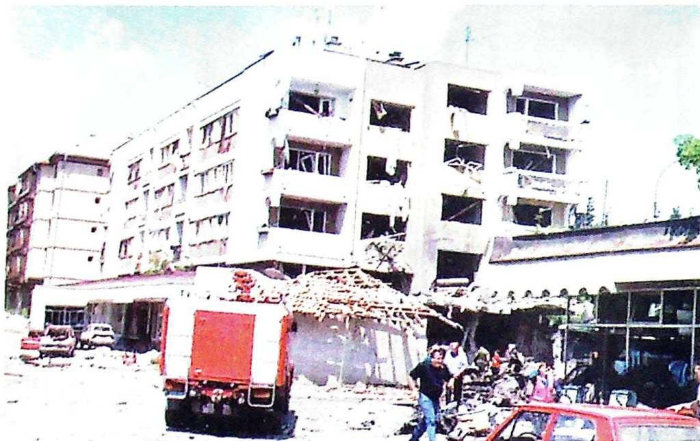
Photo 137 Bombed apartment building at No. 74 Stevana Nemanje St., near the coach station, in which 11 people were killed, about 20 severely injured, and many were left with minor injuries on 31 May 1999
