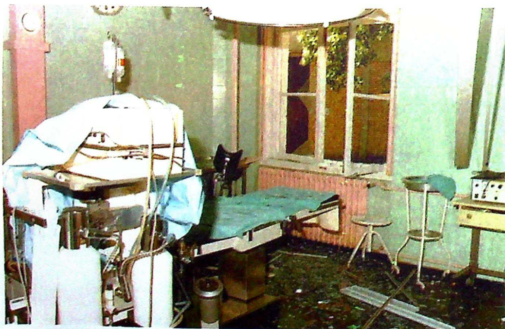
Photo 10 Damage in the operating room No. 2 of the Gynecology Clinic, "Dragiša Mišović" KBC, 20 May 1999
